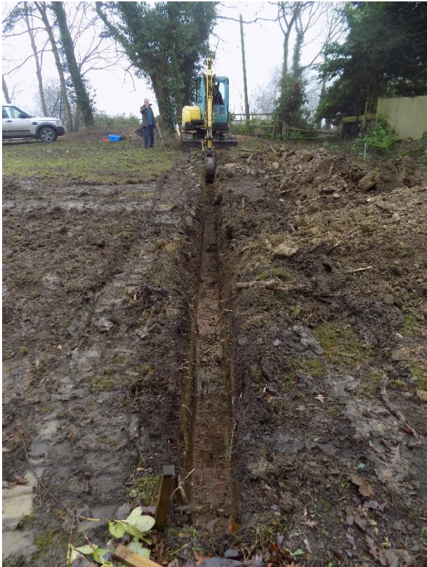
Figure 8: Post excavation of the footing trench looking east.
