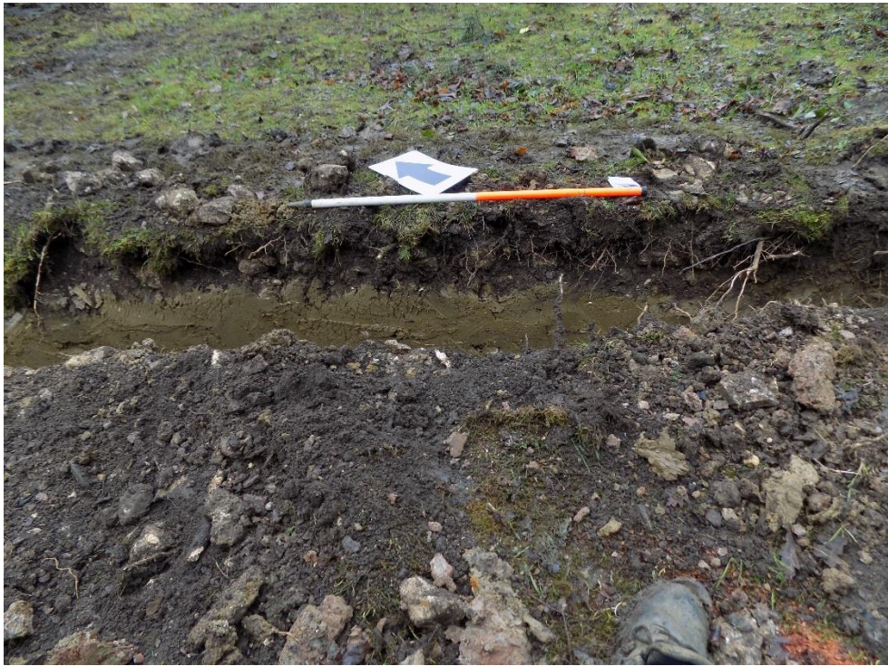
Figure 9: North-east section of the foundation trench where limestone cobbled layer was situated.
