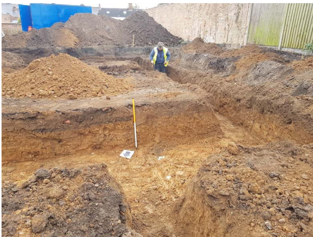
Figure 11: Visit 2. Excavation complete at the southern part of the site (plot 2).
