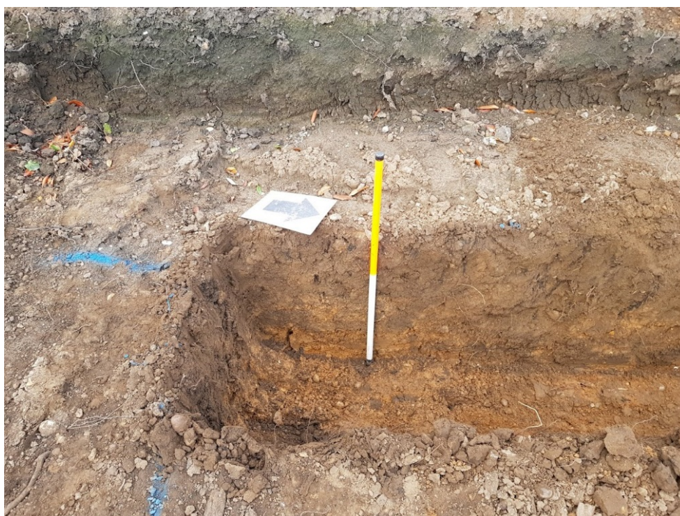
Figure 8: Visit 2. Excavation of the foundation trenches began at plot 2.
