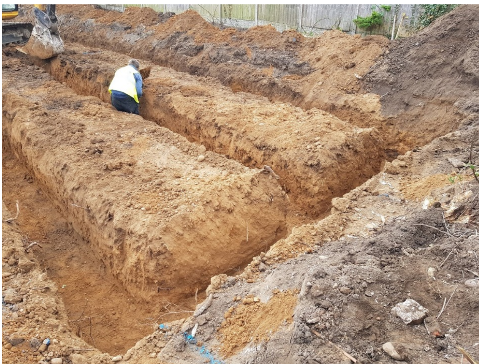
Figure 10: Visit 2. Excavation completed at the northern side of the site (Plot 3/4).
