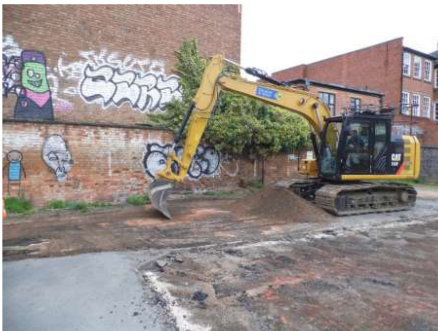
Figure 7: Machine stripping of carpark
