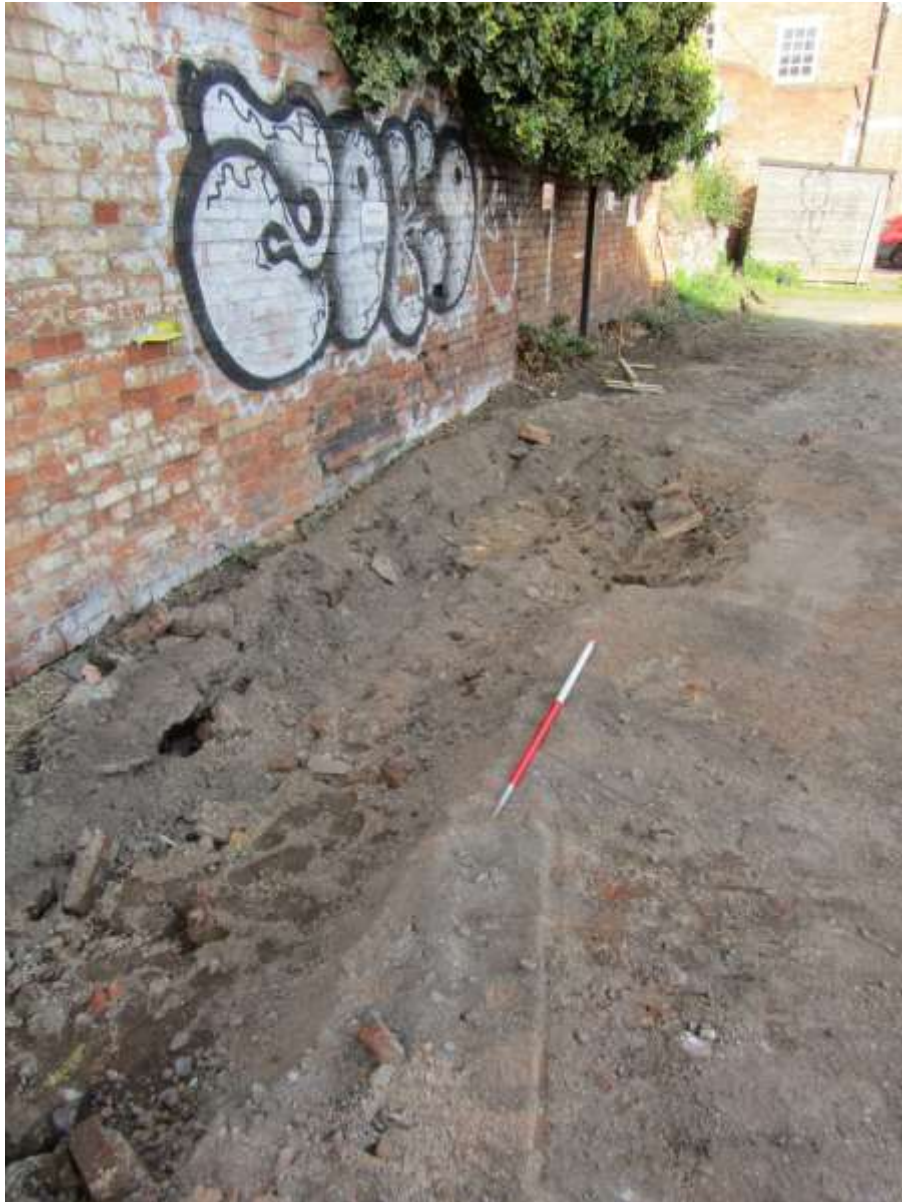
Figure 9: Perimeter kerb foundation - brick rubble
