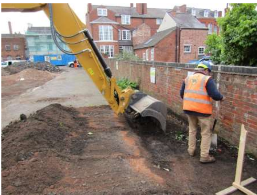
Figure 8: Perimeter kerb foundation trench
