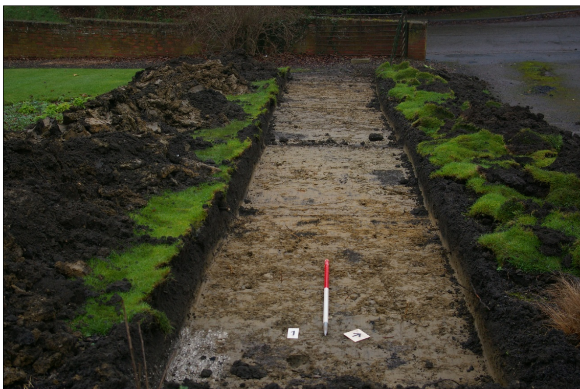
Figure 4: Trench 1 looking north west
