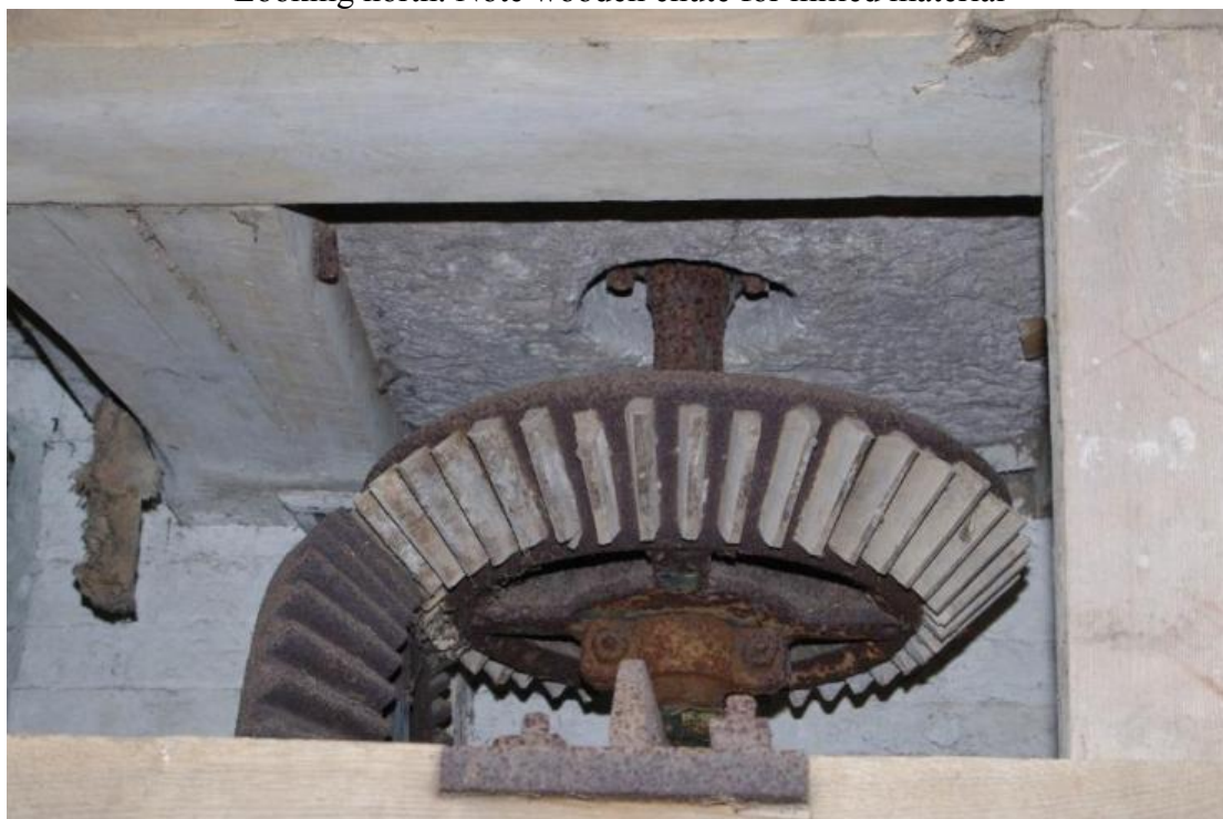
Figure 30 Building B ground floor south room millstone drive gear Looking east. Underside of millstone visible above bevel gear. Note wooden teeth on upper gear
