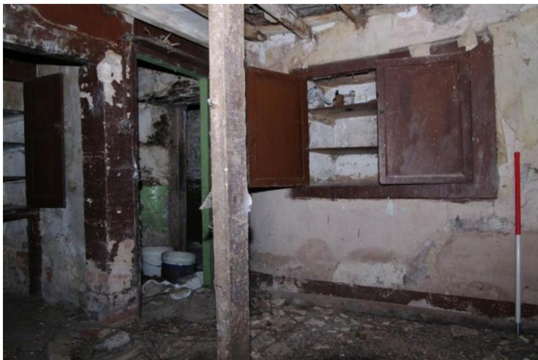
Figure 110 Room 2 former window Looking north. 1m scale
