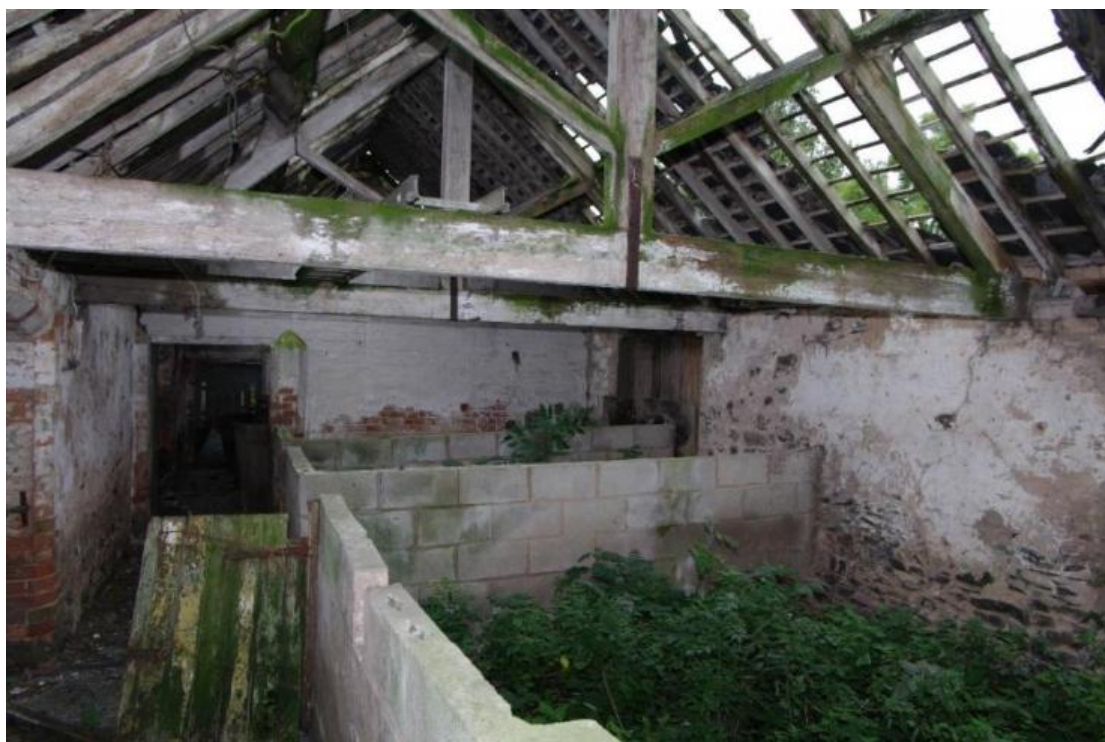
Figure 46 Building C inside detail Looking south-east from west end of building
