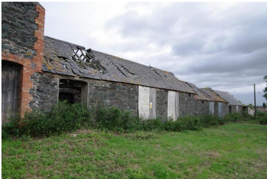
Figure 41 Building C south facing elevation Looking north-east
