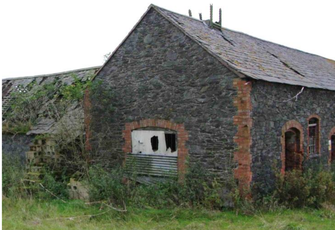
Figure 23 Building B north-facing gable end Looking south-east
