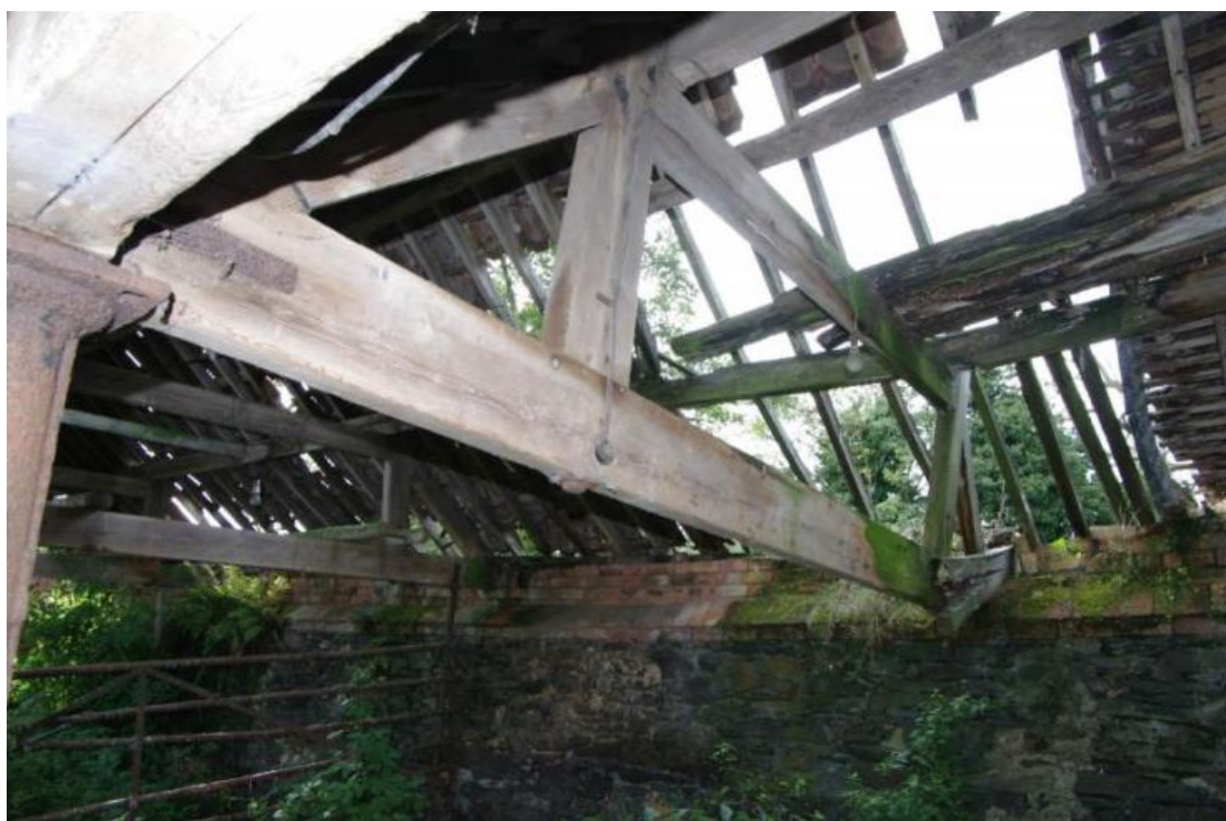
Figure 63 Building E roof structure Looking south-east
