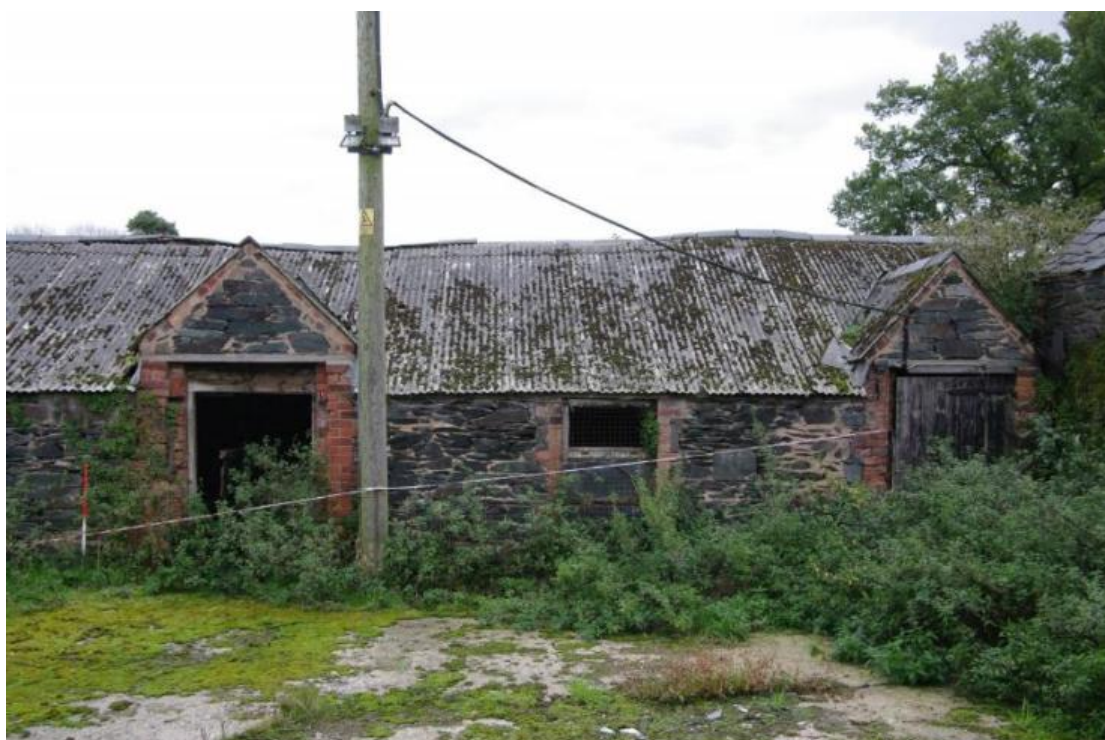
Figure 50 Building D west-facing elevation, south end Looking east. 1m scale
