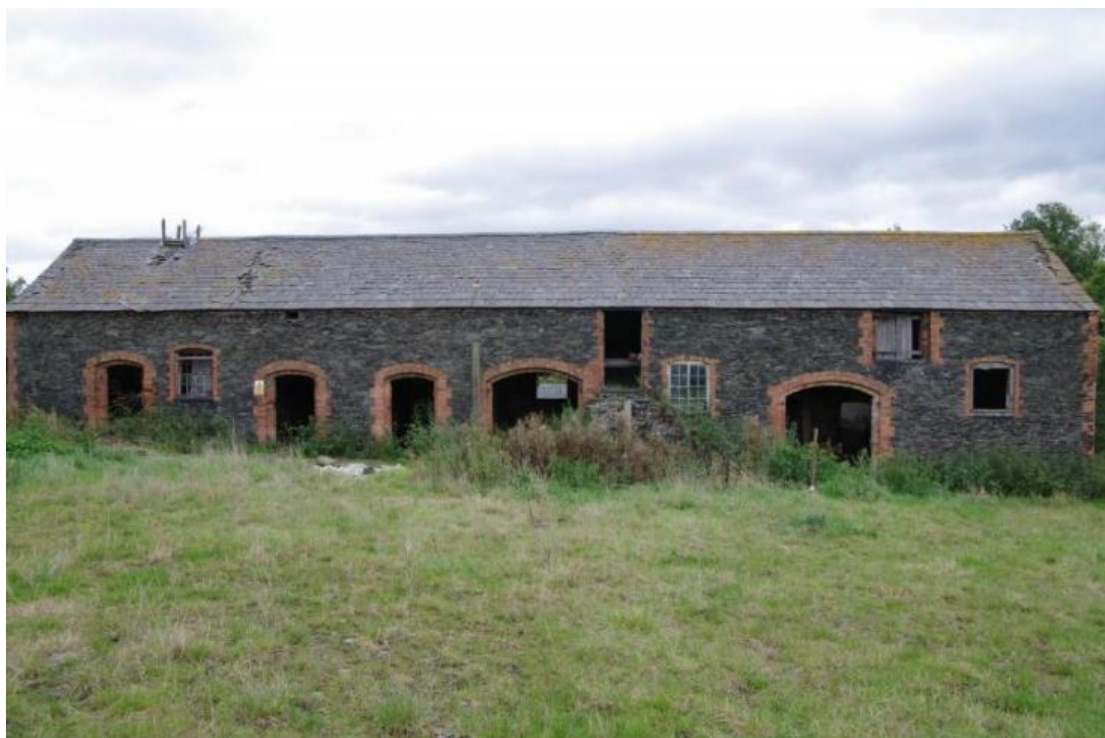
Figure 19 Building B west-facing elevation Looking east
