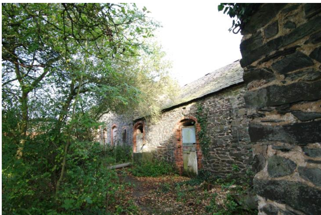
Figure 79 Building G south facing elevation Looking north-west
