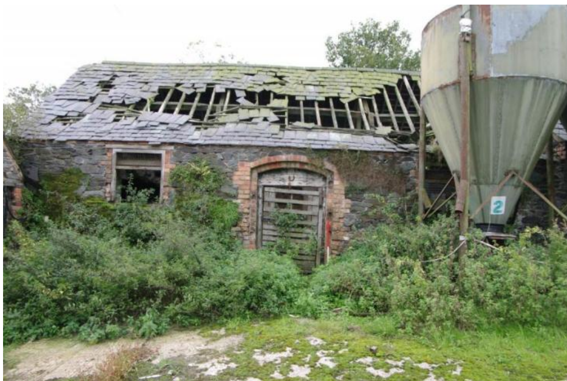
Figure 45 Building C north-facing elevation, west end Looking south. 1m scale
