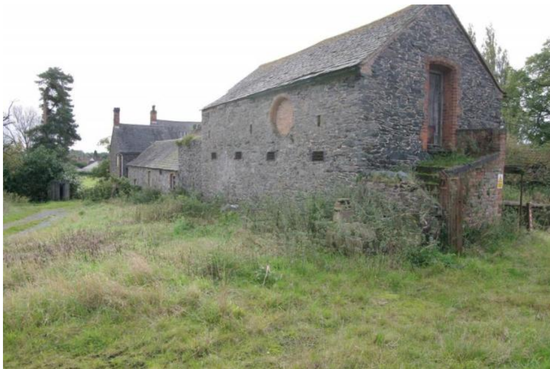
Figure 65 Building F north-facing elevation Looking south-east. Buildings G, H and house on left
