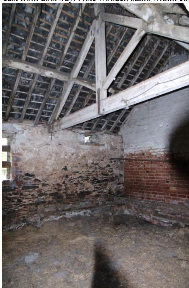
Figure 84 Building G. Former animal pen Looking north-east
