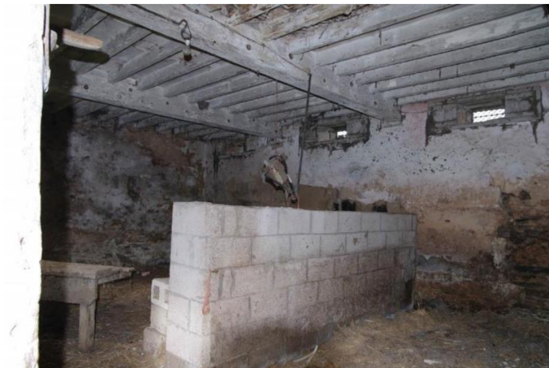
Figure 73 Building F ground floor Looking north-west. Note breeze block stall and wooden shutters on grilles in back wall
