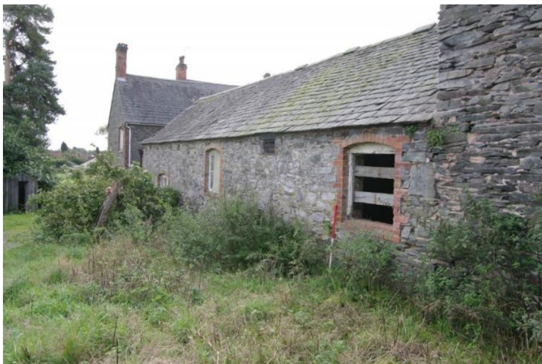
Figure 77 Building G north-facing elevation (east end) Looking south-east. 1m scale. Note joint in stonework to right of window
