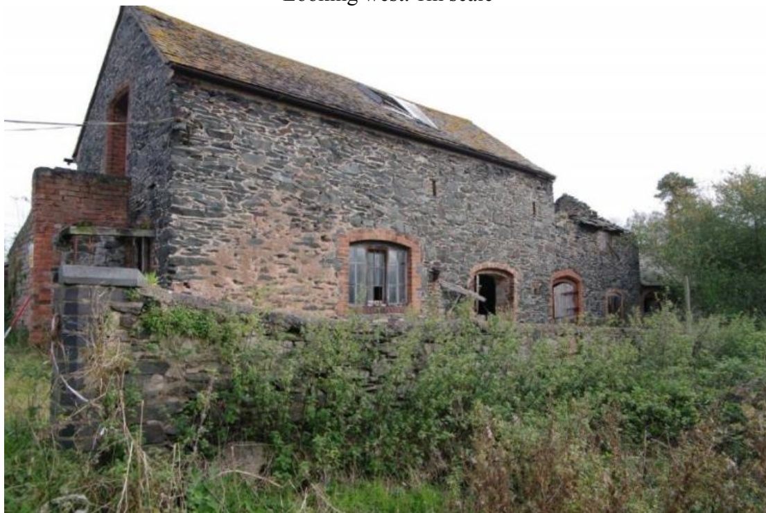
Figure 70 Building F south facing elevation Looking north-east from east yard
