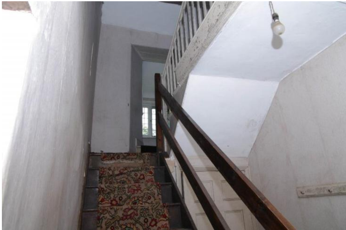
Figure 125 Stairs to first floor Looking west. Note how stairs lead to a lower landing before returning and rising to a higher landing
