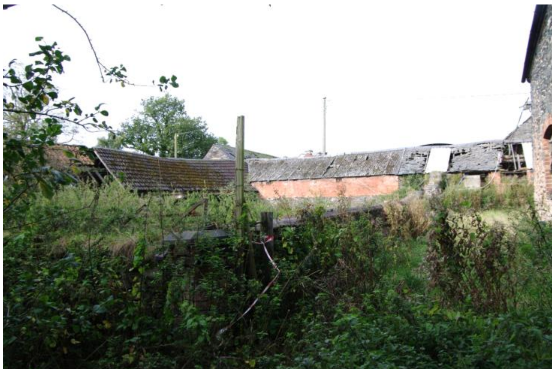
Figure 59 View of east yard Looking south-west towards Building D. Building E on left, F on right
