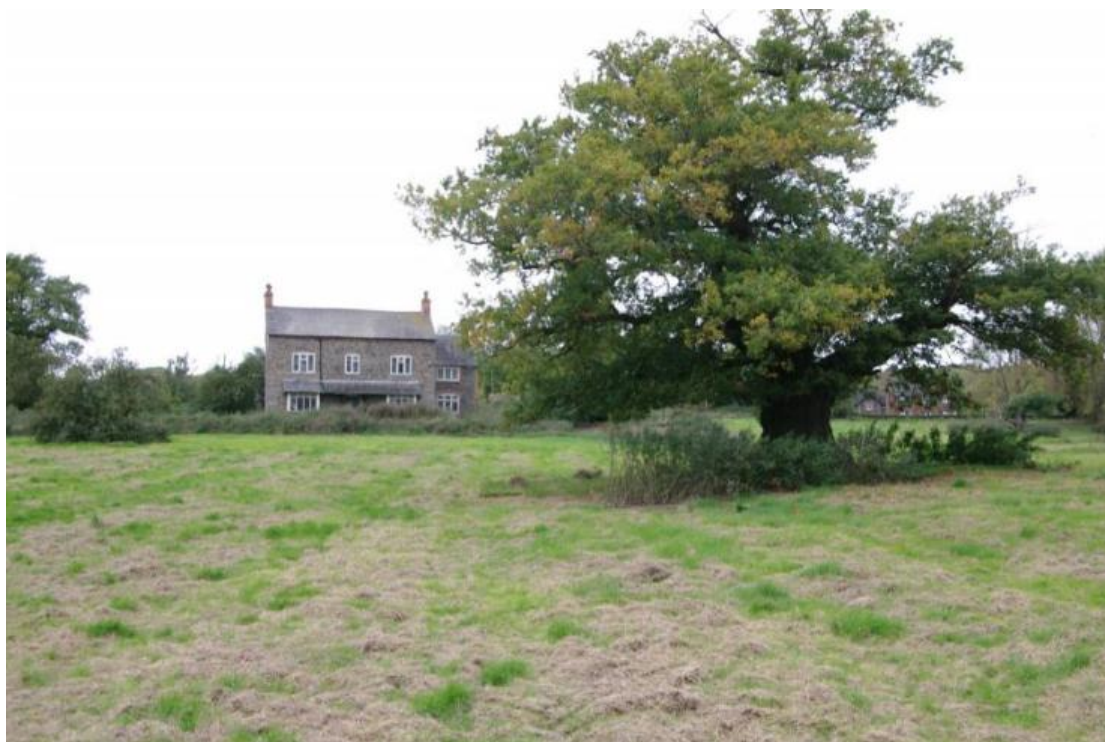
Figure 98 Main House east-facing elevation seen from across field Looking west. Markfield Road on right hand side of red brick house
