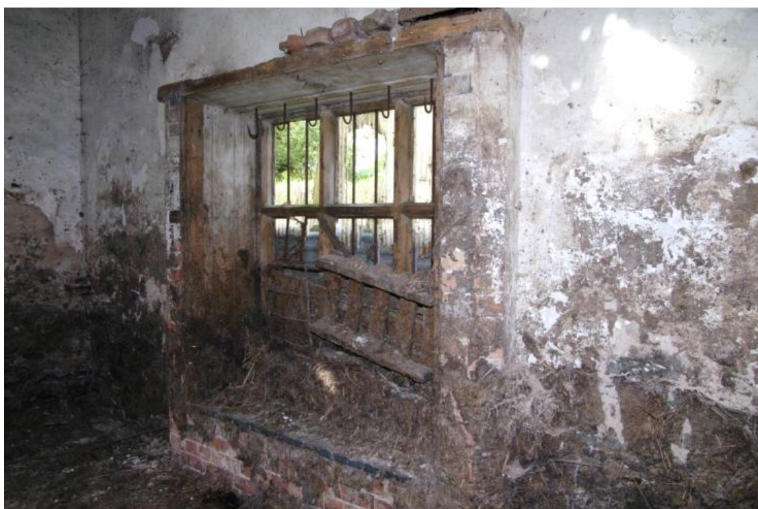
Figure 36 Building B north room, window detail Looking north-west
