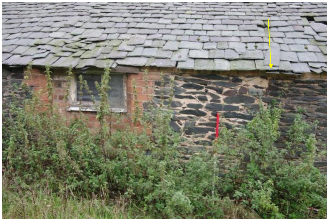
Figure 51 Building D west-facing elevation, blocked doorway Looking east. 1m scale. Yellow line indicates joint in stonework
