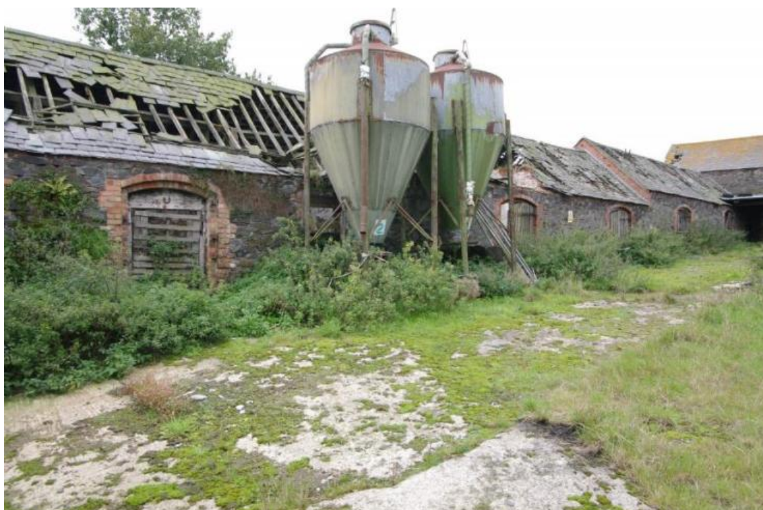
Figure 44 Building C north-facing elevation Looking south-east
