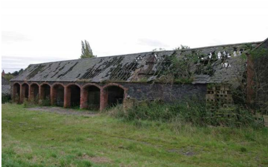
Figure 12 Building A north-facing elevation Looking south-east
