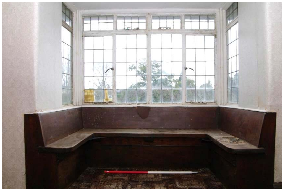
Figure 118 Room 7 bench and bay window detail Looking east. 1m scale
