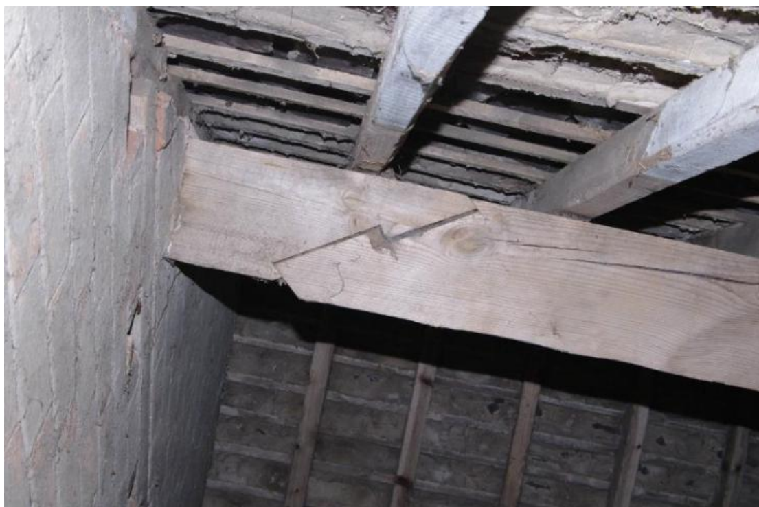
Figure 40 Building B first floor, scarf jointed purlin
