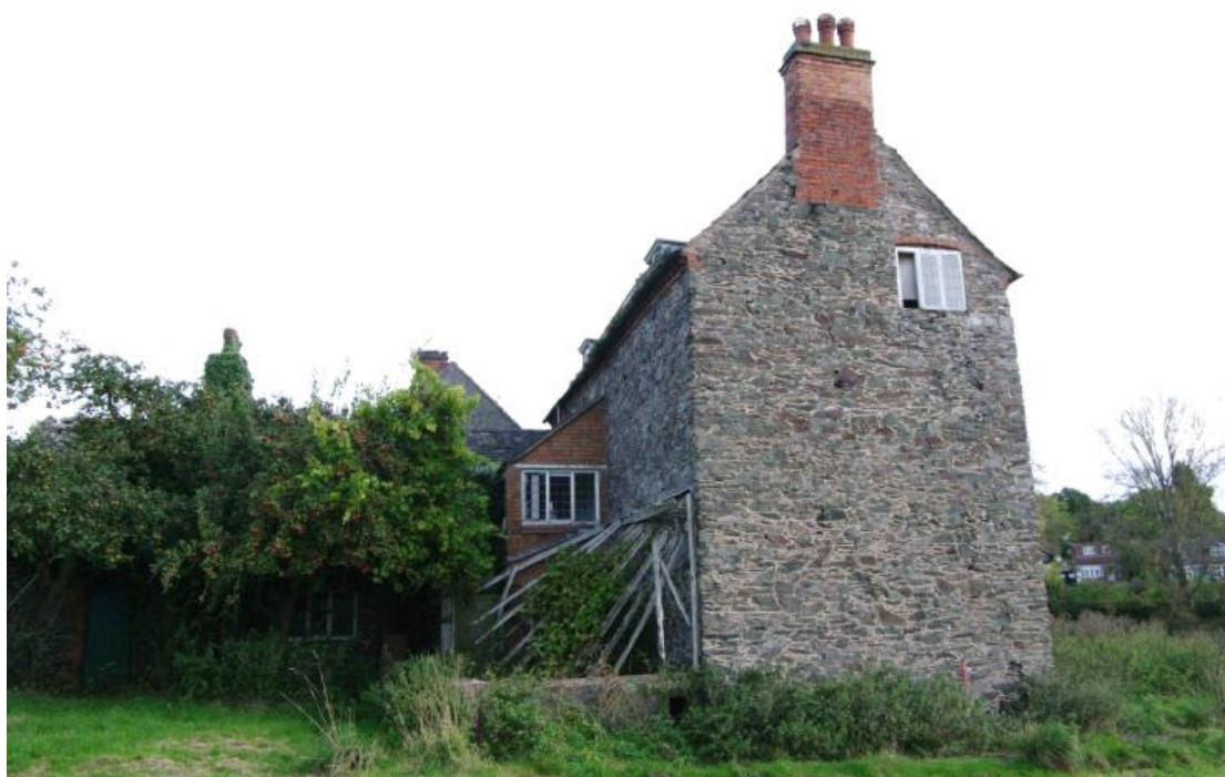
Figure 105 Main house south facing elevation Looking north
