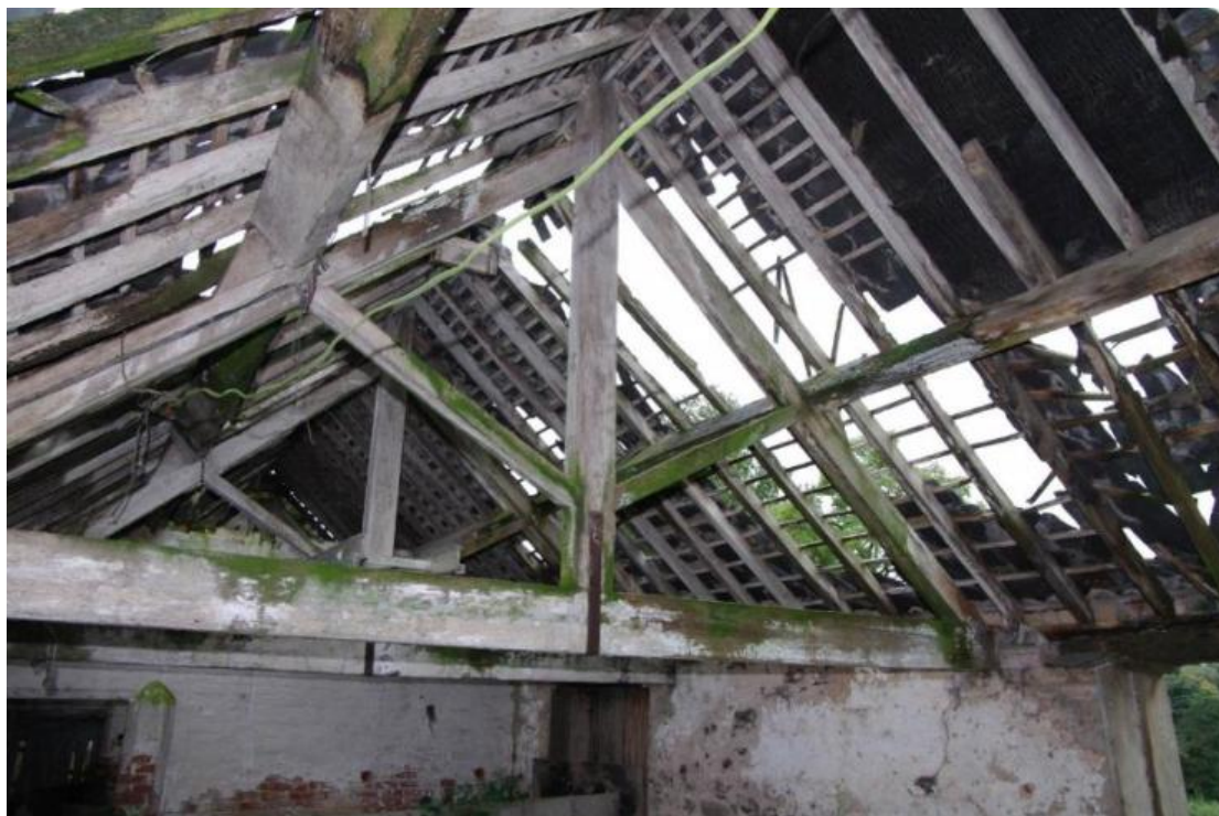
Figure 47 Building C roof structure Looking south-east from north end of building
