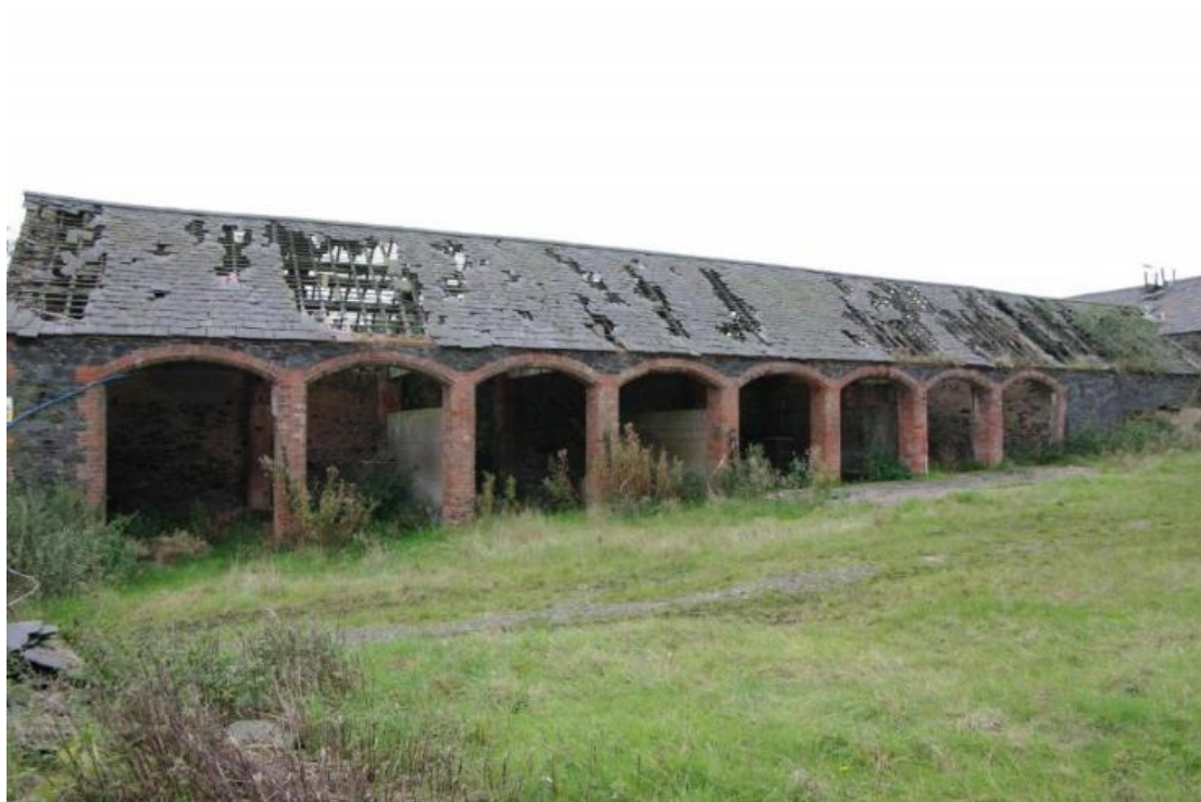
Figure 13 Building A north-facing elevation Looking south-west
