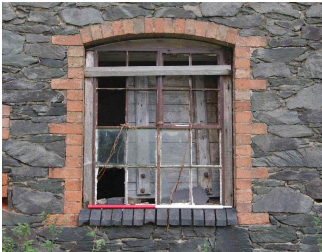
Figure 21 Building B west-facing elevation window detail Looking east. 1m scale
