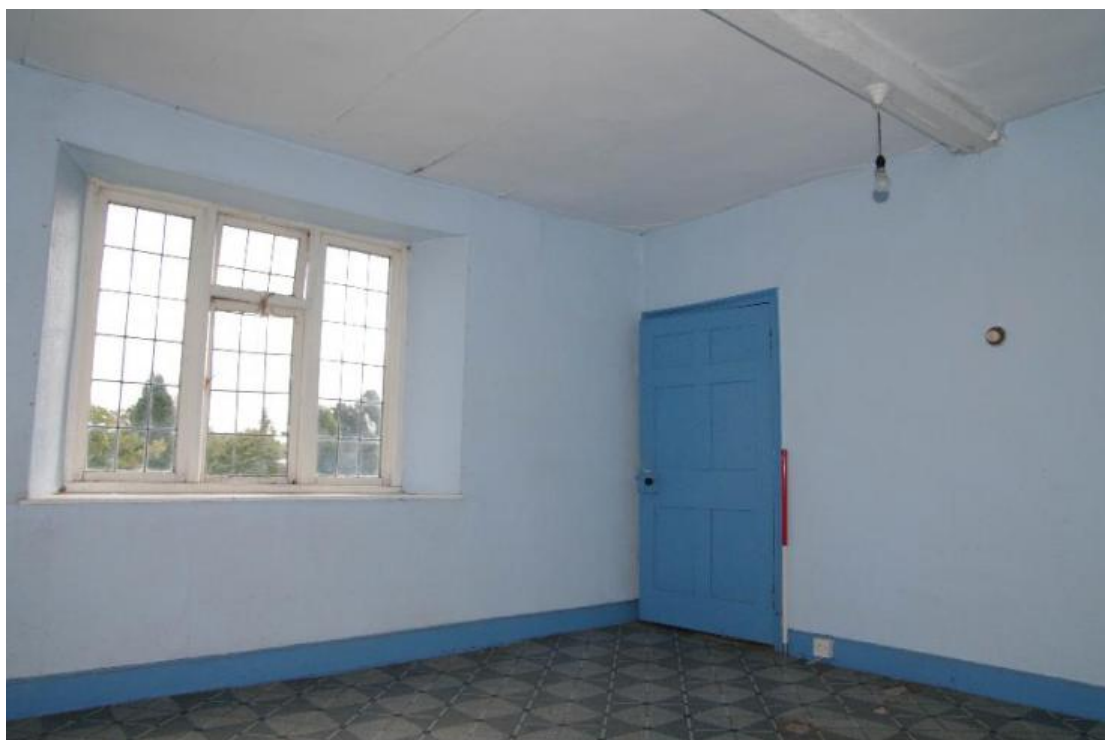
Figure 129 Room 13 Looking south-east. 1m scale
