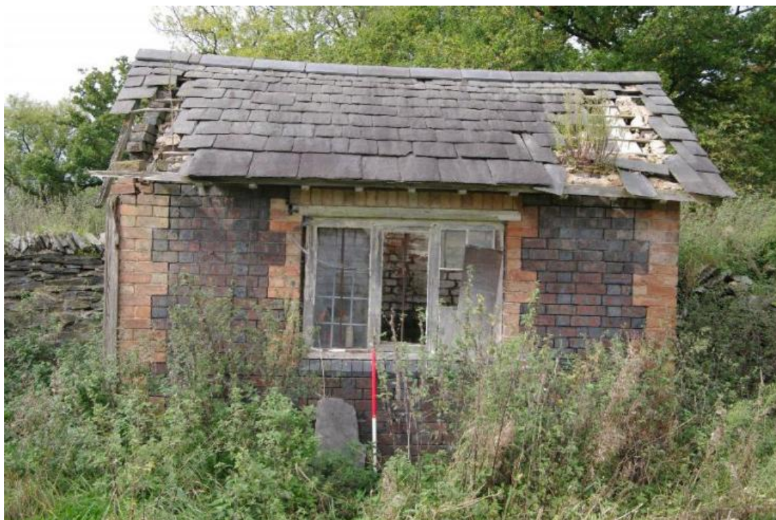
Figure 139 Weighbridge east-facing elevation Looking west. 1m scale
