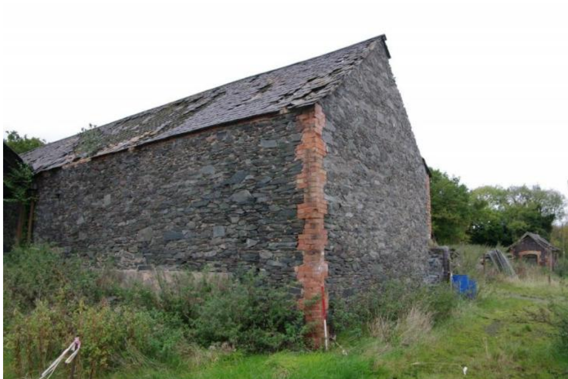
Figure 15 Building A east-facing gable and south-east corner Looking north-west. 1m scale
