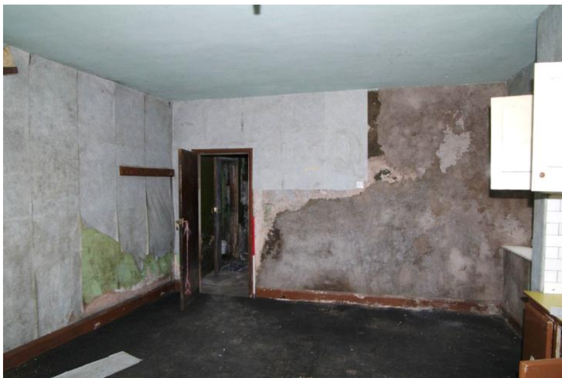
Figure 113 Room 5 Looking south-west. 1m scale. Door to Room 4 in corner
