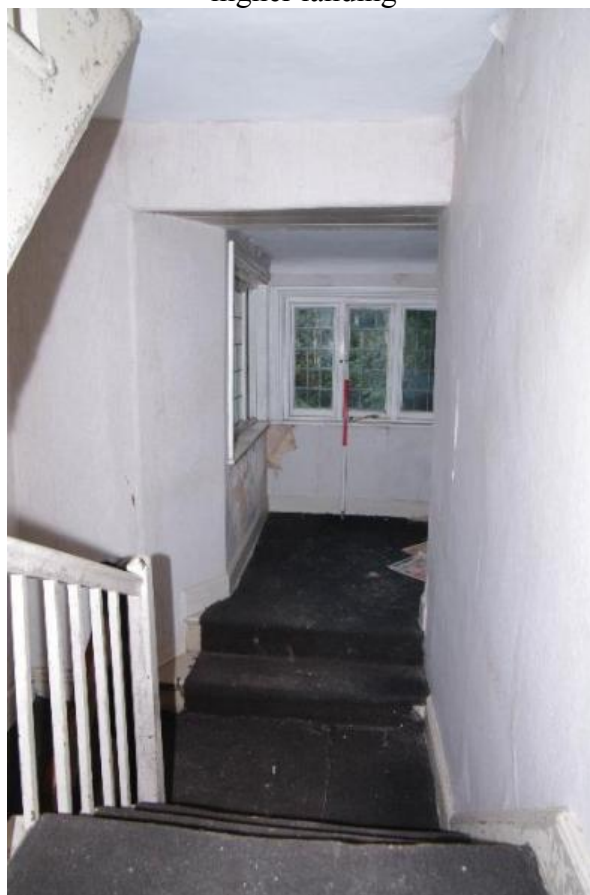
Figure 126 Stairs to landing along rear extension Looking west from original landing. 1m scale. Rear extension reached by following the landing to the right of the scale
