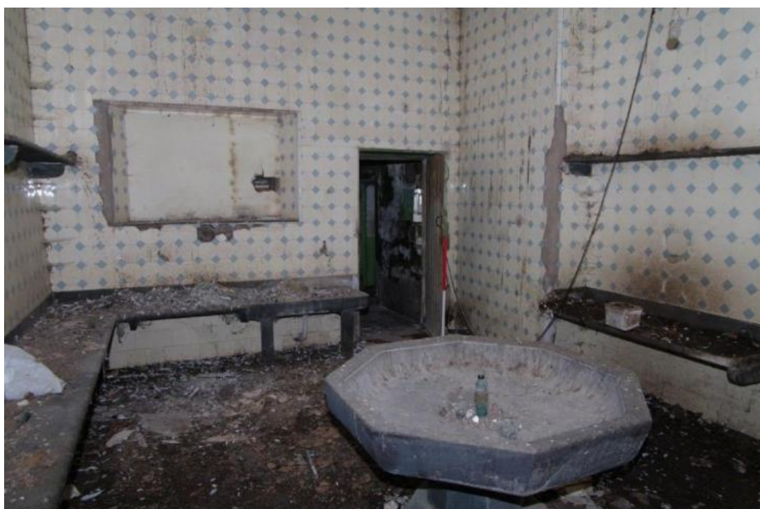
Figure 90 Building G creamery Looking south-east. 1m scale
