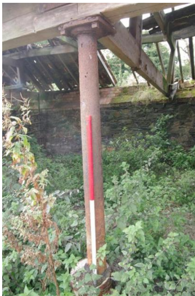
Figure 61 Building E north-facing elevation, column detail Looking south-east. 1m scale
