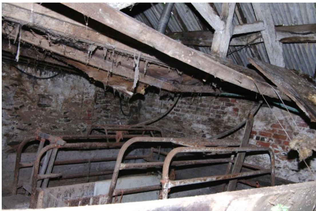
Figure 56 Building D inside southern room Looking north-east. Photo taken from doorway
