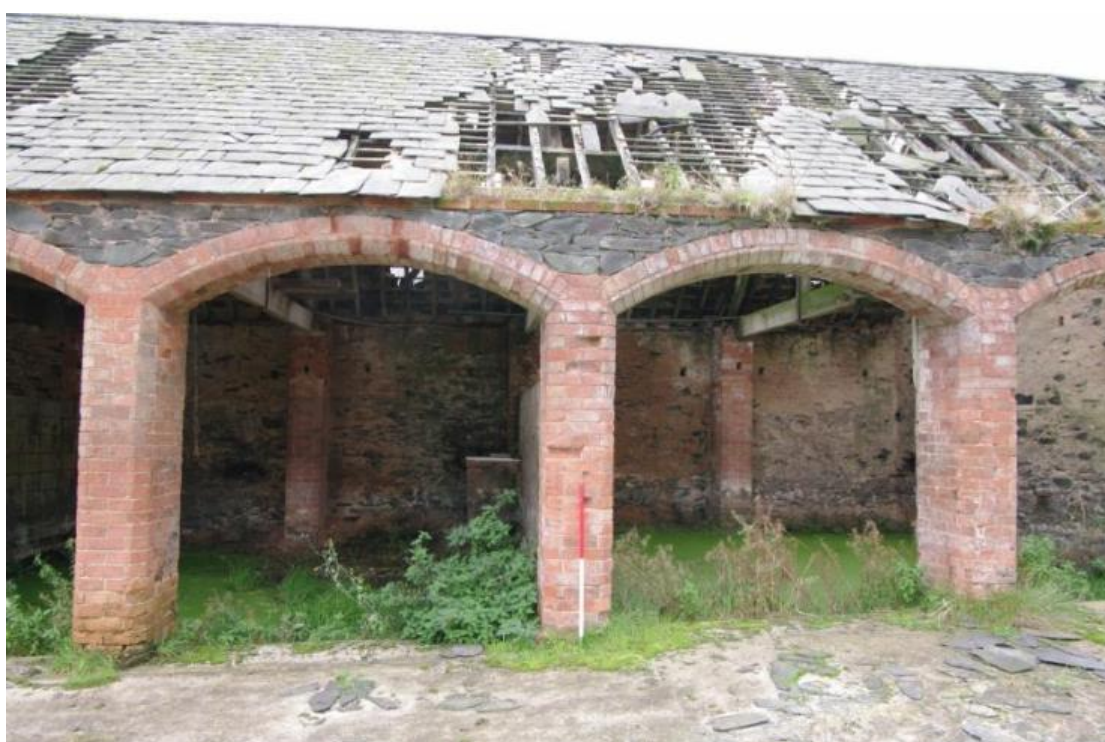
Figure 14 Building A north-facing elevation brickwork detail Looking south. 1m scale
