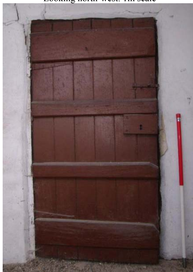
Figure 137 Attic Room 15 door detail Looking south. 1m scale
