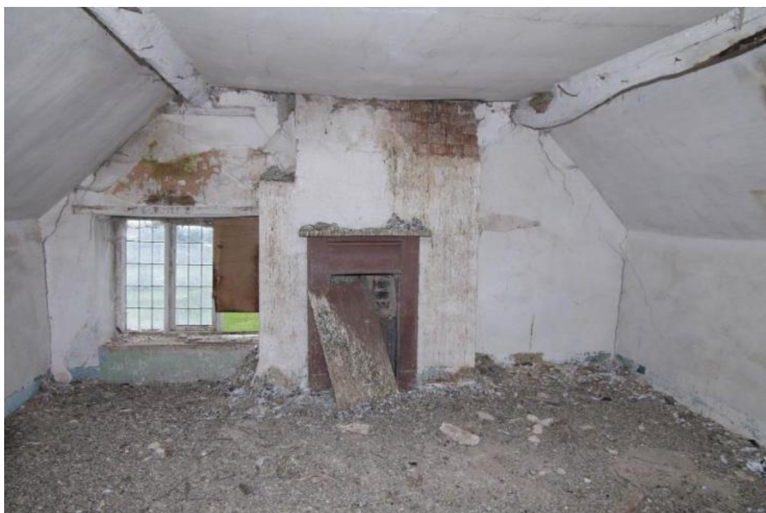
Figure 138 Attic Room 16 Looking south
