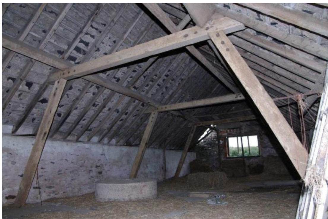
Figure 38 Building B first floor Looking south-east. Note millstone centre left and sack hatch to right of stones
