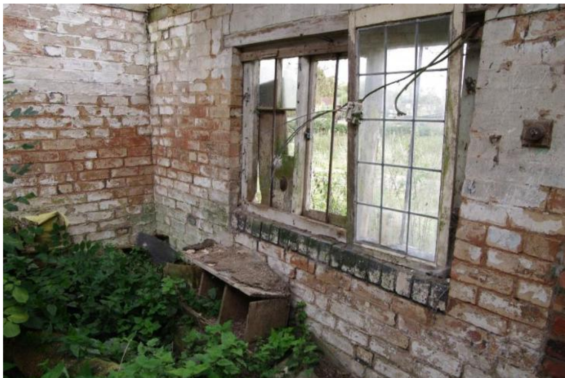
Figure 141 Inside the weighbridge Looking north-east
