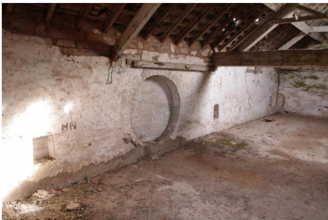
Figure 75 Building F first floor Looking north-east
