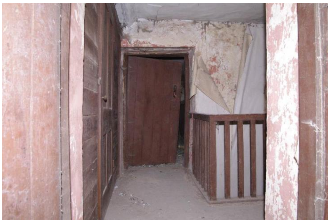
Figure 135 Attic landing Looking south towards Room 16. Linen cupboard on left
