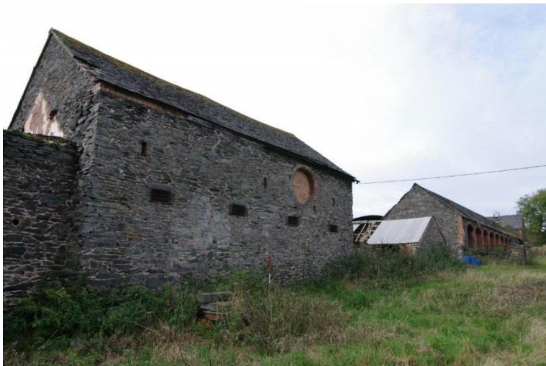
Figure 67 Building F north-facing elevation Looking south-west. 1m scale
