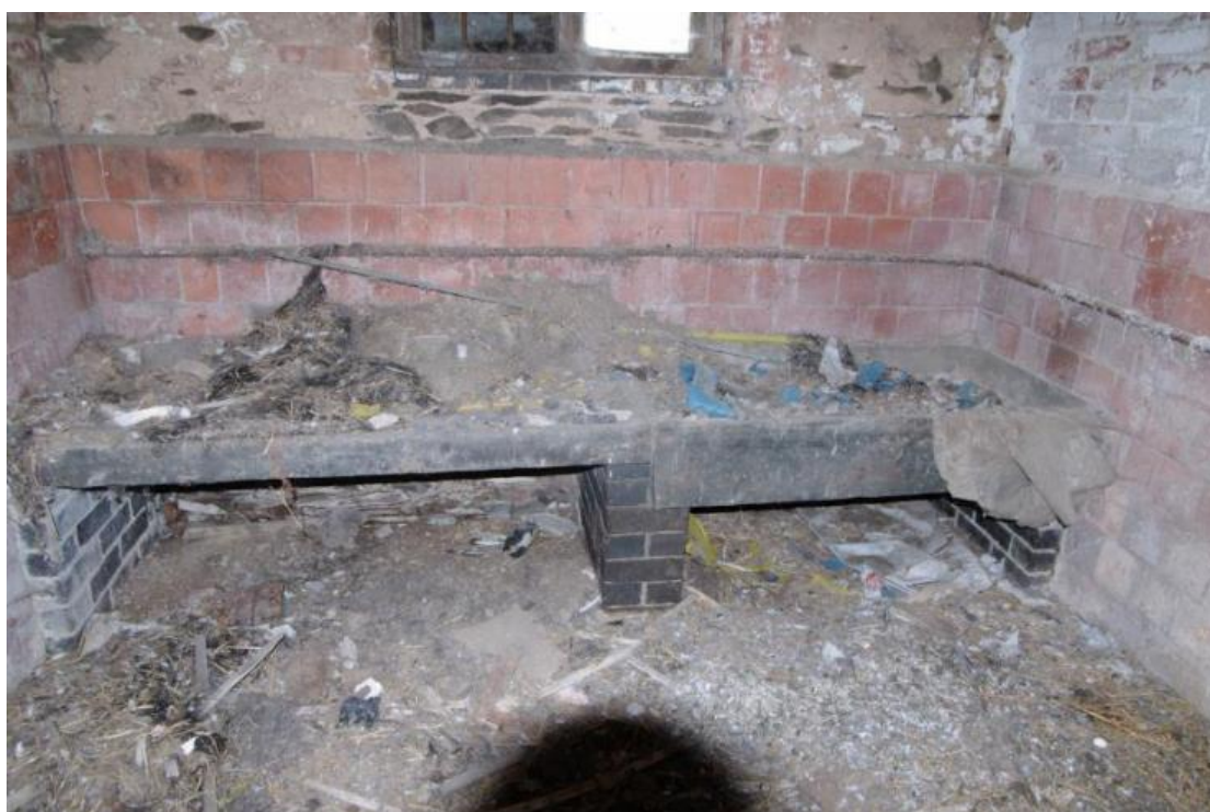
Figure 86 Building G slate troughs Looking north
