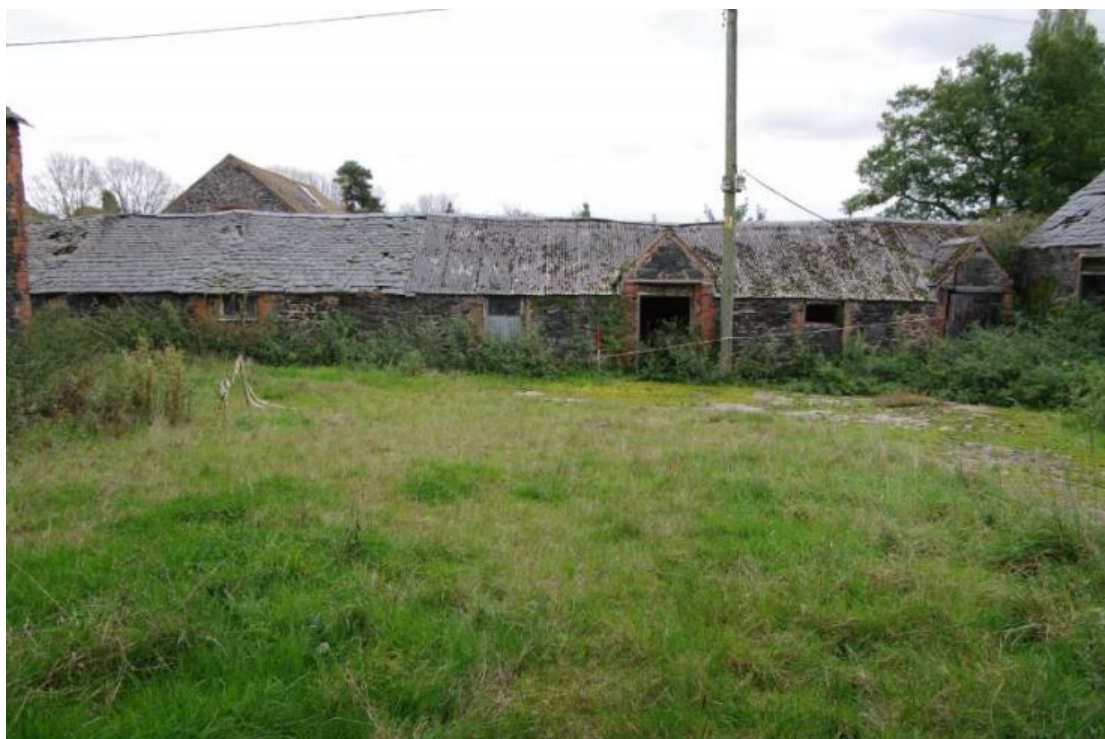
Figure 48 Building D west-facing elevation Looking east. 1m scale
