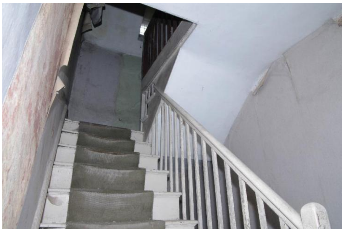
Figure 134 Stairs to attic rooms Looking west from first floor landing
