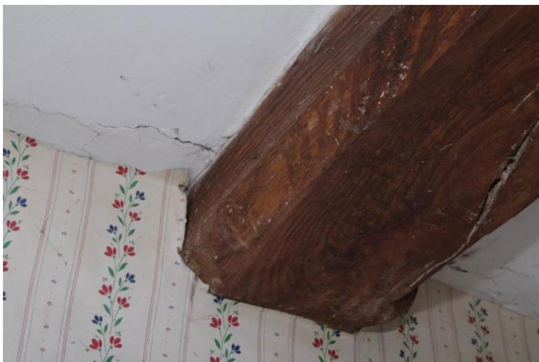
Figure 133 Room 14 stops on beam
