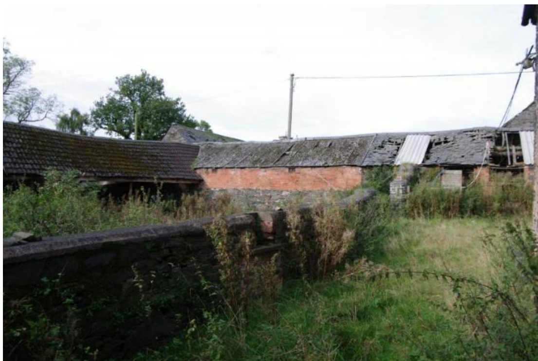
Figure 53 Building D east-facing elevation Looking south-west. Building E on left
