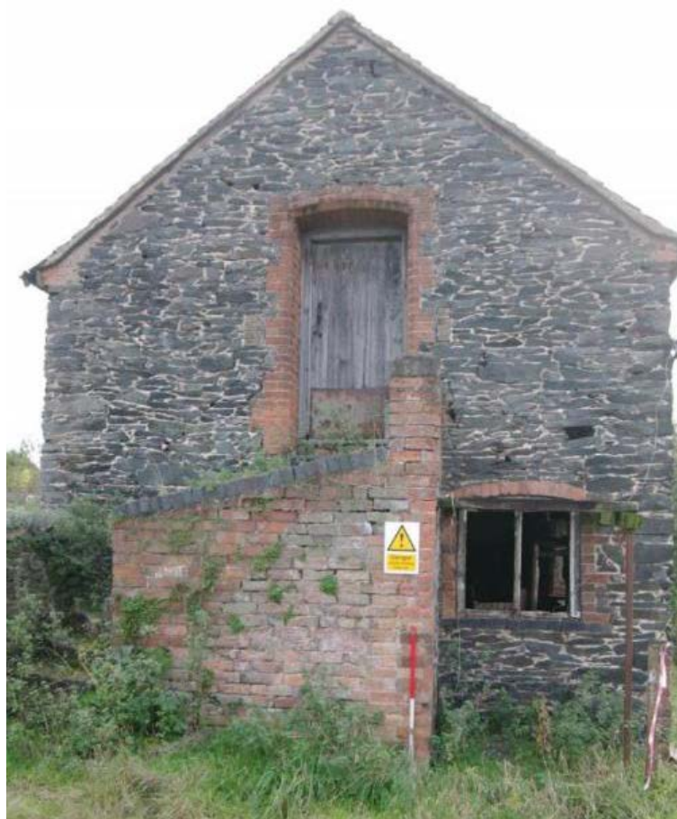
Figure 69 Building F west-facing elevation Looking west. 1m scale
