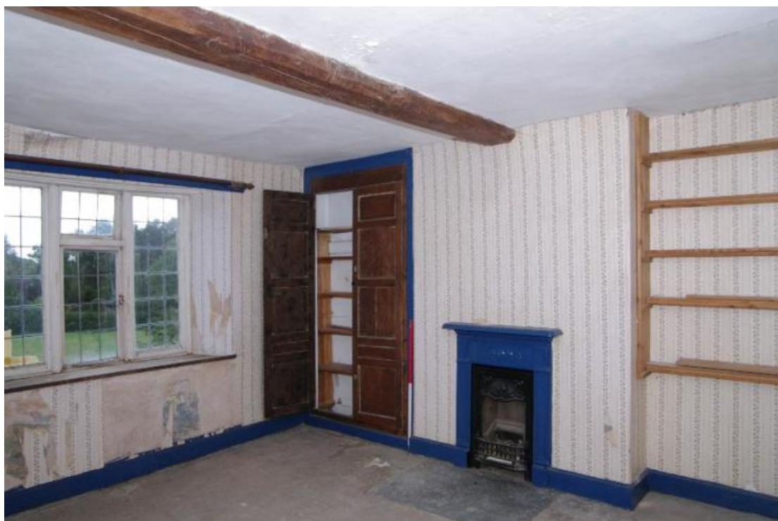
Figure 131 Room 14 Looking south-west. 1m scale
