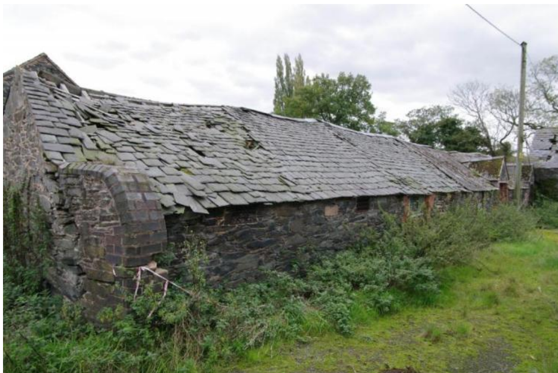
Figure 49 Building D west-facing elevation, north end Looking south-east
