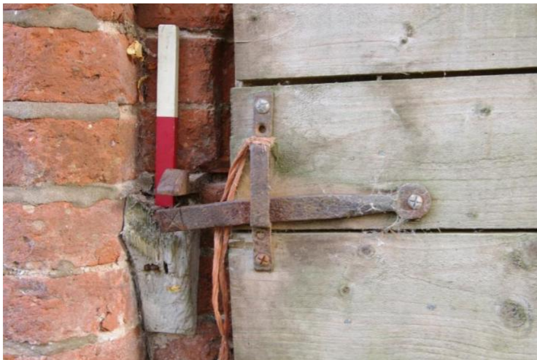
Figure 81 Building G south facing elevation latch detail 0.2m scale. Note use of modern screw fixings
