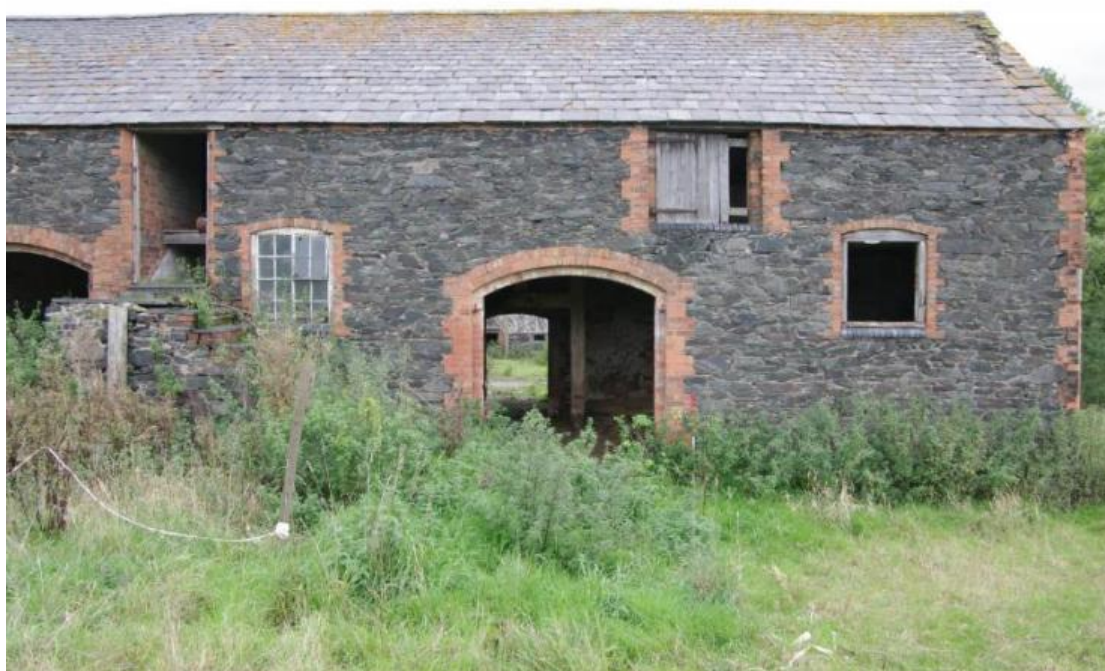
Figure 22 Building B south end of west-facing elevation Looking east. 1m scale
