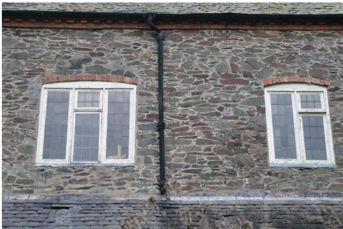
Figure 102 Main House east-facing elevation first floor window detail Looking west
