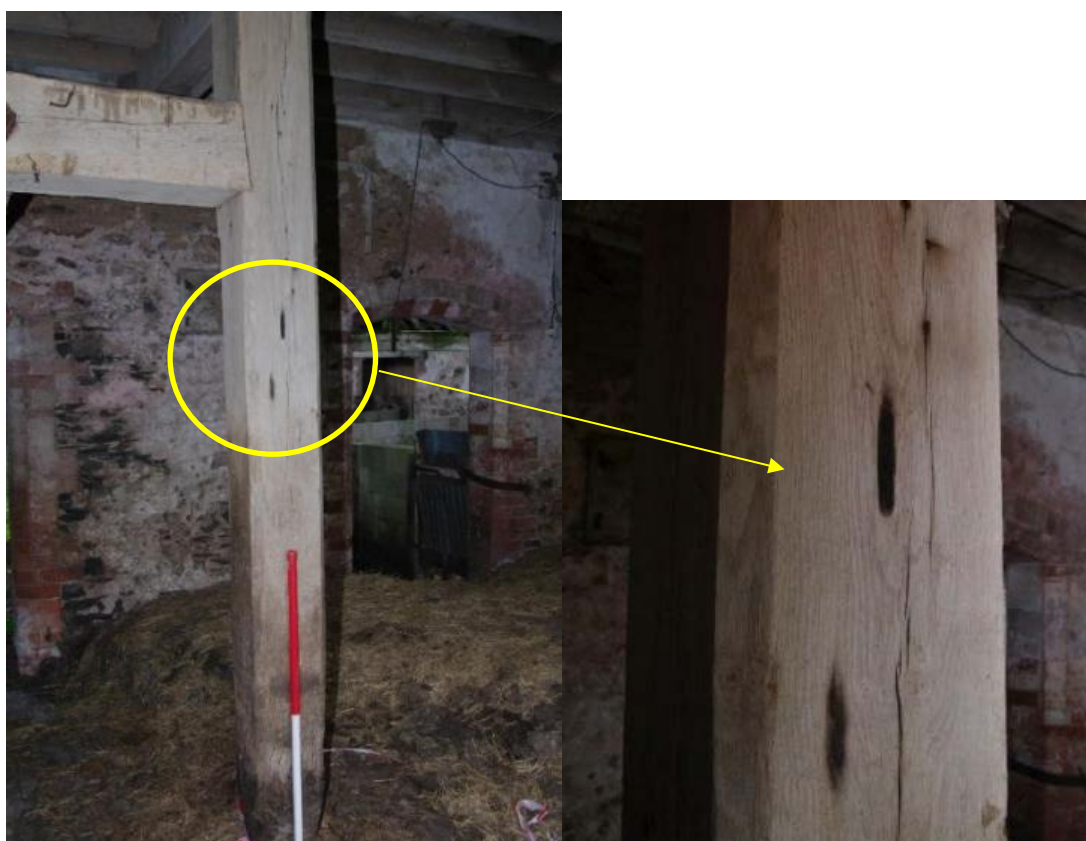
Figure 32 Building B ground floor south room possible apotropaic scorch marks Looking south-east. 1m scale in main picture. See also Figure 27
