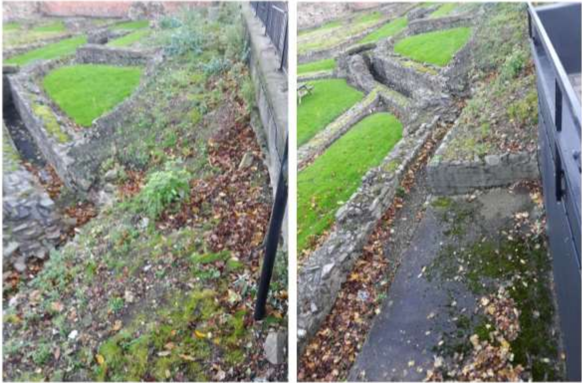
Figure 6: Views of the investigation area (looking east), prior to start
