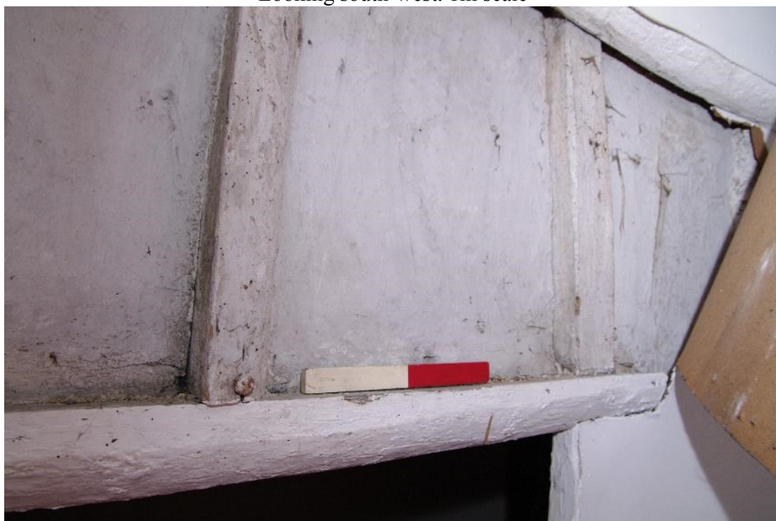
Figure 106 Room 19 stud walling Looking south-east. 0.2m scale. Door lintel across bottom left of picture
