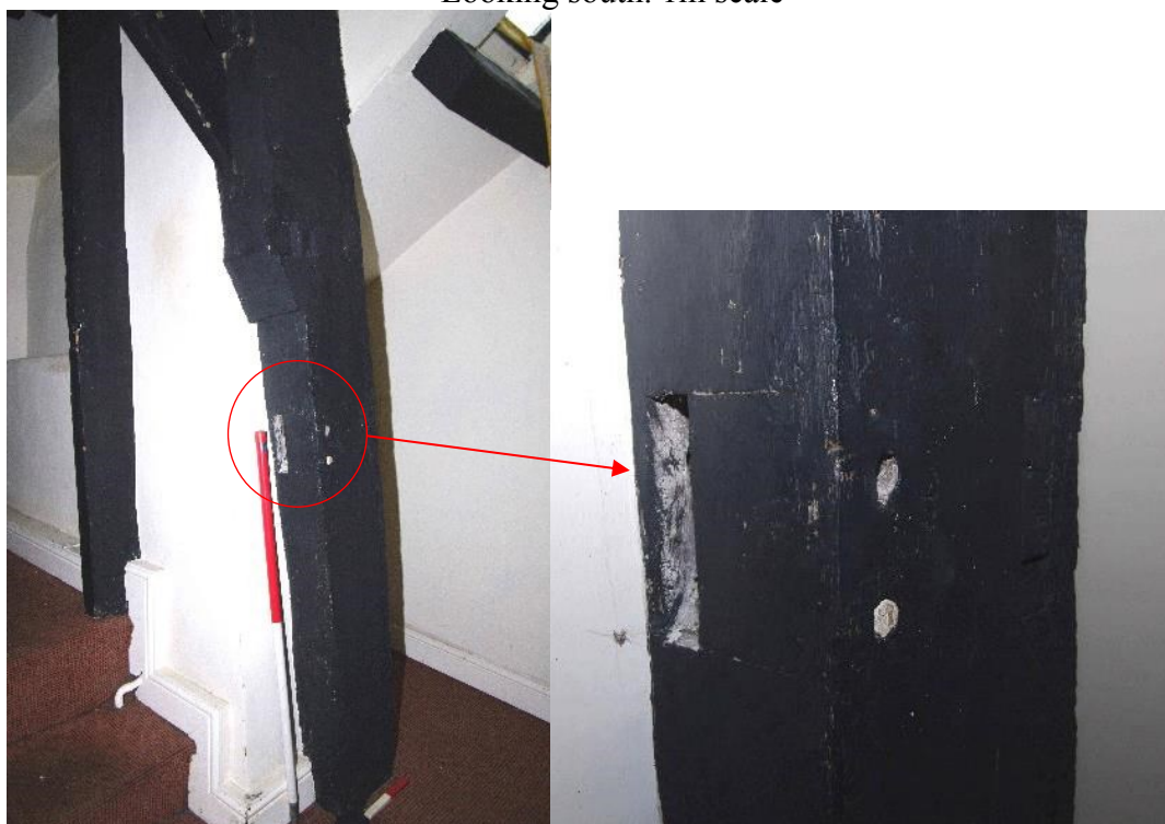
Figure 87 Corridor 12 large timber post near staircase Looking west. 1 and 0.2m scales. Note empty mortice and peg holes near to top of 1m scale, also shown in inset picture
