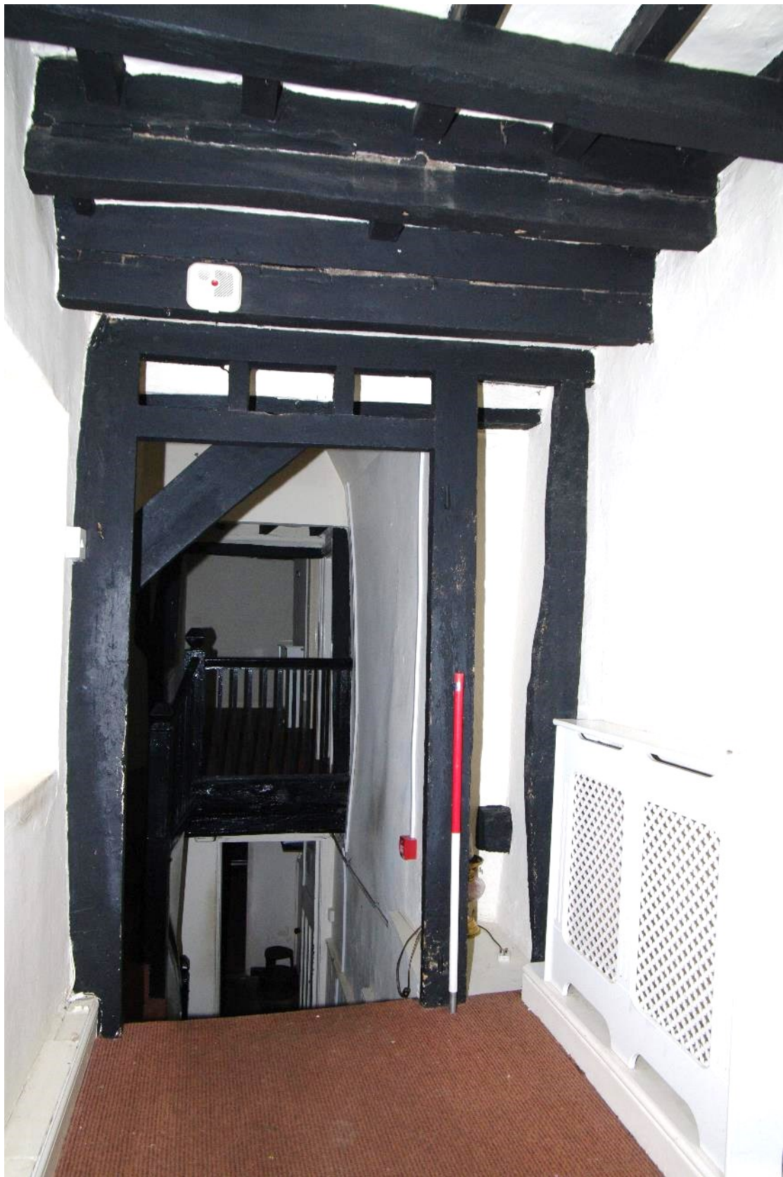
Figure 88 Corridor 12 timber stud walling Looking north. 1m scale
