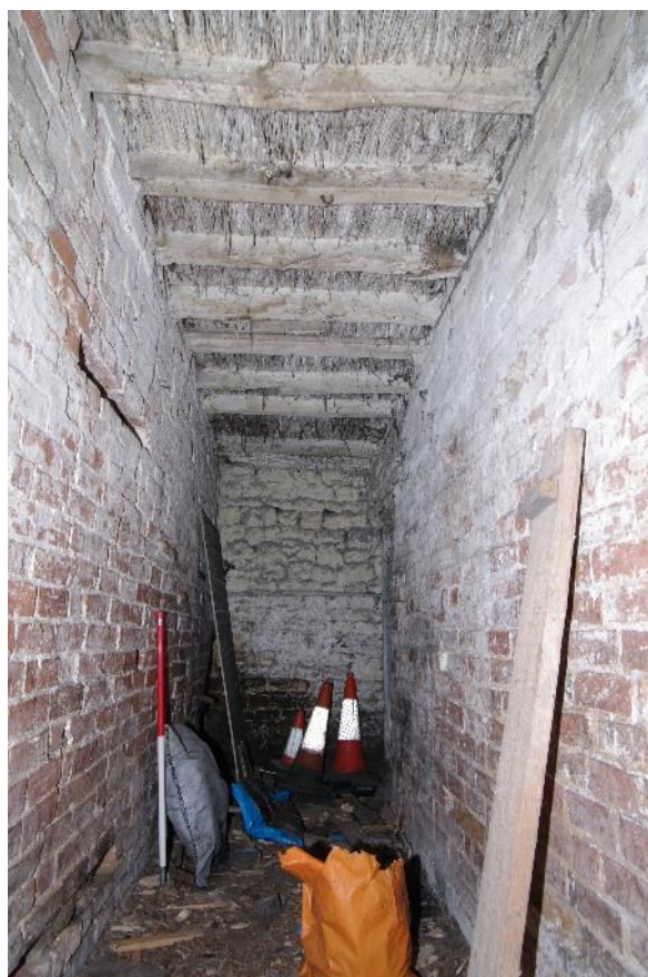
Figure 77 Room 10 coal store Looking east. 1m scale. Note reed and plaster ceiling
