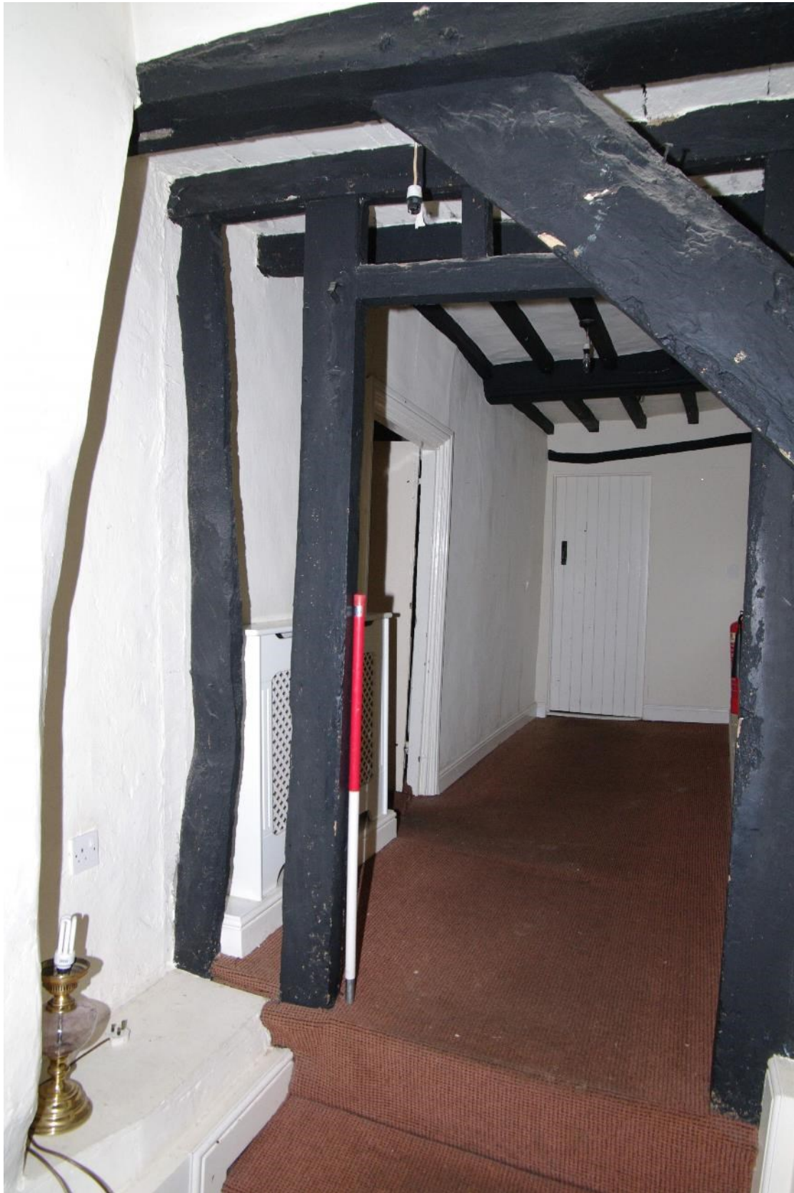
Figure 89 Corridor 12 timber stud walling Looking south. 1m scale. Note redundant mortice hole in closer beam
