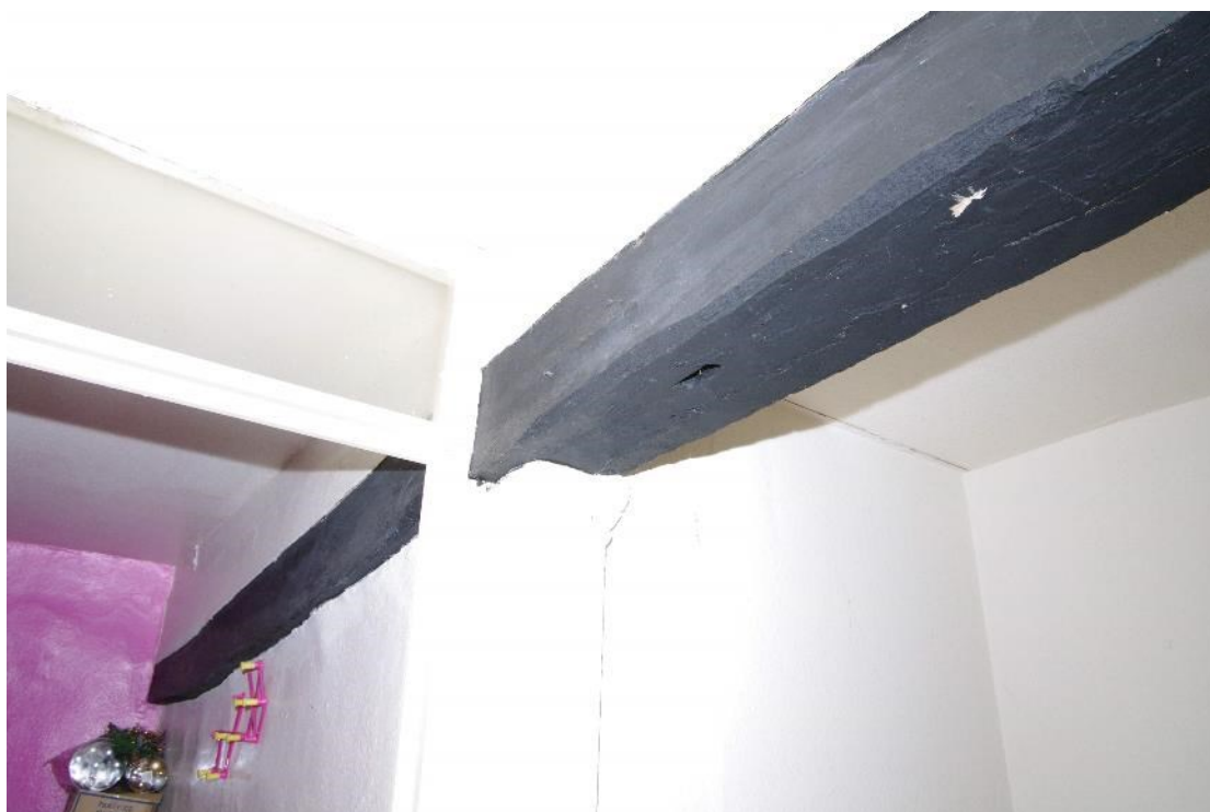
Figure 103 Beam extending from Room 18 across Corridor 12 Looking south-west. Note redundant socket on underside of beam
