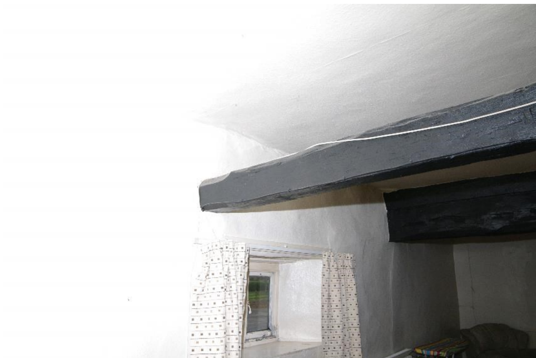
Figure 111 Room 20 smaller east to west beam Looking west. Larger axial beam to right
