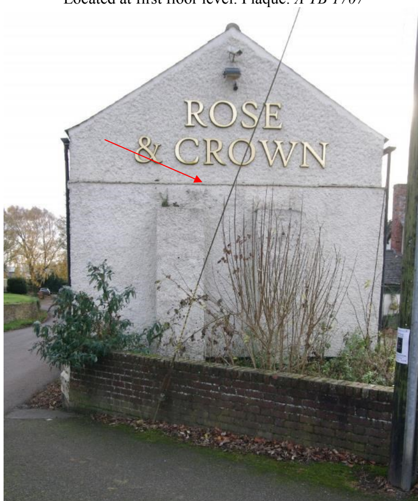
Figure 21 North-facing gable end of principal range Looking south. Main Street on left. Note scar (arrowed) left by demolished building
