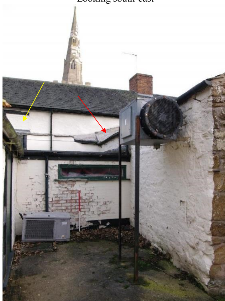
Figure 27 West-facing elevation between both east to west ranges Looking east. 1m scale. Blocked window (yellow) and structural timbers (red)
