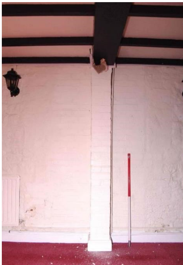
Figure 73 Room 9 pilaster over blocked doorway Looking north. 1m scale
