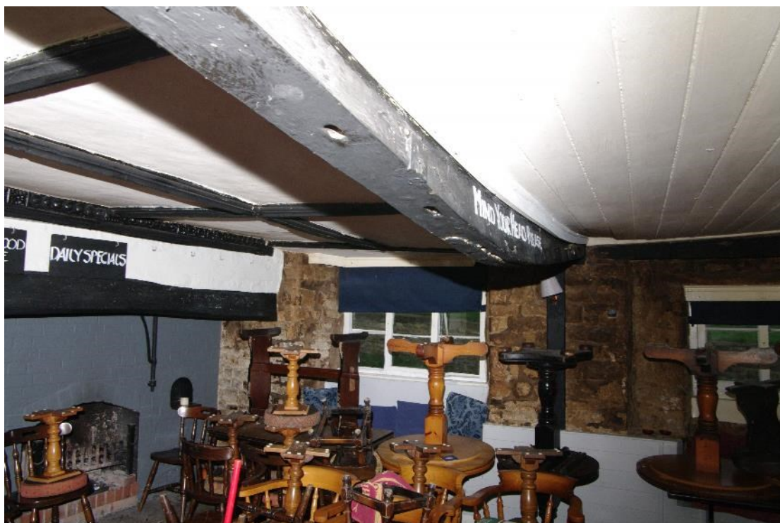
Figure 51 Room 2 axial beam above former cross wall Looking west. Note holes for uprights for wattle panels
