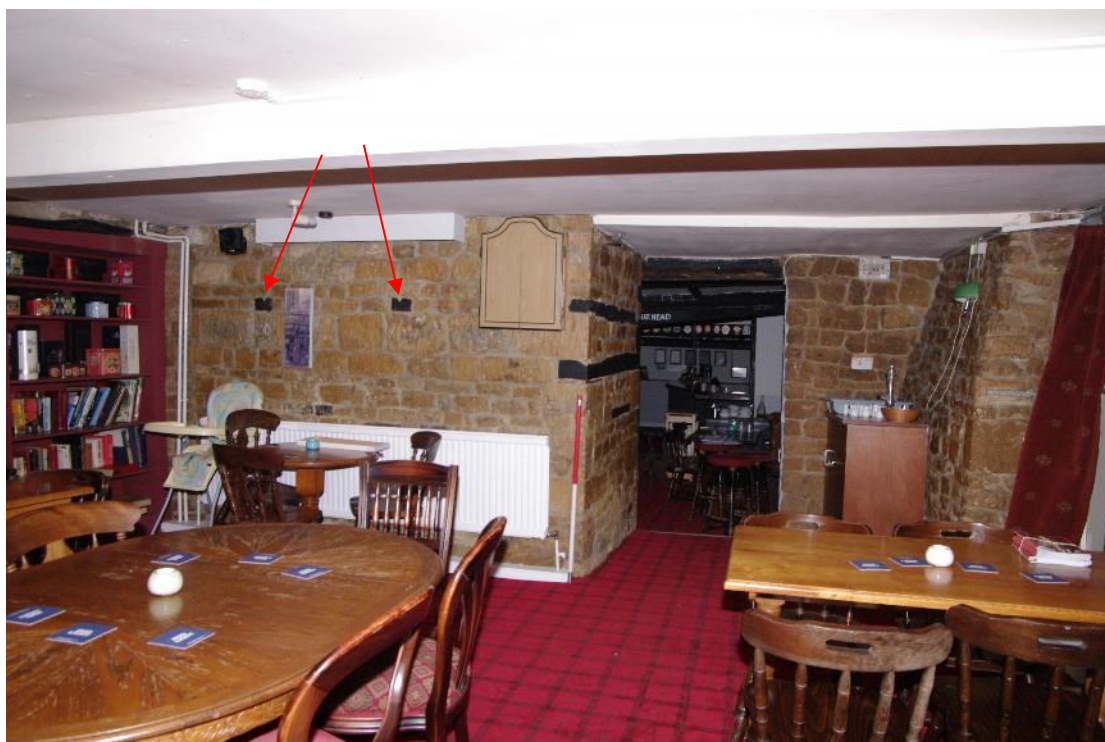
Figure 42 Room 1 Looking west towards doorway to Room 1. 1m scale. Bookcase on left fills the gap of a former doorway. Note V-shaped timbers on chimney breast (arrowed)
