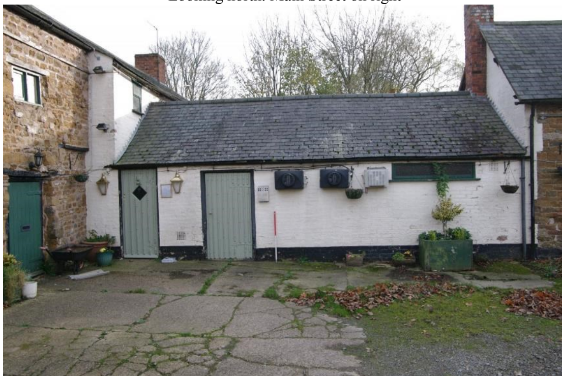
Figure 33 North-facing elevation of east to west stable range, eastern end Looking south. 1m scale. Note how N-S range construction changes from stone to brick and steps out at this point
