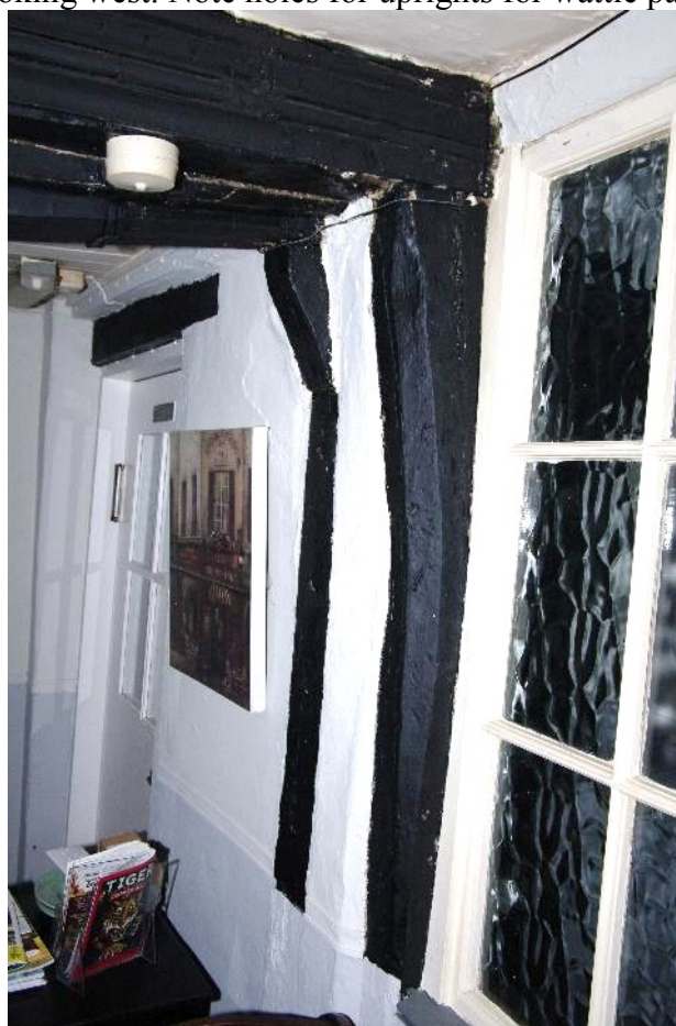
Figure 52 Room 2 supporting posts for axial beams Closest, chamfered, beam supports the smaller beam with carved cornice, the further beam supports the former cross wall beam
