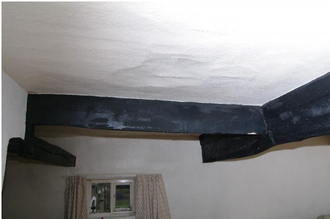
Figure 110 Room 20 thin beam from axial beam to chimney breast Looking west
