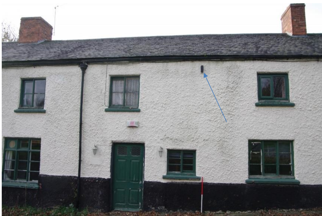
Figure 15 East-facing elevation, front door Looking west. 1m scale. Note projecting timber beam (arrowed)
