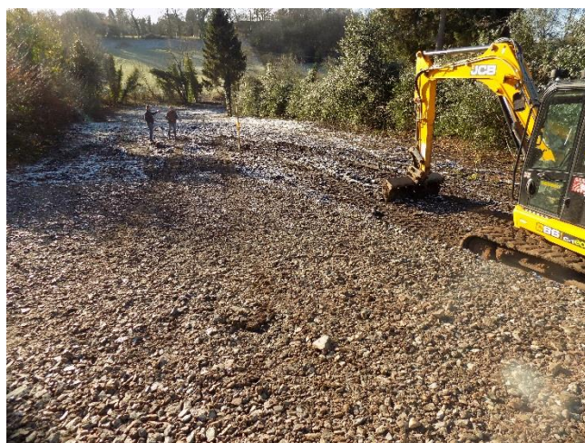
a. South facing view of assessment area
