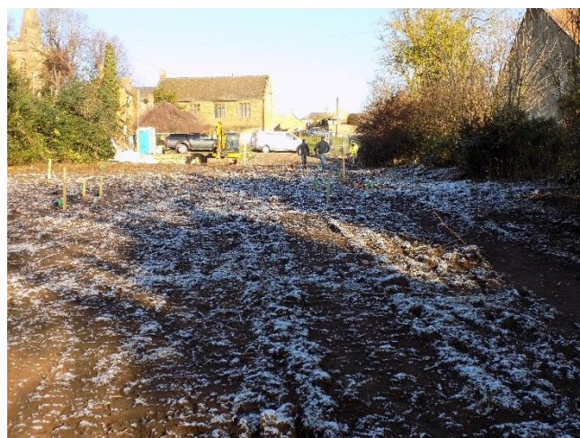
b. North facing view of assessment area
