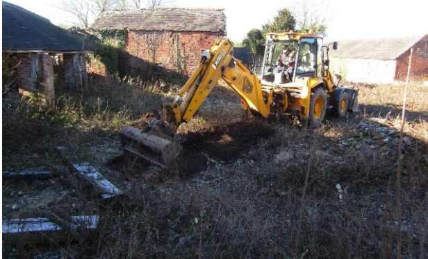
Figure 4: Maching Trench 03, looking west
