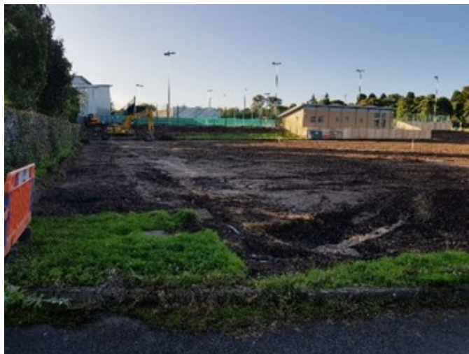
Figure 5: Looking south-east from the north-western extent of the site
