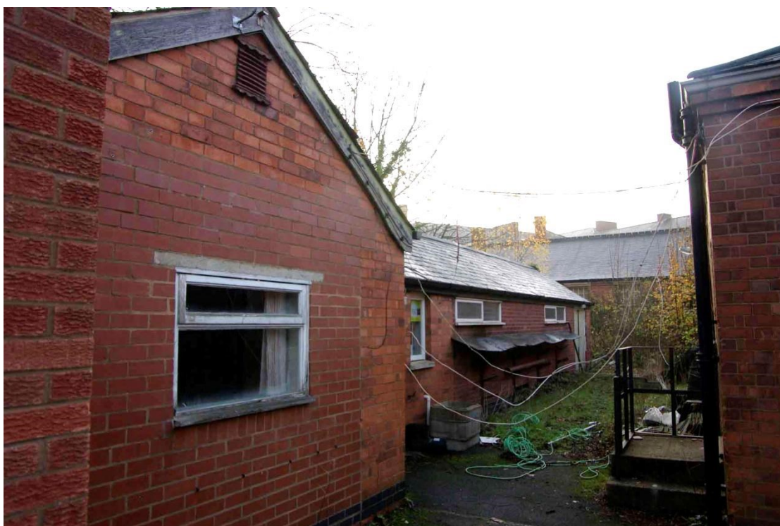
Figure 66 Workshop WS5 Looking south-east. Workshop WS3 on right of photo
