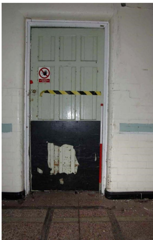
Figure 38 Main corridor doorway into the engineering block Looking north, 1m scale
