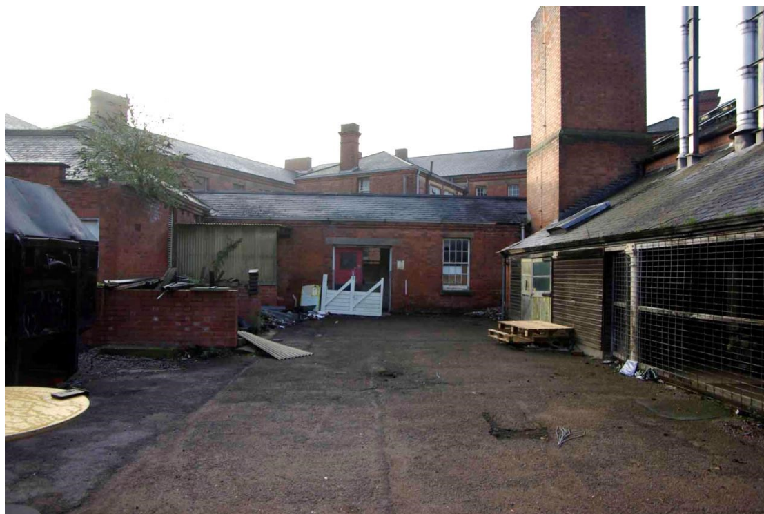
Figure 24 North elevation of main corridor adjacent to boiler house
