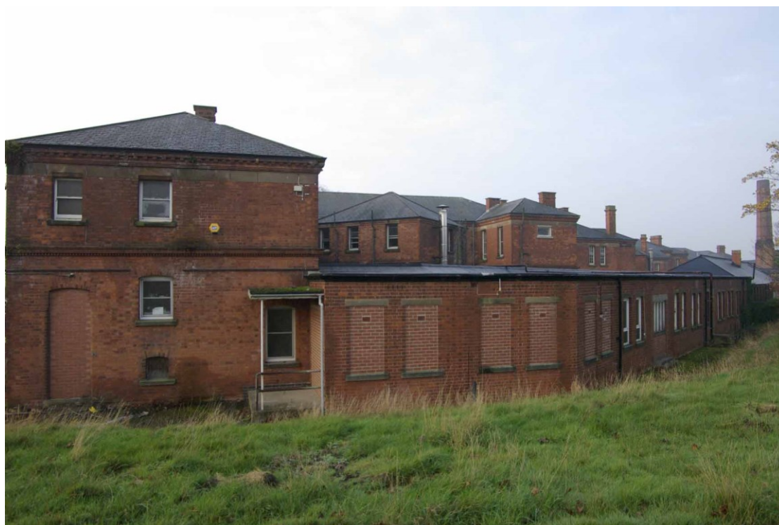
Figure 23 East end of main corridor
