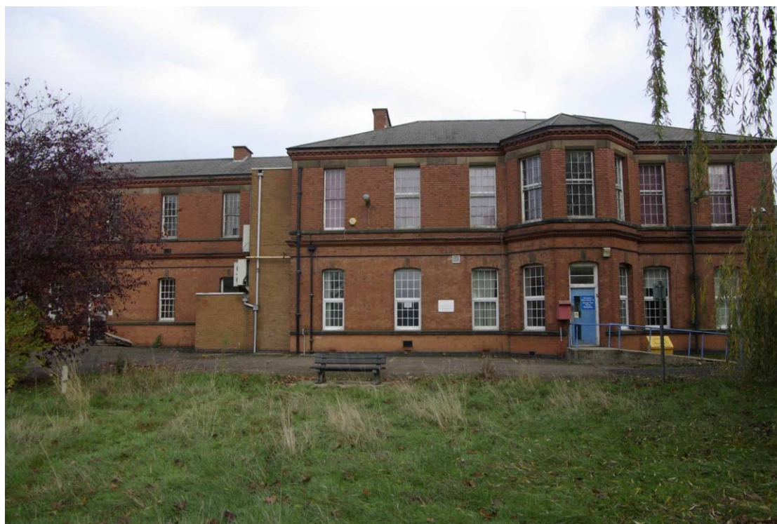
Figure 90 East end of Daisy Peake Building. Fosse and Belgrave wards Looking north. Inserted lift shaft centre left
