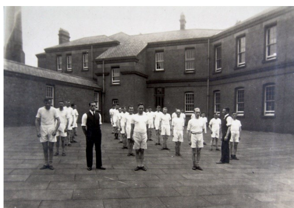
Figure 98 Courtyard behind Beaumanor ward Looking east. Angled and main corridors on left Lower picture same view during exercise in the 1930s
