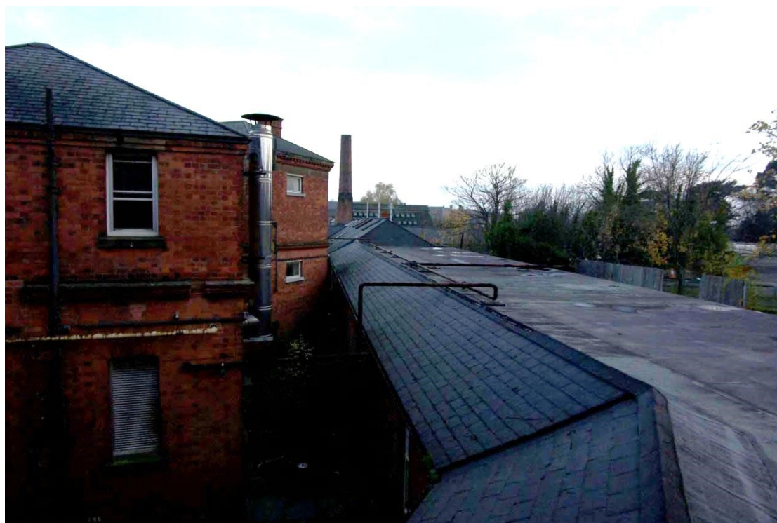
Figure 18 View of corridor roof at eastern end
