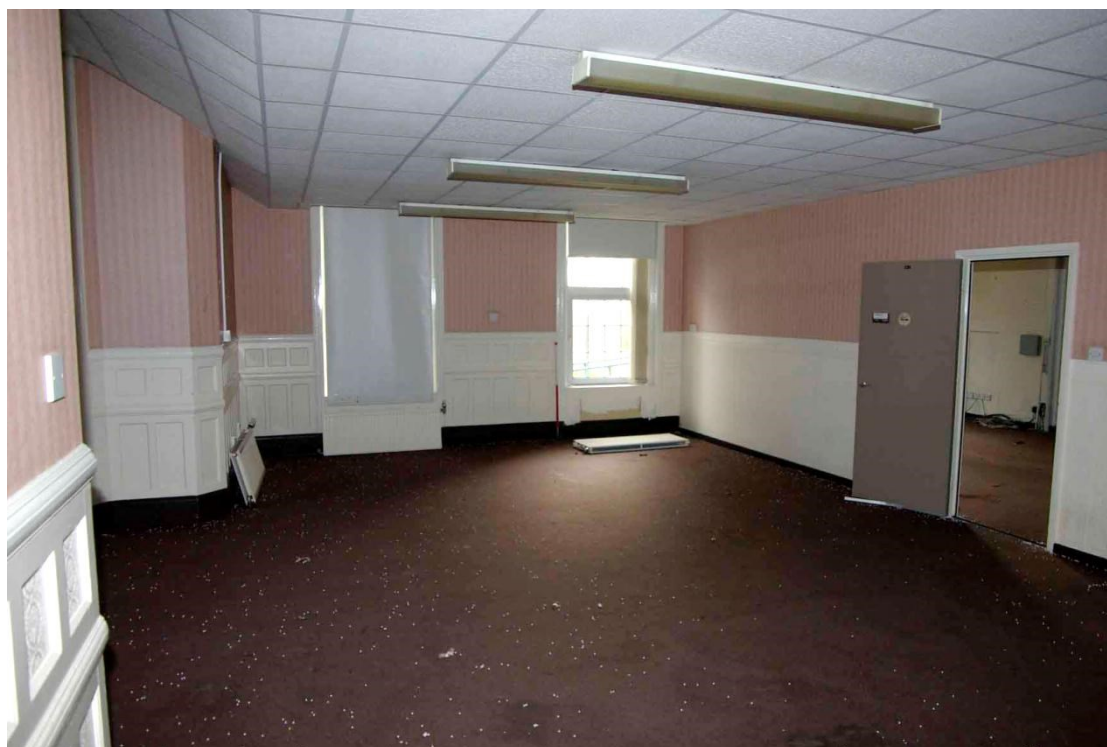
Figure 104 Fosse ward dayroom Looking south-west, 1m scale. Note inserted plasterboard wall on right
