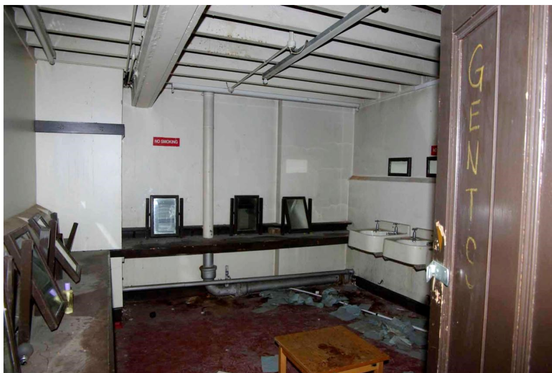
Figure 125 Men's changing room below stage
