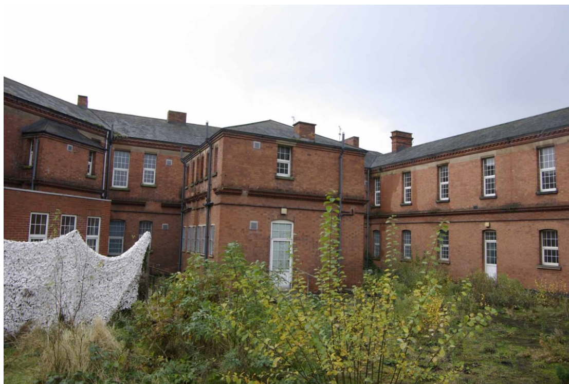
Figure 99 Courtyard behind Beaumanor ward and offices Looking south-west
