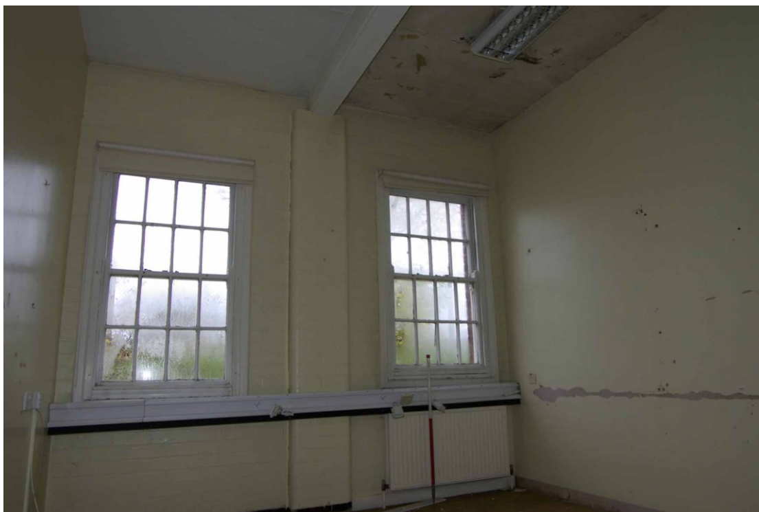
Figure 34 Re-used sash windows in 1940s extension Looking north, 1m scale
