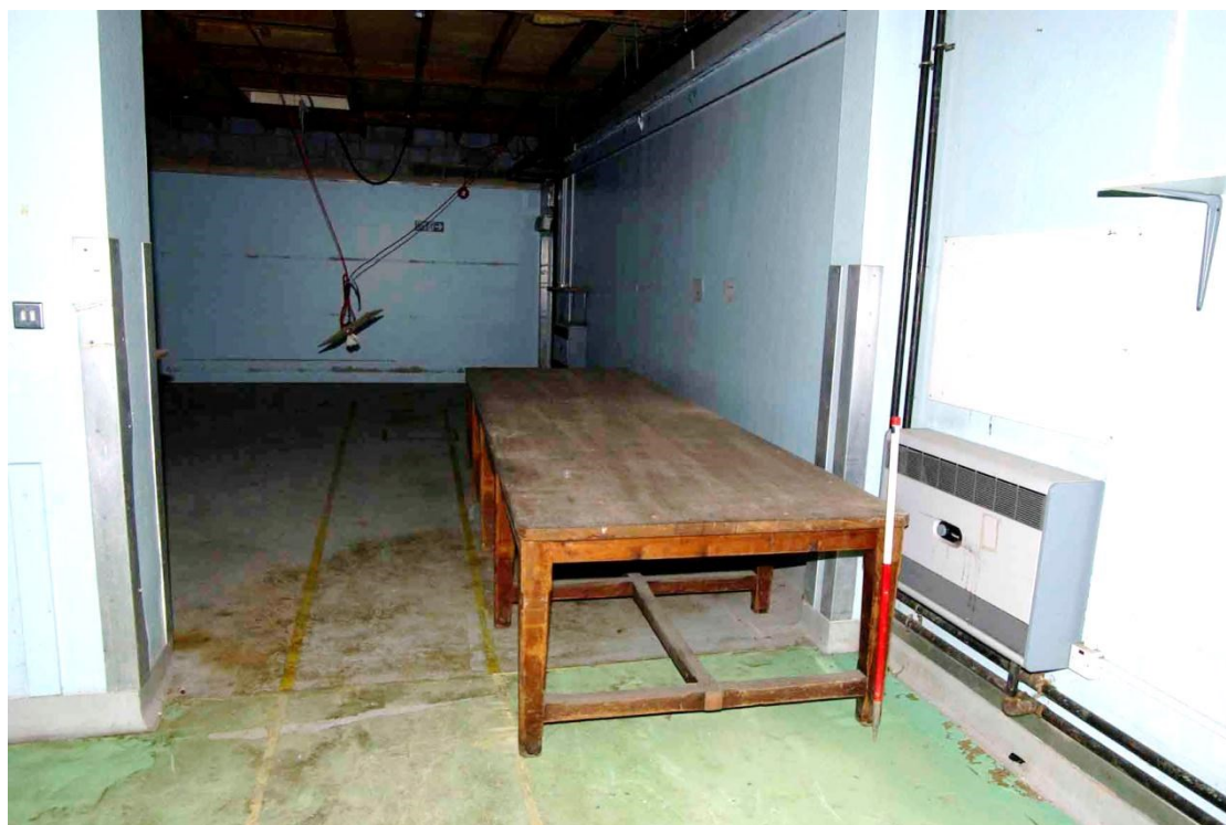
Figure 86 Food preparation room GF18 Looking south-west, 1m scale
