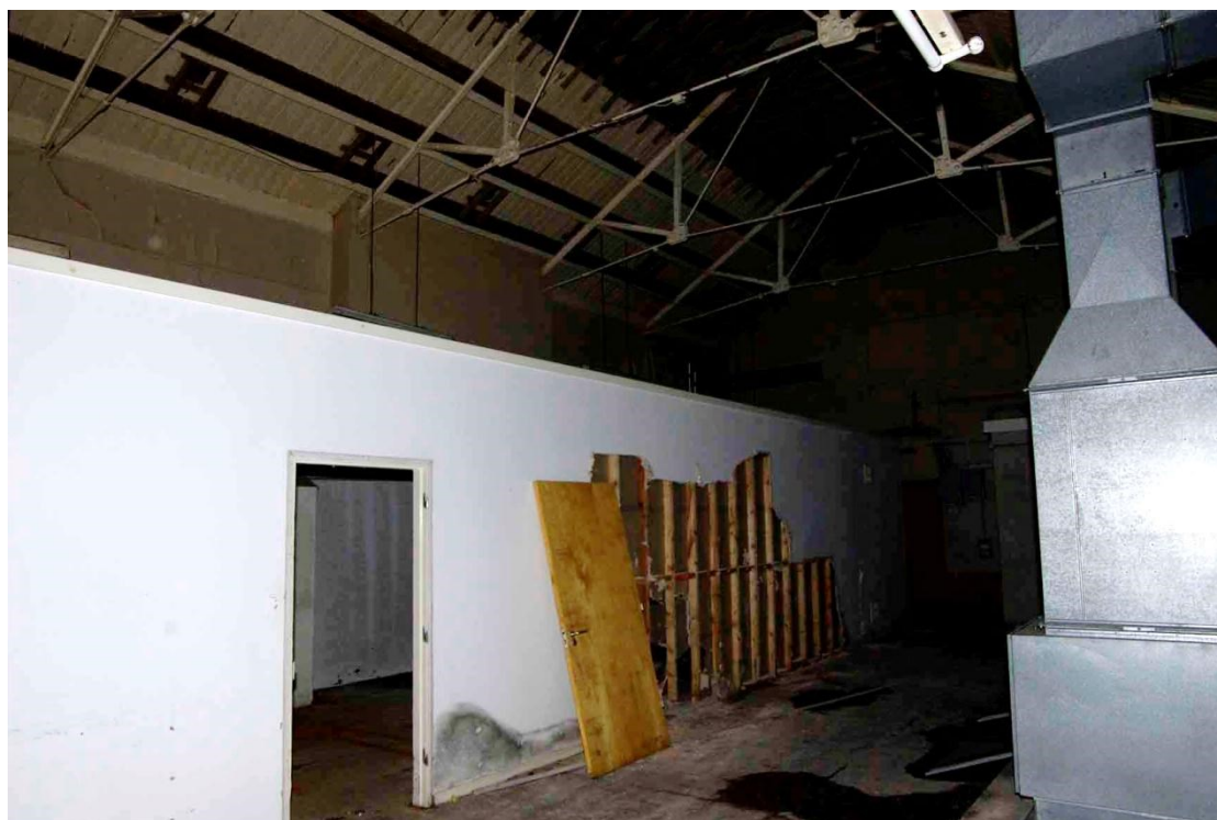
Figure 84 Large food preparation hall Looking west.
