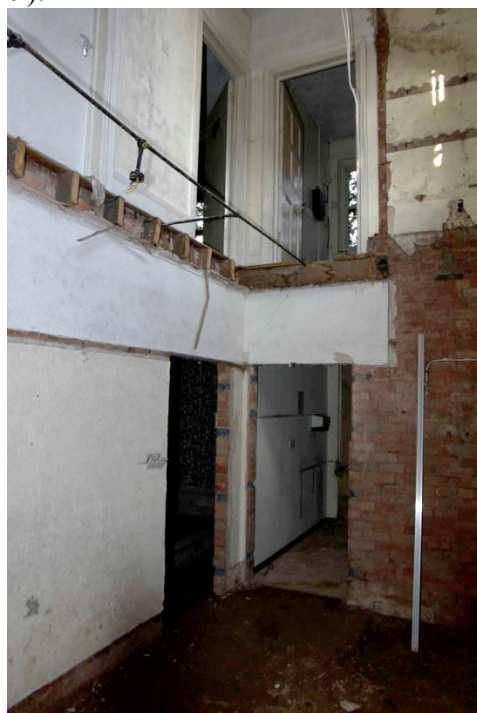
Figure 53 Room GF19 Looking north-west
