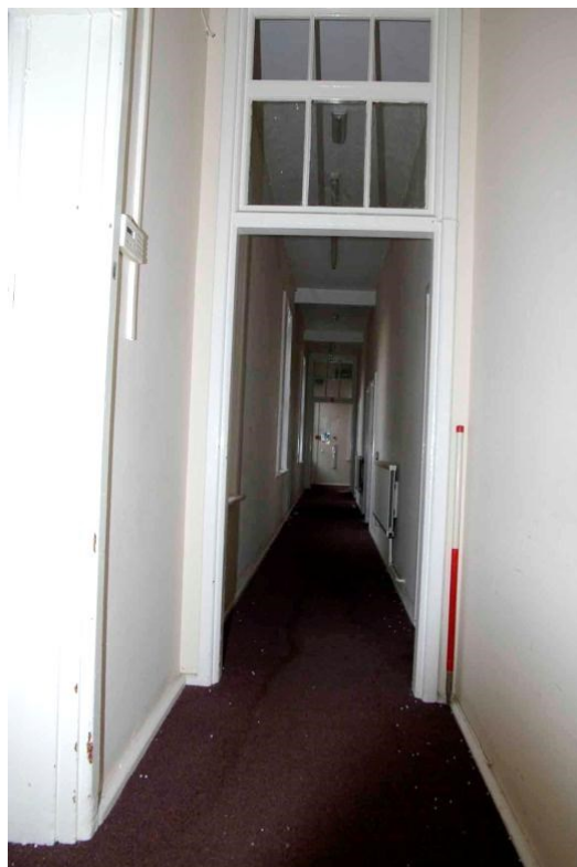
Figure 115 First floor corridor linking attendant's rooms Looking south over main corridor, 1m scale
