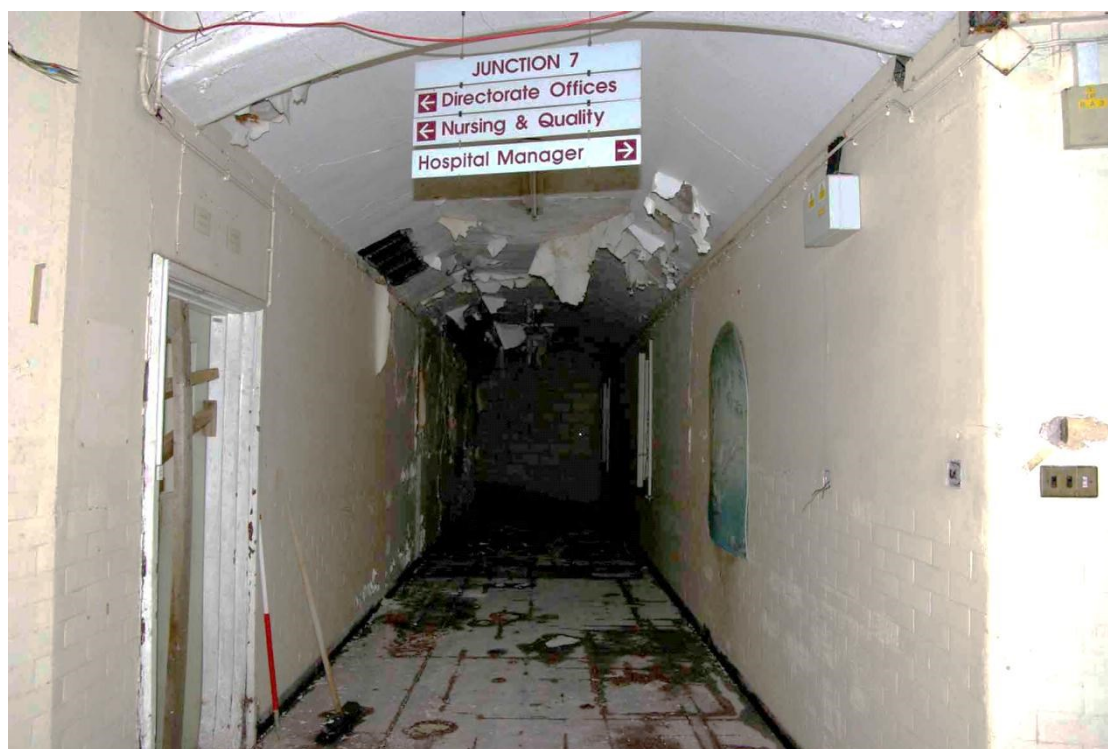
Figure 22 Main corridor at Junction 7
