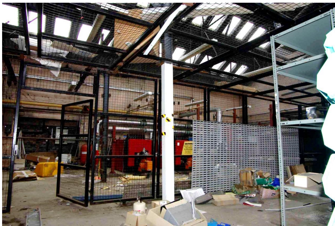
Figure 70 Boiler house interior Looking south-east
