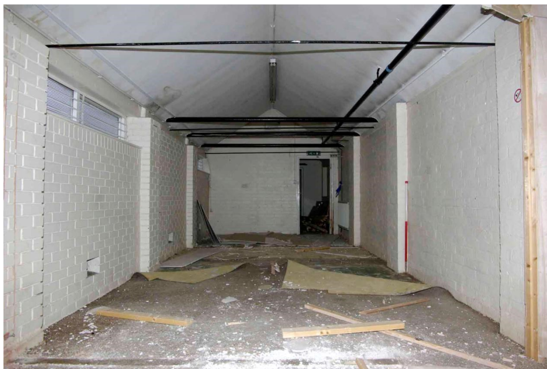
Figure 67 Workshop WS5 Looking north, 1m scale
