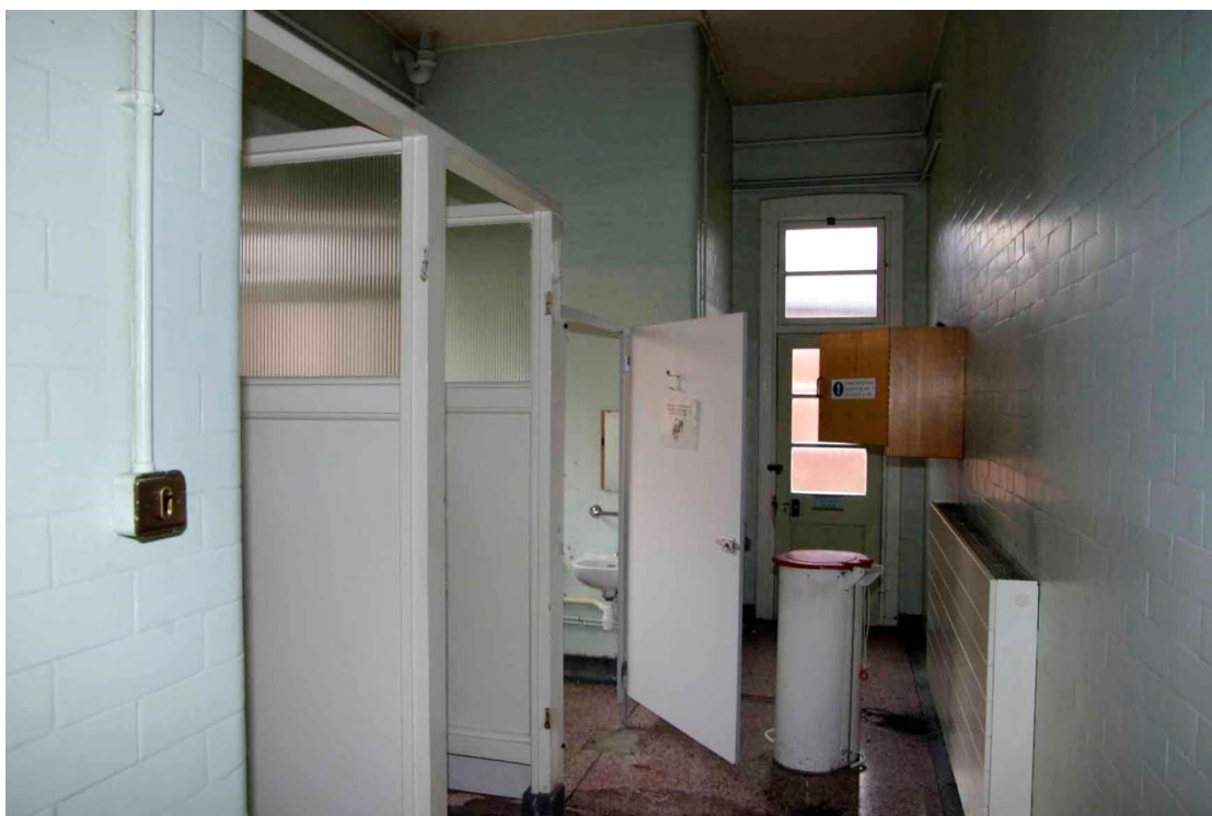
Figure 109 Toilet block on north side of Grace Dieu ward Looking north
