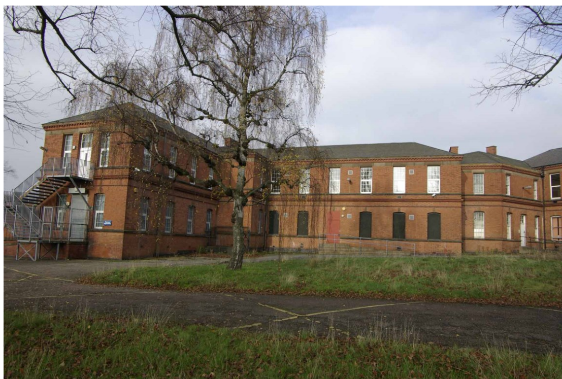
Figure 91 Daisy Peake Building – Beaumanor and Cropston wards Looking north-west
