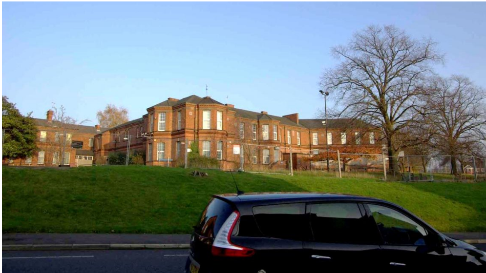
Figure 3 Daisy Peake Building Seen from Heronbridge Road. Looking north east
