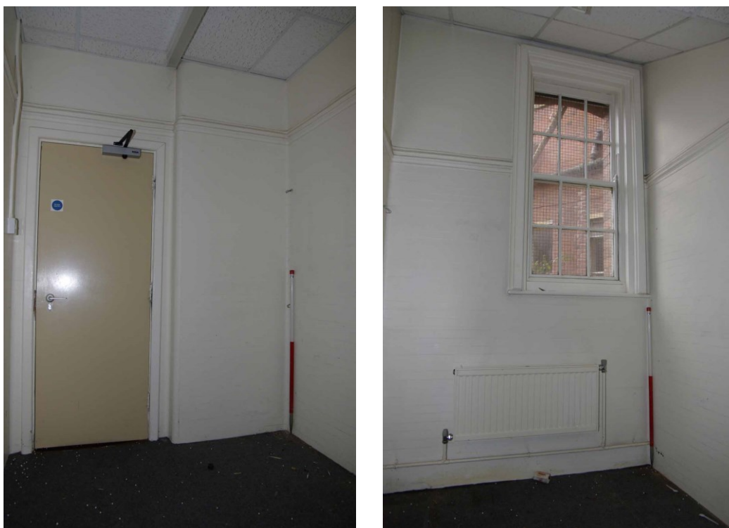
Figure 106 Cell in Fosse ward Looking south-west (left photo) and north-east (right), 1m scale. Note painted glazed tiles
