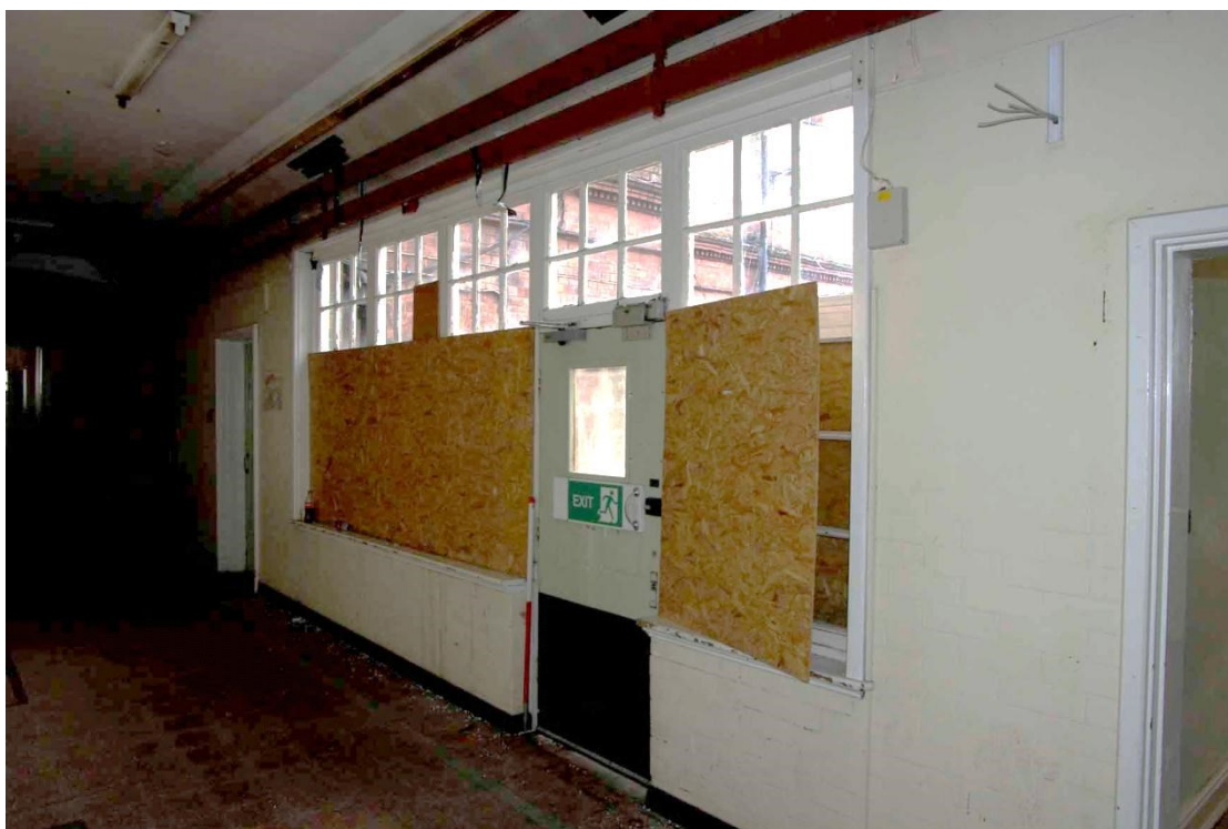
Figure 46 Main entrance to main corridor Looking south-east, 1m scale
