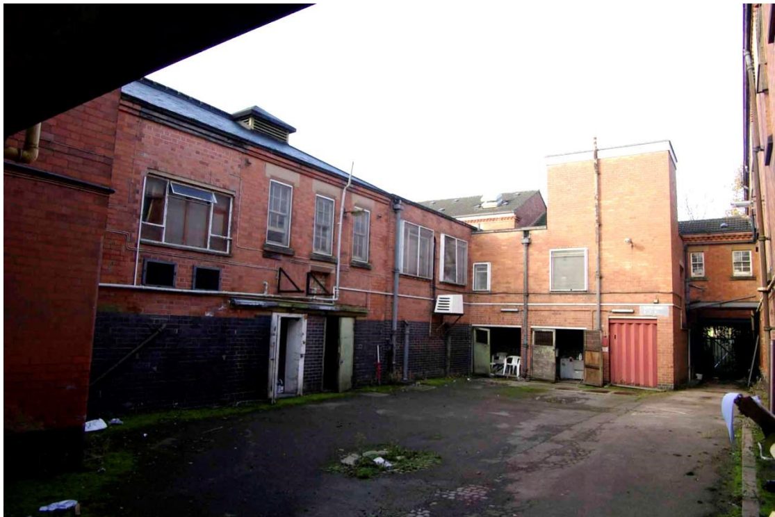
Figure 83 North facing elevation of food preparation area Looking south west, 1m scale. Modified Crittall window on left, Joint in building to right of ranging pole, inserted lift shaft over red doors and western corridor heading towards George Hine House on right of photo. Note basement store rooms
