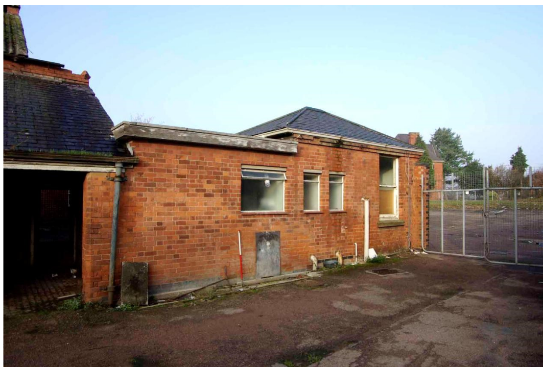
Figure 71 Boiler house washroom Looking north-west, 1m scale
