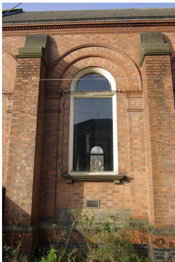
Figure 119 Side window detail of hall
