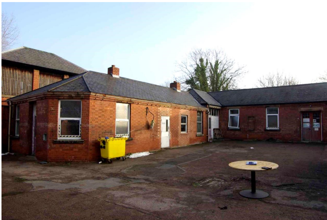
Figure 54 Workshop WS2 and 3 Looking north-east. Photo taken facing away from boiler house
