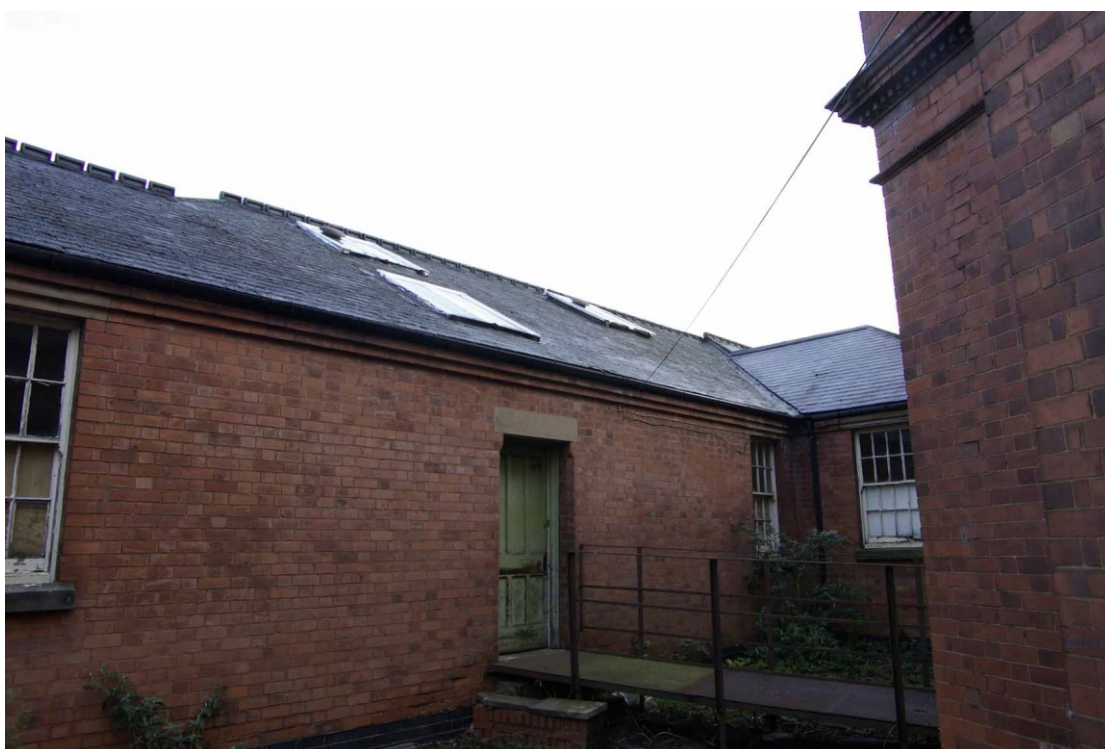
Figure 26 South facing elevation of main corridor at Junction 5 Looking north-east. Note variations in ridge heights
