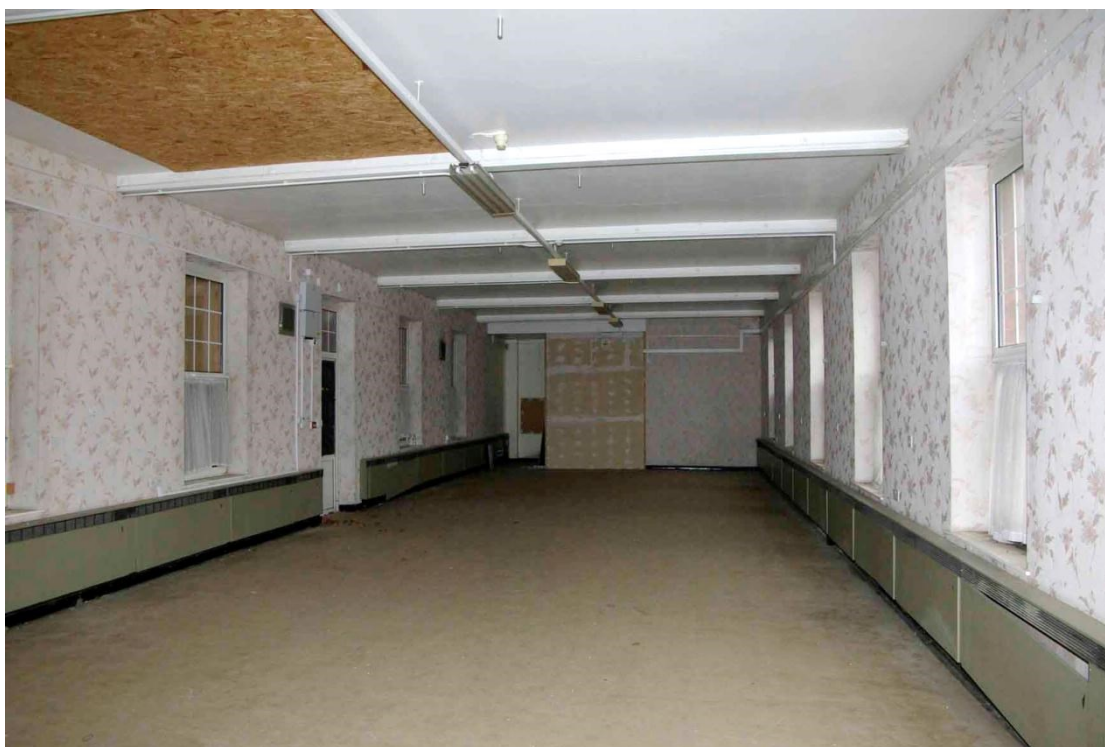
Figure 110 Beaumanor ward (east) Looking south-west, 1m scale. Note blocked end wall
