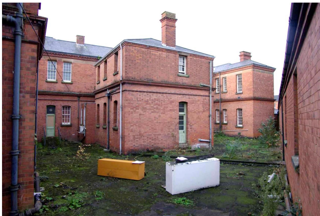
Figure 96 Yard behind Grace Dieu and Fernie wards Looking south-west. Main corridor on right
