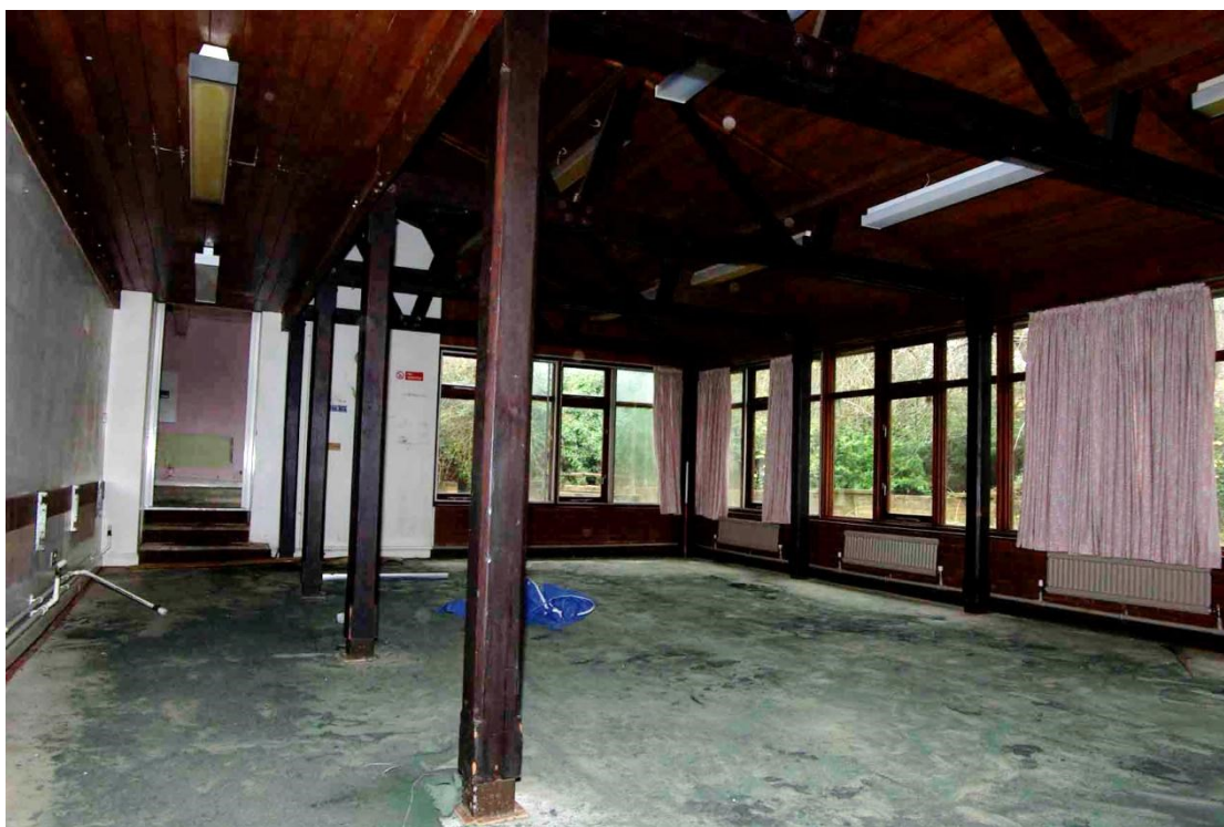
Figure 80 Modern conservatory Looking north-east. Doorway to coffee lounge up steps on left of picture
