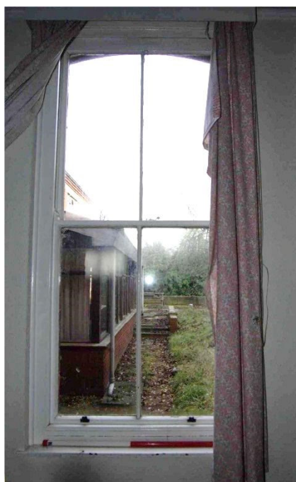
Figure 44 Ward GF 12 north east facing sash window Looking north east, 1m scale. Modern coffee lounge is visible in the courtyard
