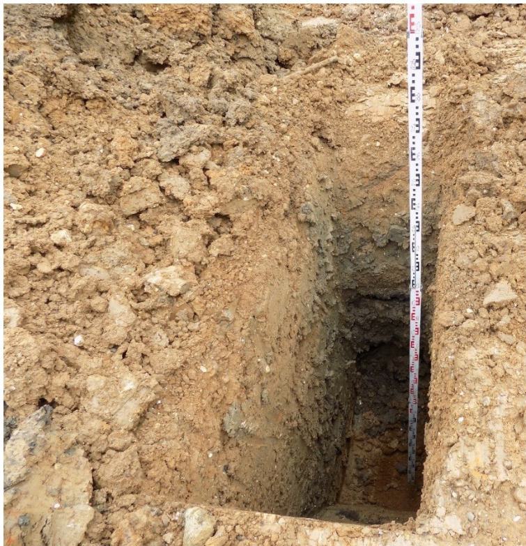
Figure 11: Exploratory trench through the redeposited soil
