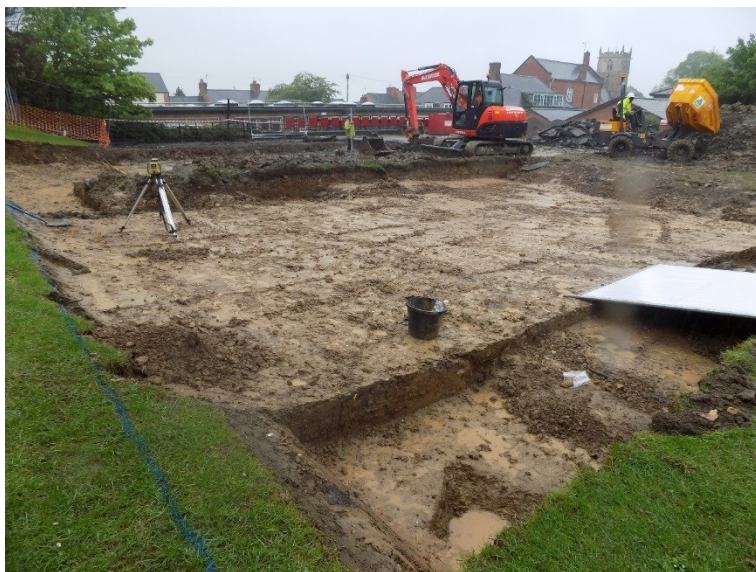
Figure 7: View southwest across the site to towards the end of the strip. Trench 3 in foreground. The human bones were recovered from the area in the foreground where spoil is mounded.
