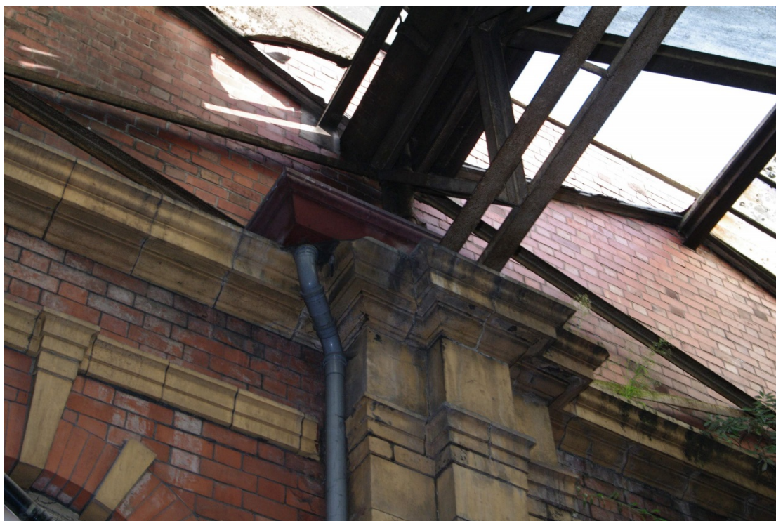
Figure 37 Portico area G1 east wall and roof structure Looking east
