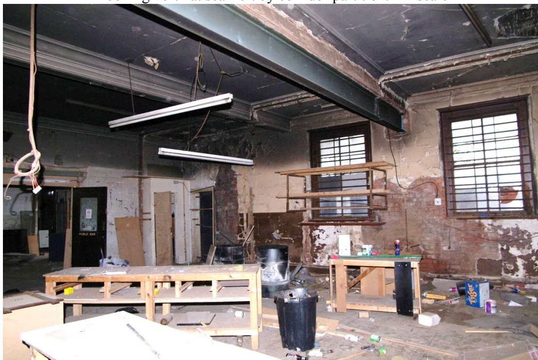
Figure 109 Parcels office Room F2 Looking south-east
