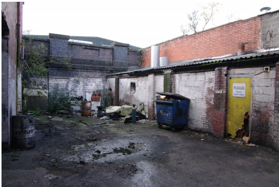
Figure 52 Booking hall yard G2 lean-to structures Looking north-west
