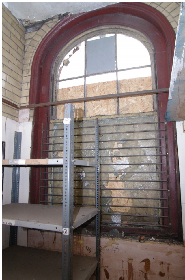
Figure 122 Parcels office Room F6 window detail Looking south-east. Note glazed bricks
