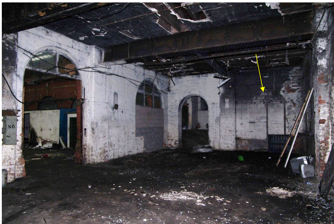
Figure 77 Parcels office ground-floor Room G9 Looking south-east. Arches to portico on left. Arches to Room G8 (including blocked arch arrowed) on right
