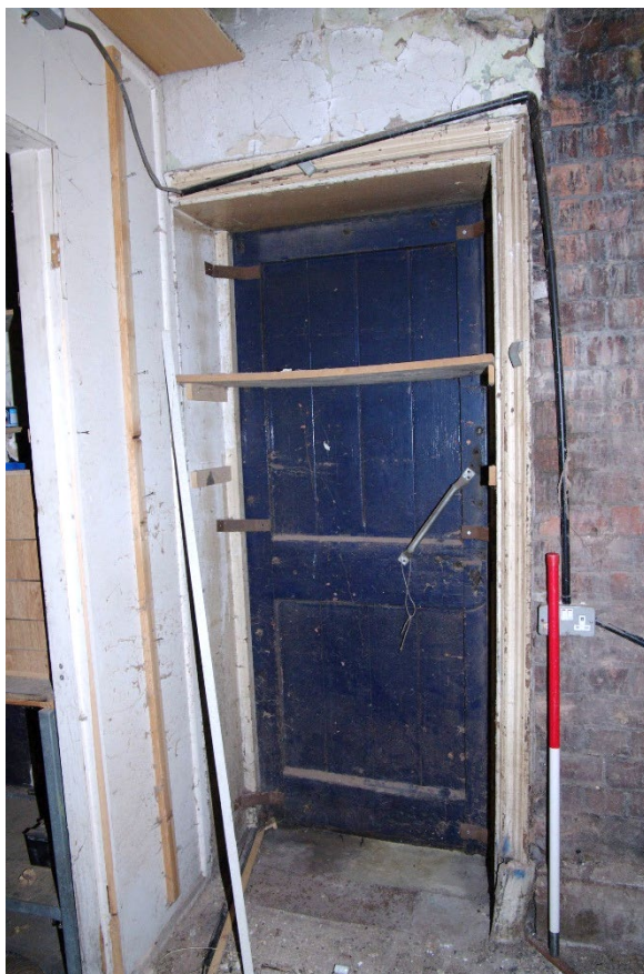
Figure 112 Parcels office Room F2 west wall door Looking south-west. 1m scale
