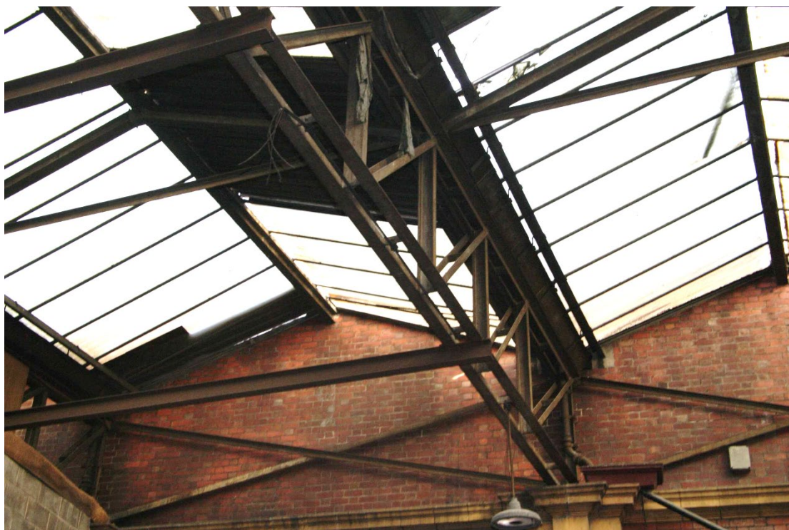
Figure 38 Portico area G1 roof structure Looking west
