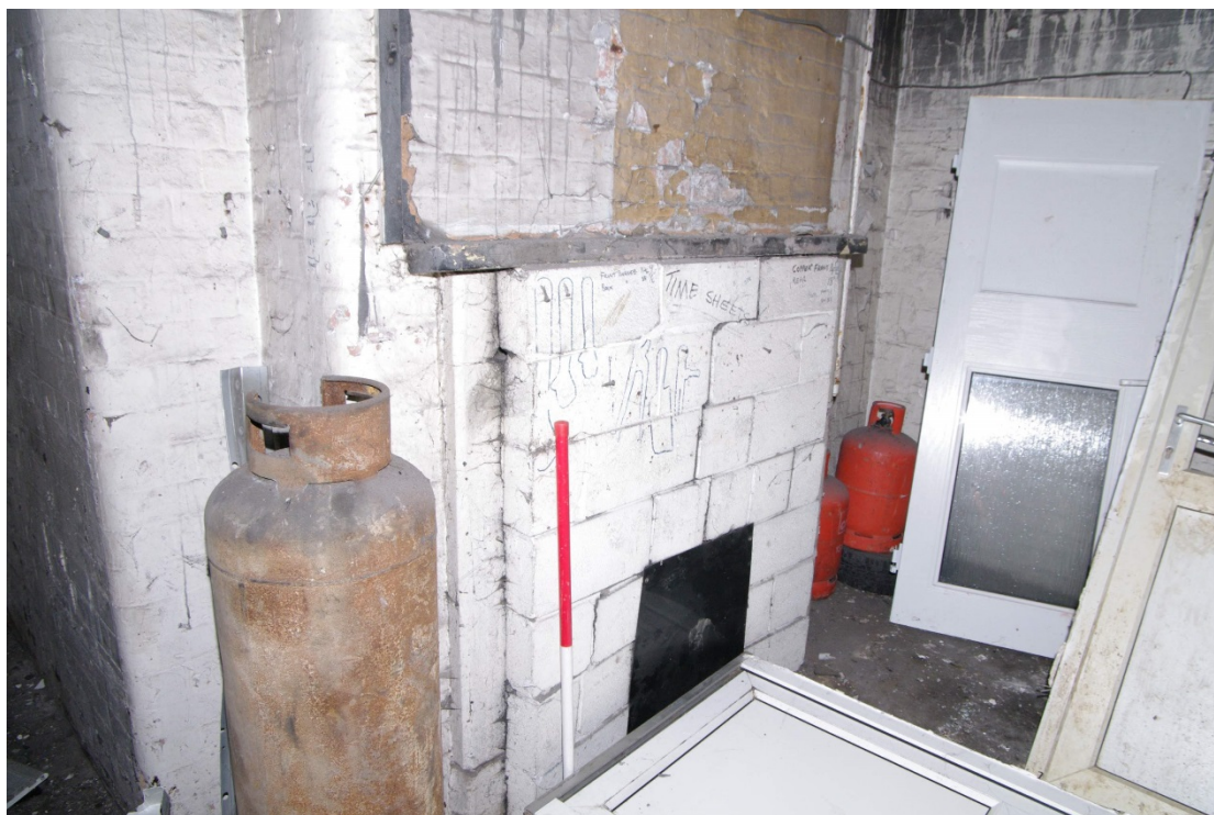
Figure 79 Parcels office Room G9 fireplace Looking north-east. 1m scale
