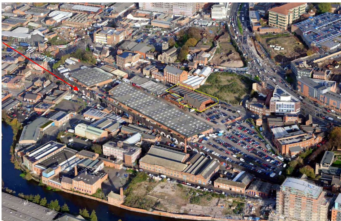
Figure 15 Aerial view of station site early 2010s Looking north-east. Yellow outline shows the portico and parcels office discussed in this report. Red arrow indicates the line of the brick viaduct
