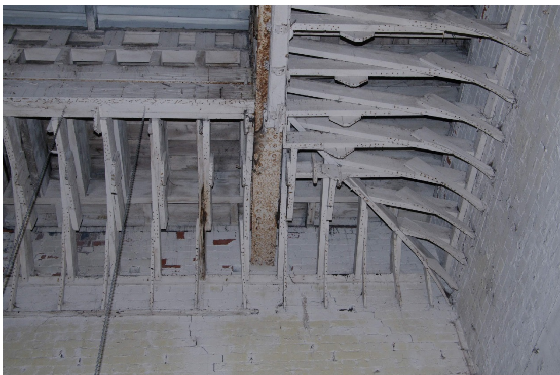
Figure 71 Room G6 ceiling detail North-west corner of room
