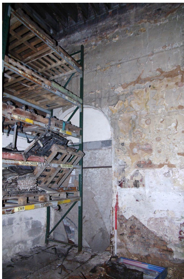
Figure 65 Room G4, blocked archway on south wall Looking south-east. 1m scale
