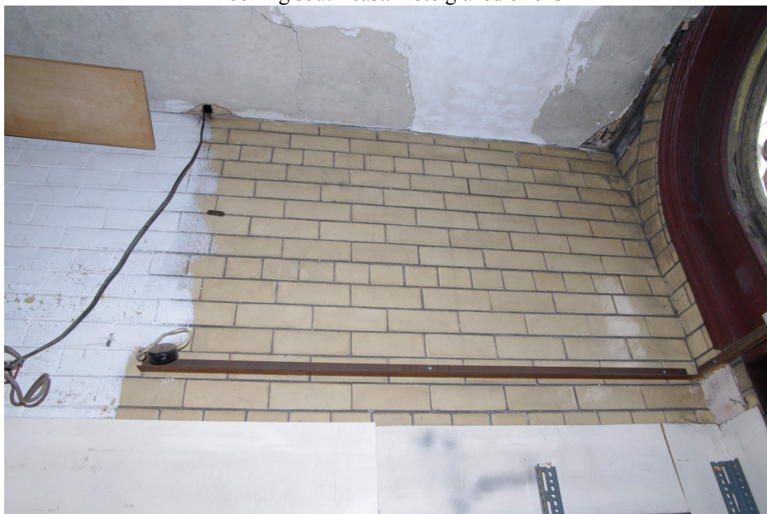
Figure 123 Parcels office Room F6 east wall Looking east
