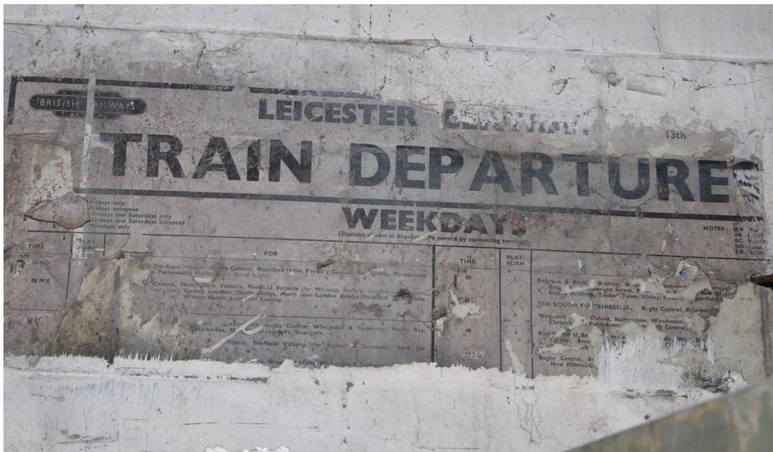
Figure 86 Parcels office Room G10 timetable remnant Looking towards north-east corner.
