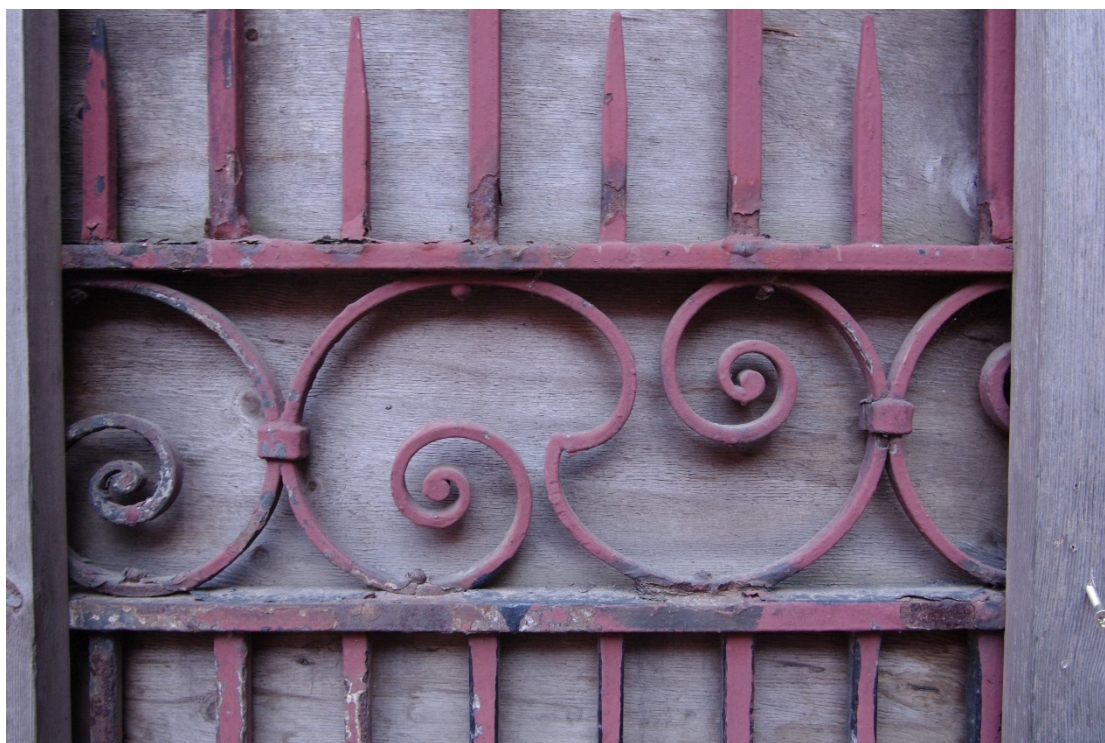
Figure 22 Detail from the parcels office gates Viewed from the inside
