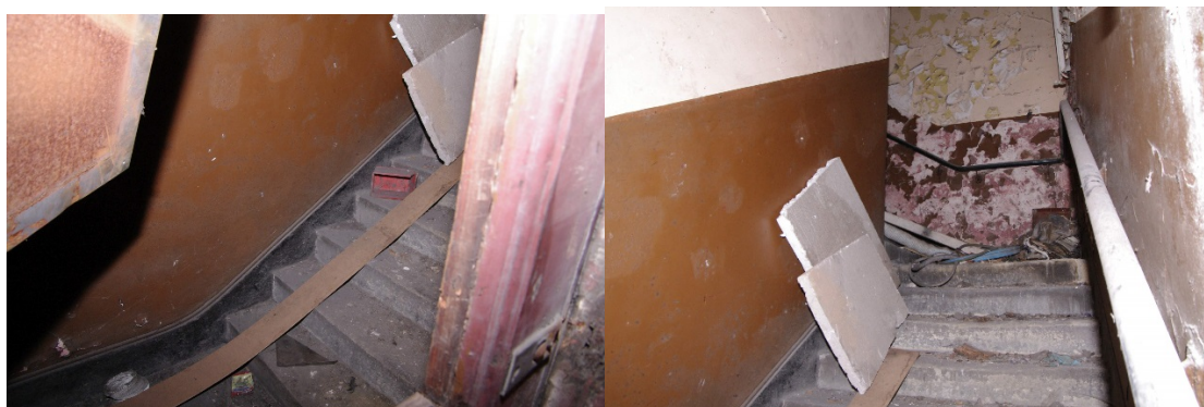
Figure 49 Portico area G7 parcels office stairs Photos taken through doorway window.
