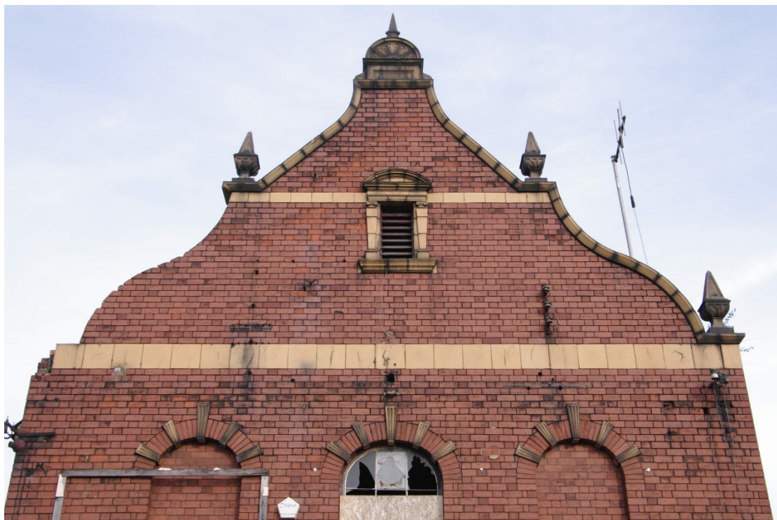
Figure 95 Parcels office south-facing elevation gable detail Looking north
