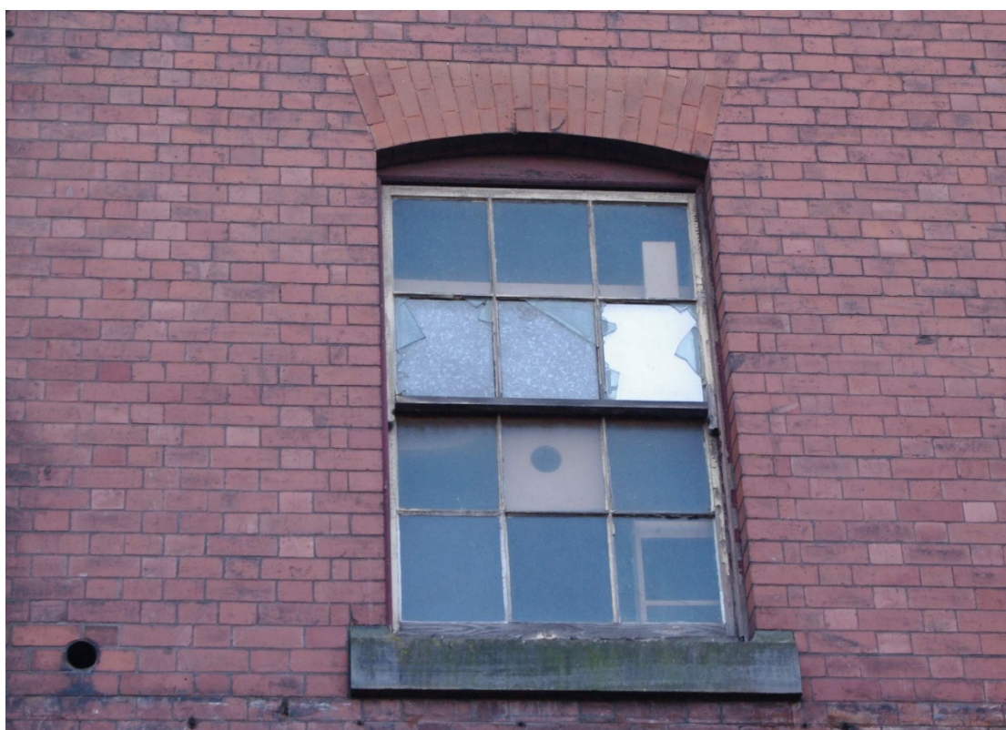
Figure 92 Parcels office east-facing elevation first-floor window Looking west
