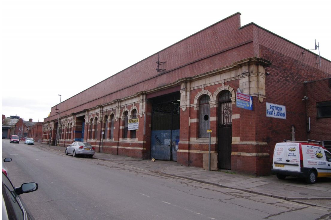
Figure 19 East-facing elevation of portico Looking south-west
