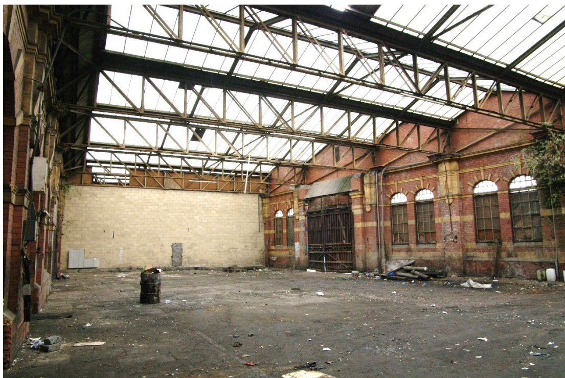
Figure 43 Portico area G7 Looking north-east
