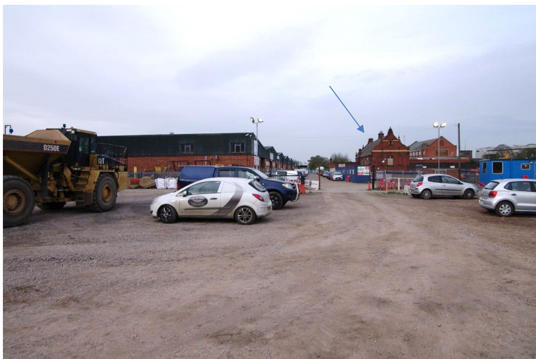
Figure 5 Looking northwards along former track bed Parcels office on right (arrowed)
