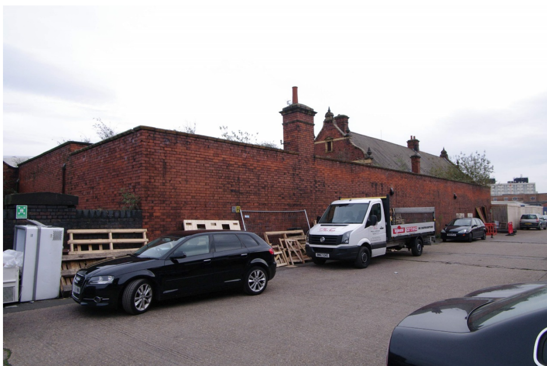
Figure 102 Parcels office north-facing gable Looking south-east over parapet around the external yard and booking hall area. The chimney in the foreground serves the fireplace in G3 ticket office
