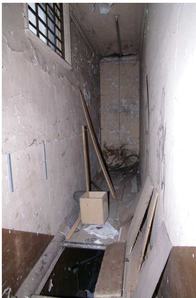
Figure 104 Parcels office Room F1 Looking east across inserted floor over stairs
