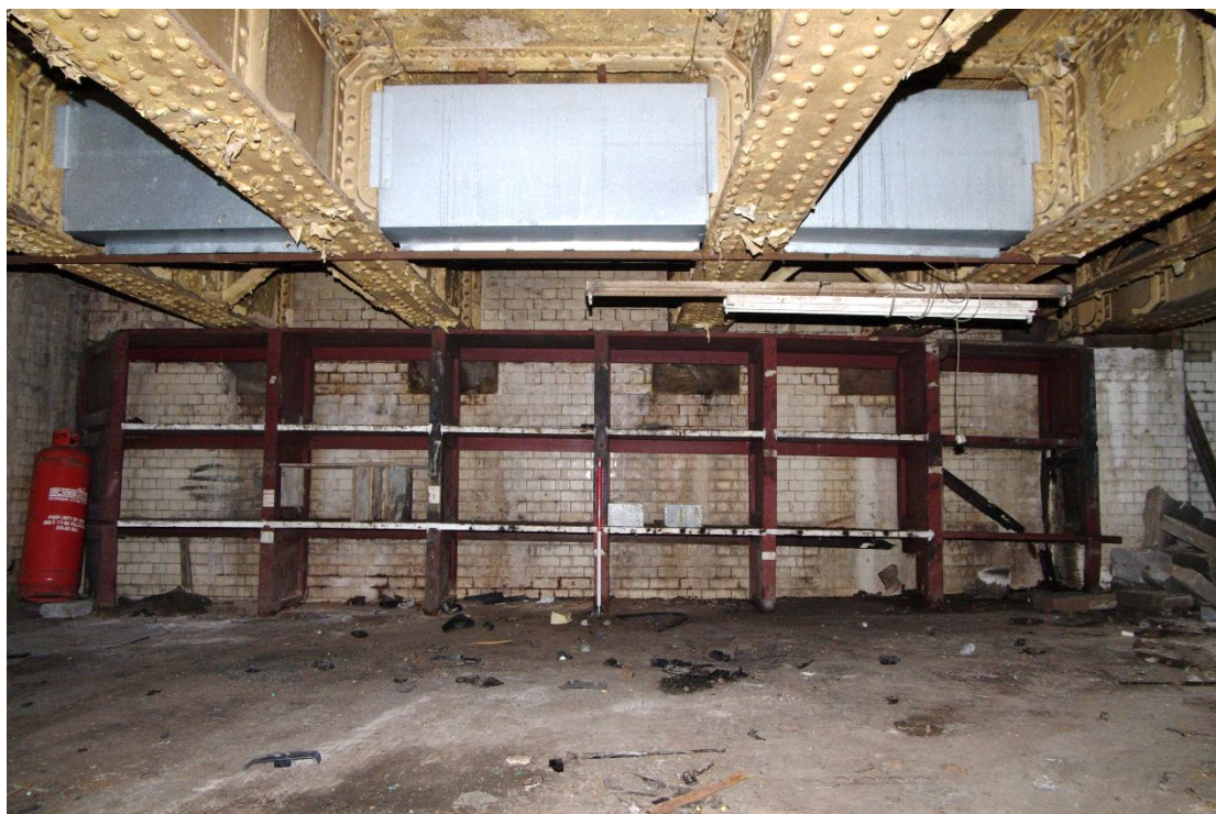
Figure 89 Parcels office Room G11 left luggage rack Looking north. 1m scale
