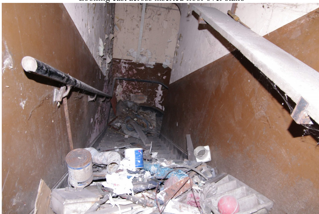
Figure 105 Parcels office Room F1 stairs Looking east (see also Figure 49)
