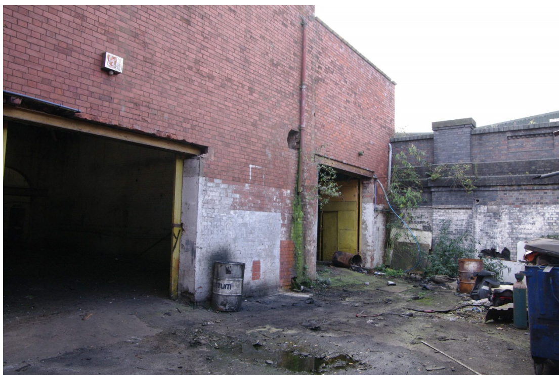
Figure 53 Booking hall yard G2 Looking south-west. Viaduct for platform on right
