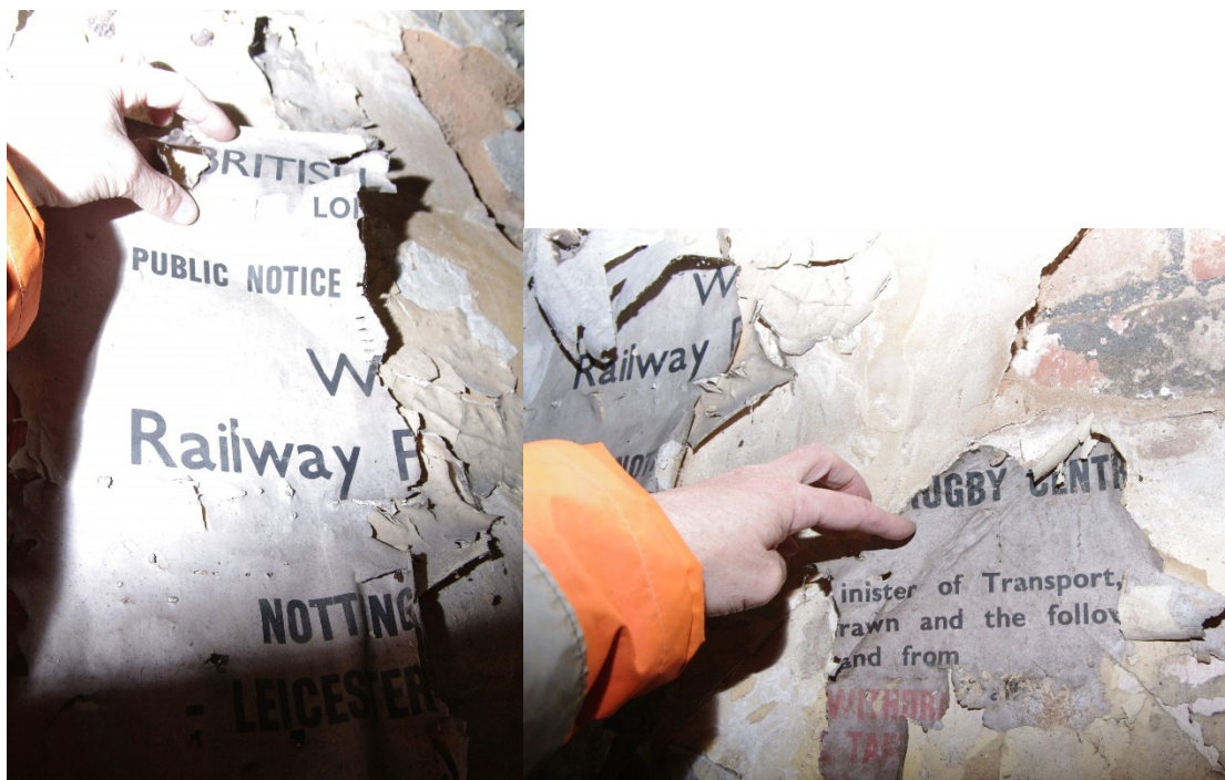
Figure 64 Room G4, remnants of 1969 closure poster On south wall
