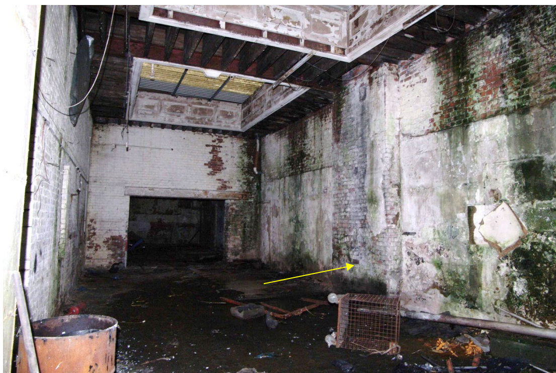
Figure 55 Room G3, ticket office Looking south-west. Blocked fireplace arrowed
