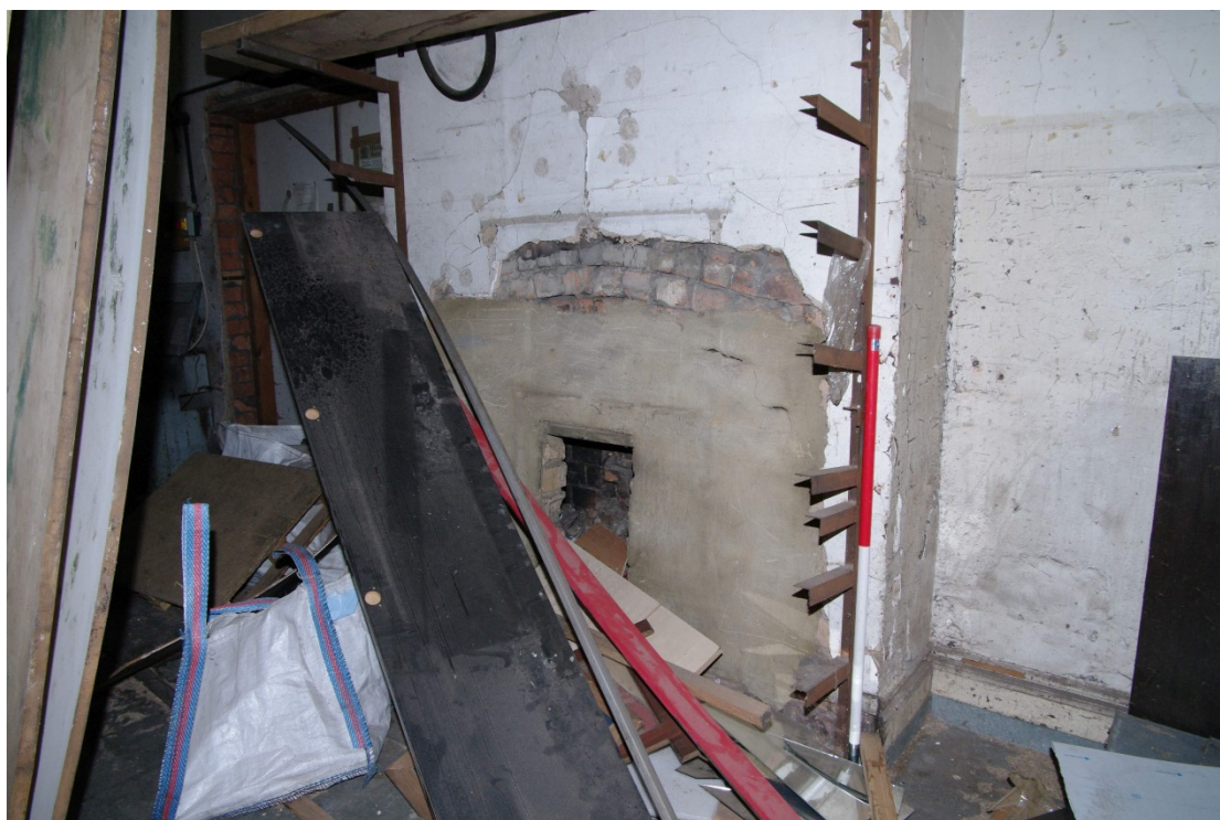
Figure 115 Parcels office Room F3 fireplace Looking south-east. 1m scale
