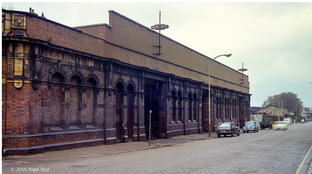
Figure 29 East-facing elevation in October 1974 Looking north-west. Note 'British Railways' signs on brackets. Photo courtesy of Nigel Tout
