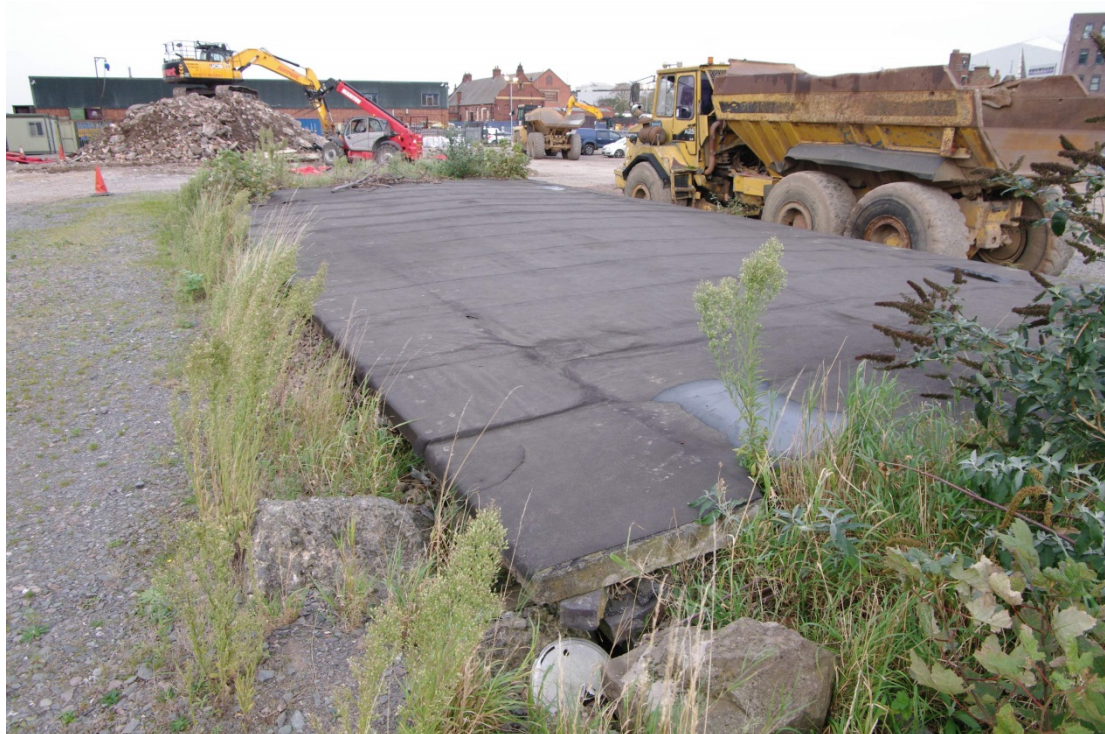
Figure 10 Platform and former roof over tessellated pavement Looking north-east. Parcels office centre background
