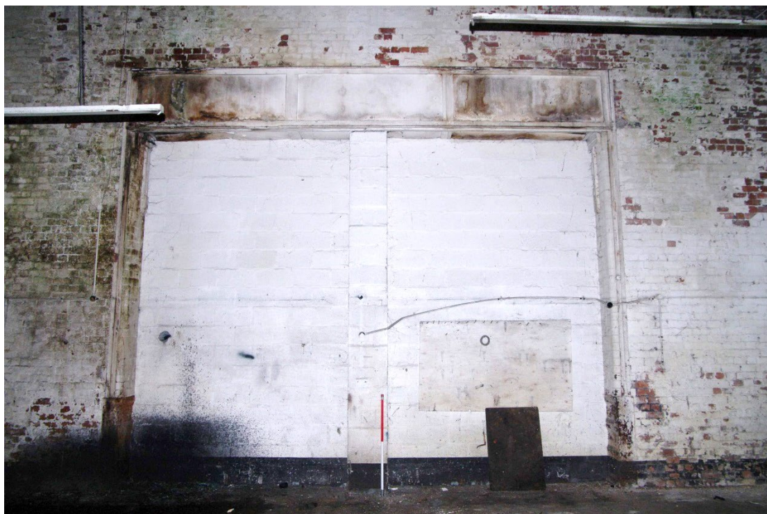
Figure 67 Room G5, blocked entrance from the portico Looking east. 1m scale
