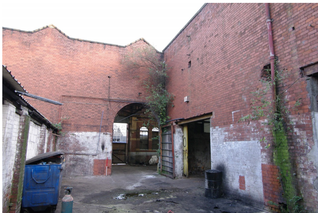
Figure 51 Booking hall yard G2 Looking east towards portico archway. 1m scale
