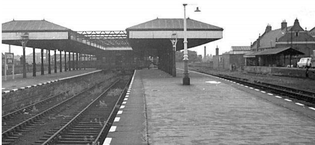
Figure 98 Platforms and parcels office in 1967 Looking north with parcels office on right. Note the covered platform against the parcels office. Photo: courtesy of Nigel Tout
