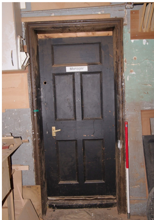
Figure 120 Parcels office Room F4 door detail Looking south. 1m scale
