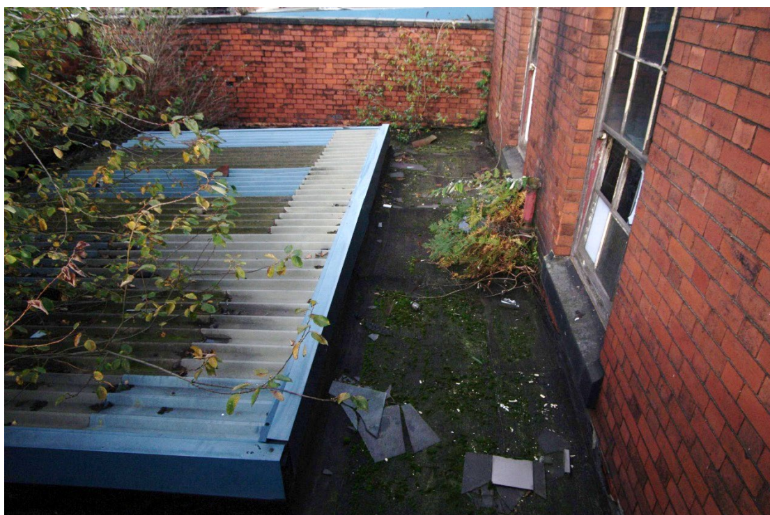
Figure 101 Parcels office west-facing elevation above skylight G10 Looking north
