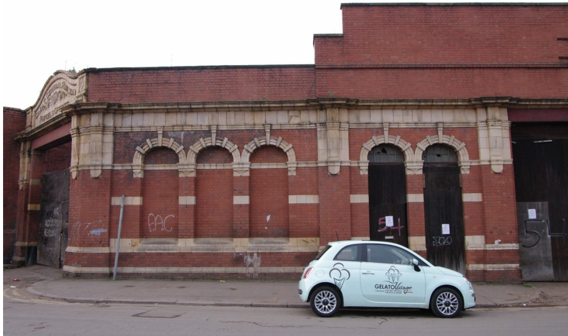
Figure 23 East-facing elevation of portico, blind and open arch detail Looking west. The 4th and 5th arches are for pedestrian access. Note modern parapet
