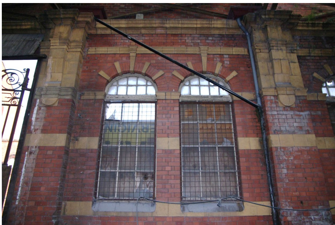
Figure 36 Portico area G1 east wall window detail Looking east
