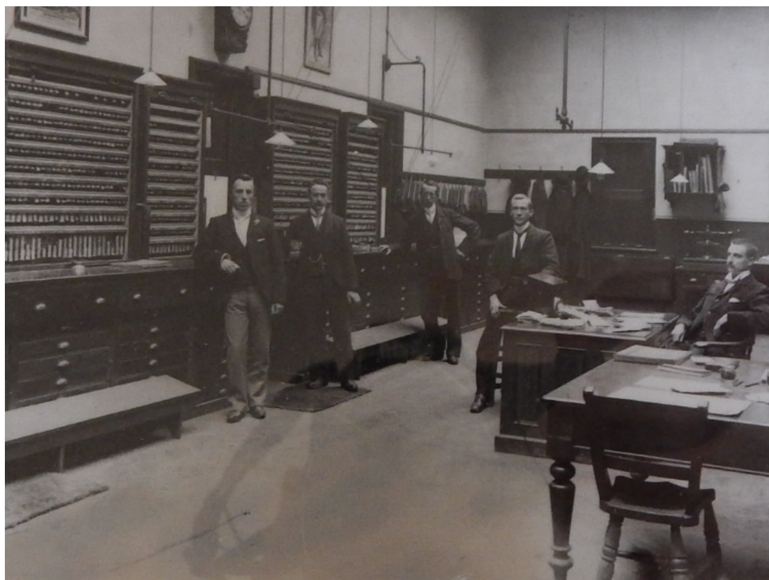
Figure 57 Room G3, ticket office in use Taken from same position as Figure 56. ROLLR Newton collection
