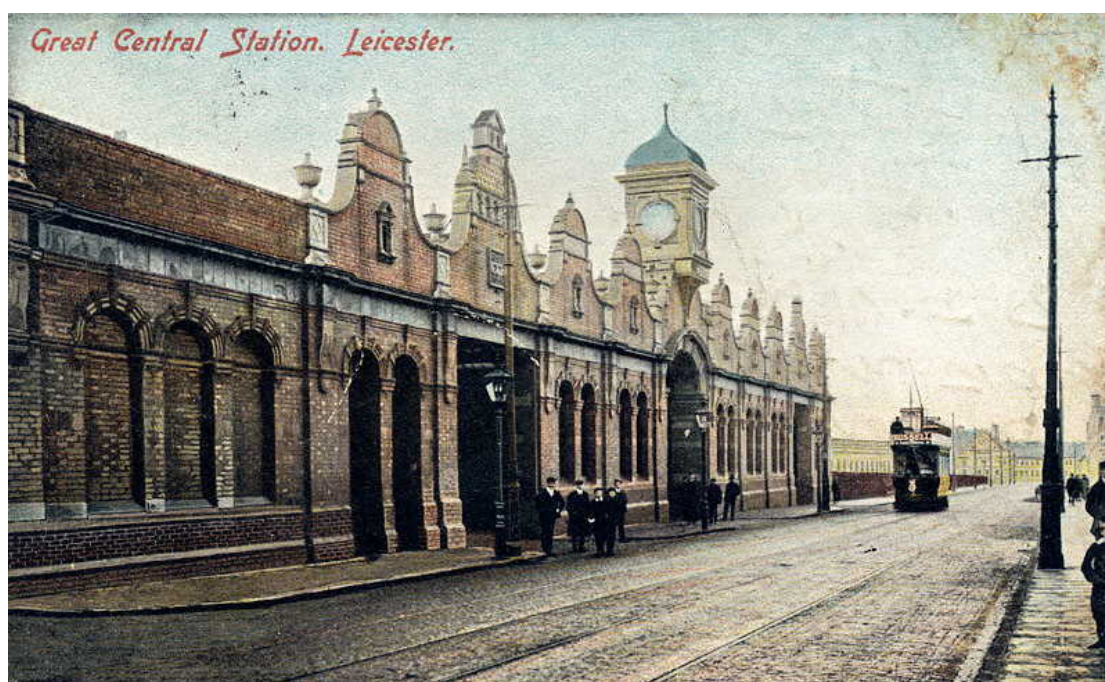
Figure 28 East-facing elevation in 1910 Looking north-west. Photo courtesy of Nigel Tout
