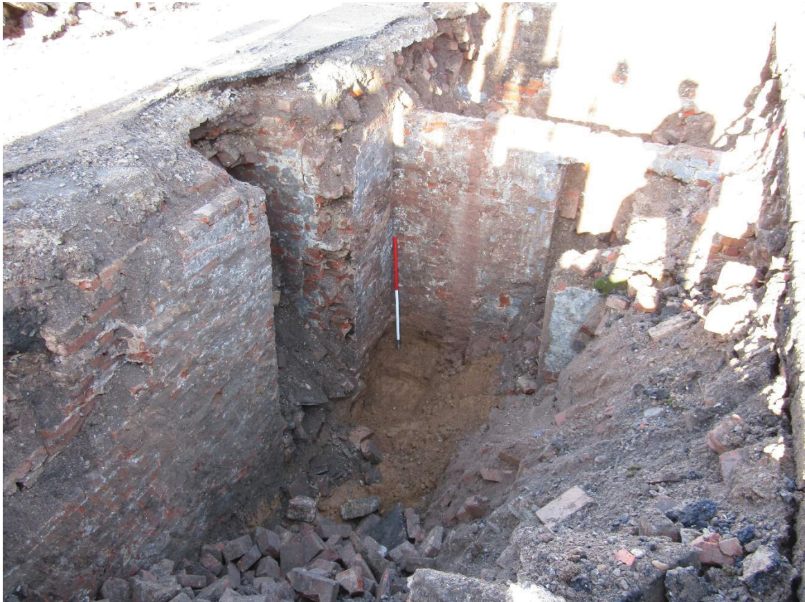
Figure 8: View of brick cellar at no.142 Highcross Street, looking NW, 1m scale.
