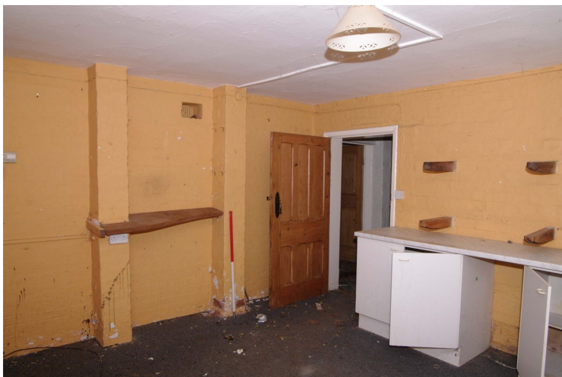
Figure 49 Room 6 Looking north-west. 1m scale
