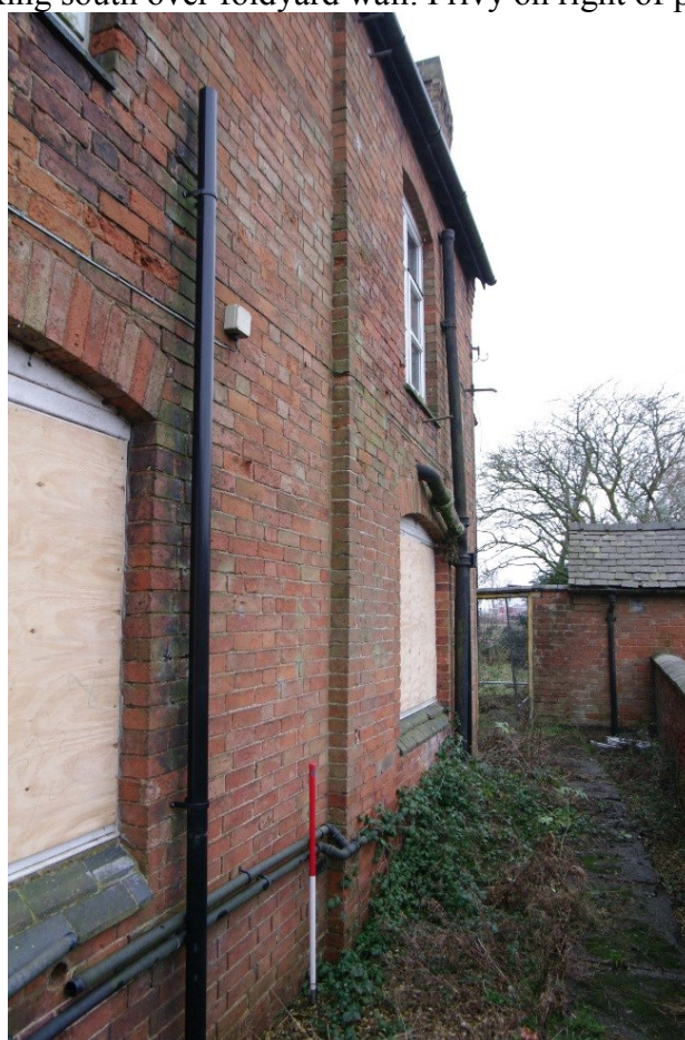
Figure 27 North facing elevation and foldyard wall Looking south-west. 1m scale. Note step in wall just beyond the scale
