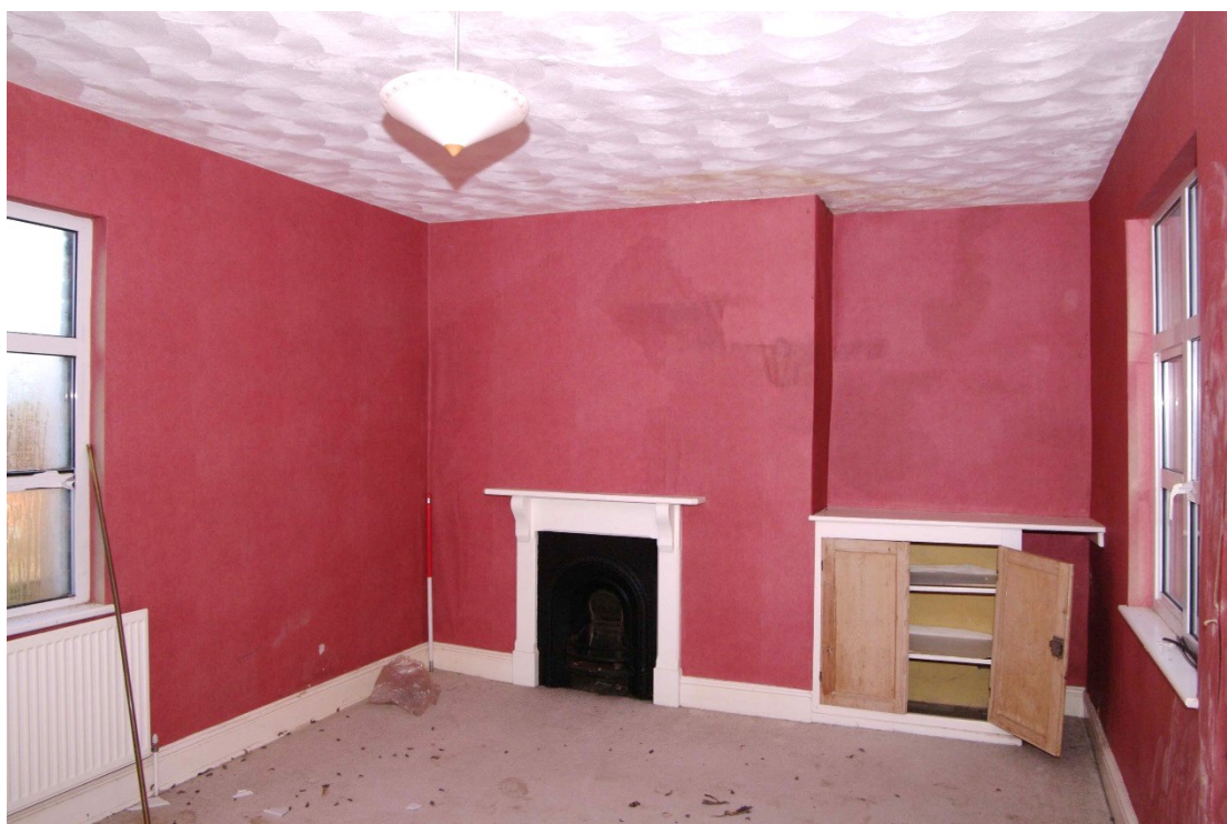
Figure 78 Room 15 Looking north-east. 1m scale
