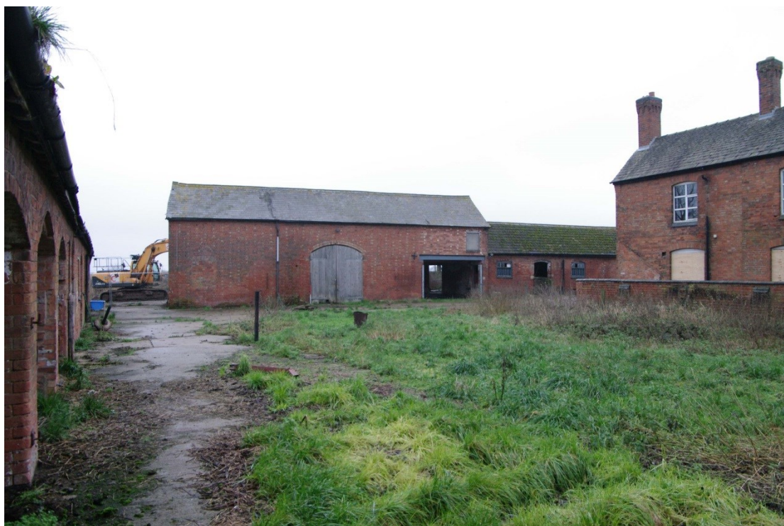
Figure 82 North to south barn, west facing elevation across foldyard Looking east. East to west barn on left
