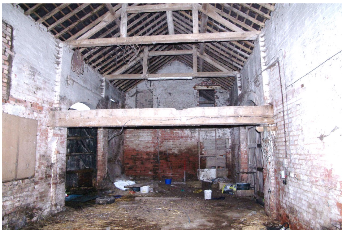
Figure 94 North to south barn. Room 1 Looking south. 1m scale
