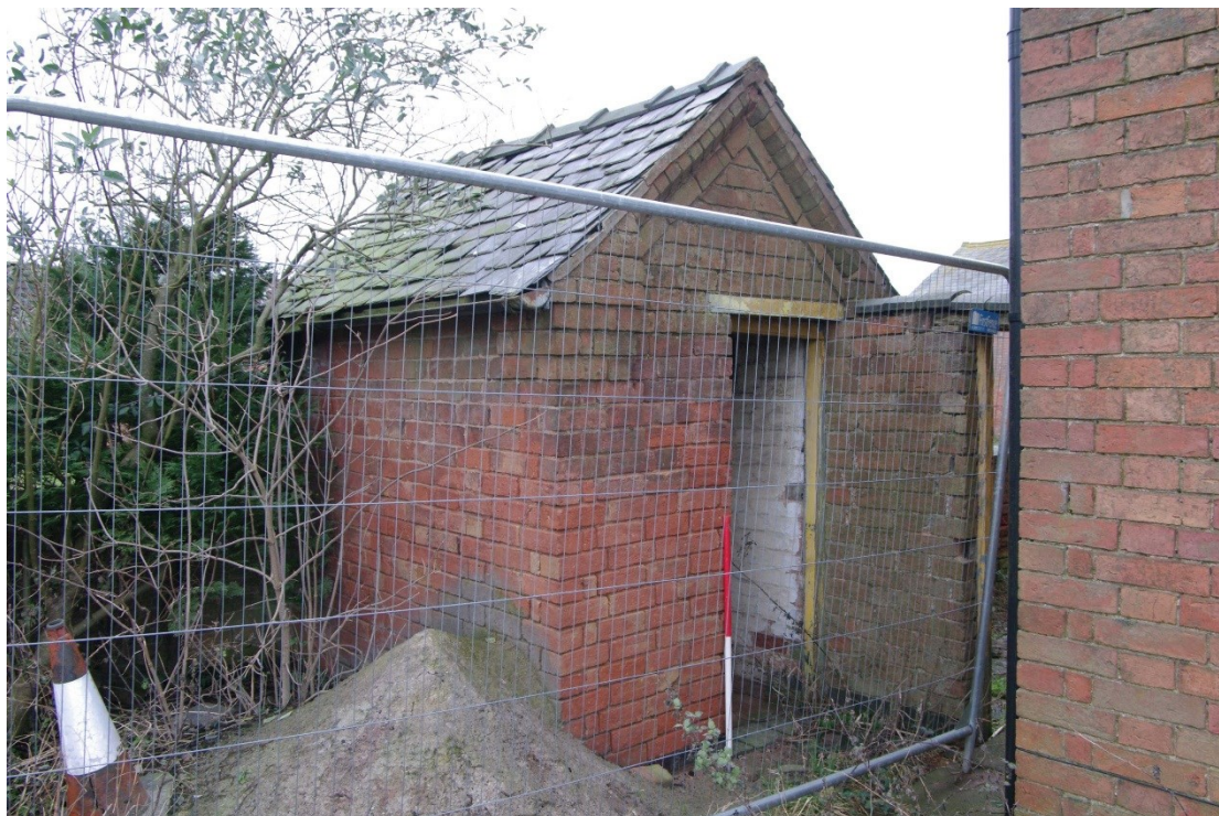
Figure 30 Privy at north-west corner of the house Looking north-east. 1m scale
