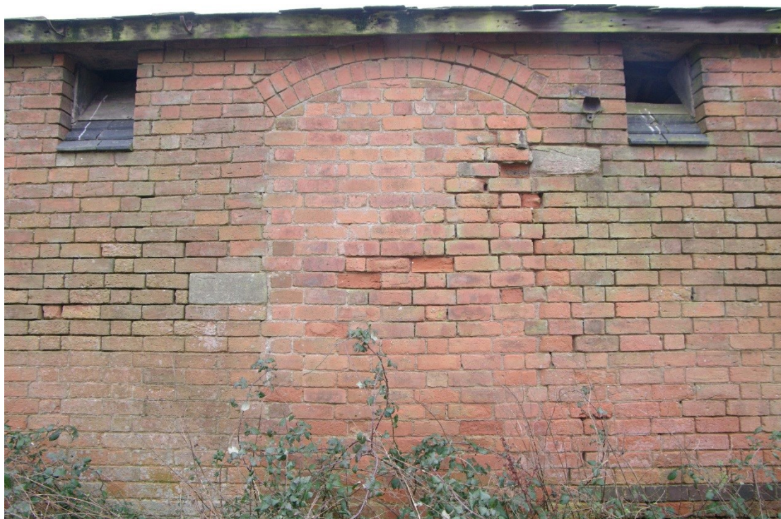
Figure 112 East to west barn, north facing elevation, vents and blocked doorway Looking south
