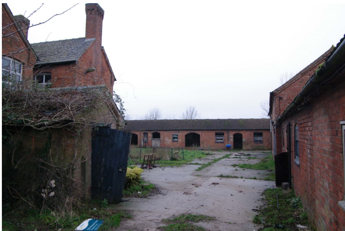
Figure 4 Old Warren Farm general view Looking north across foldyard. House on left
