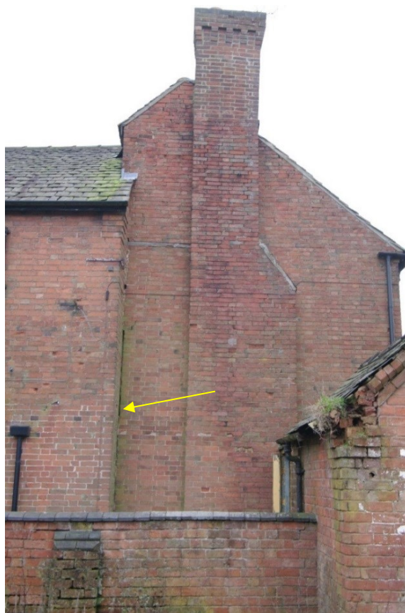
Figure 28 North facing gable of main farmhouse Looking south. Foldyard wall in foreground. Privy on right. Arrow points to butt joint of farmhouse and rear range
