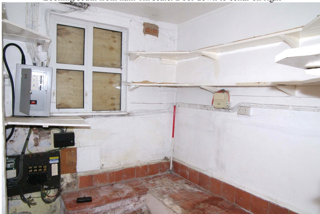
Figure 44 Room 4 Looking south-west. 1m scale. Note shelves and wooden supports
