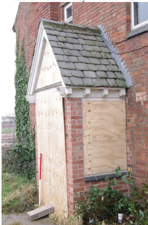
Figure 17 South facing elevation, porch detail Looking north-west. 1m scale
