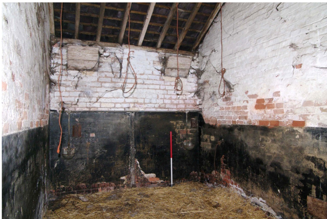
Figure 118 East to west barn. Room 3 Looking north. 1m scale
