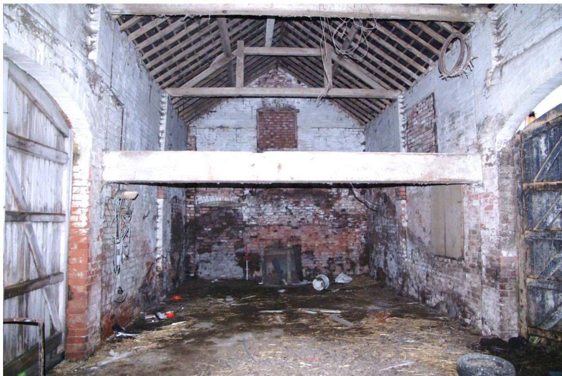
Figure 93 North to south barn. Room 1 Looking north. 1m scale
