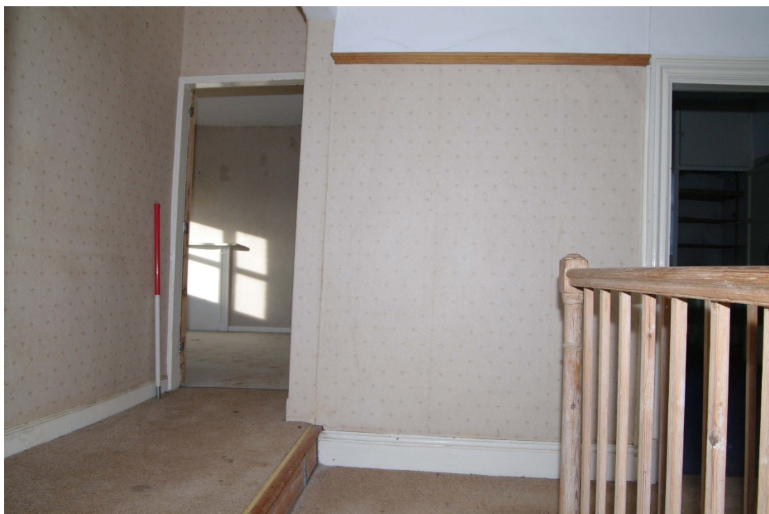
Figure 67 Room 12/landing Looking north-west. 1m scale. Note step in floor level, also note difference in door frame moulding detail
