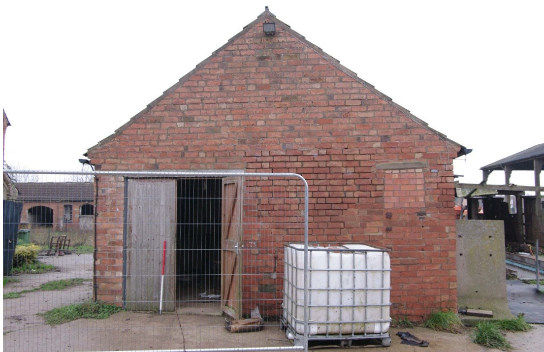
Figure 86 North to south barn. South facing elevation Looking north. 1m scale
