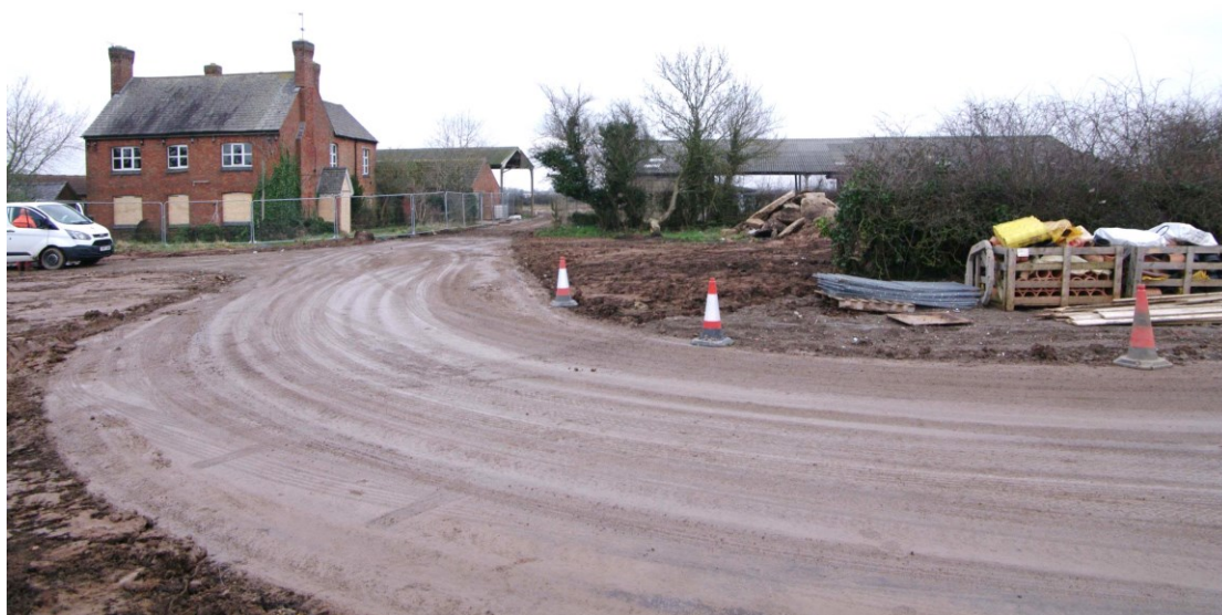
Figure 2 Old Warren Farm Looking north-east along freshly installed access road
