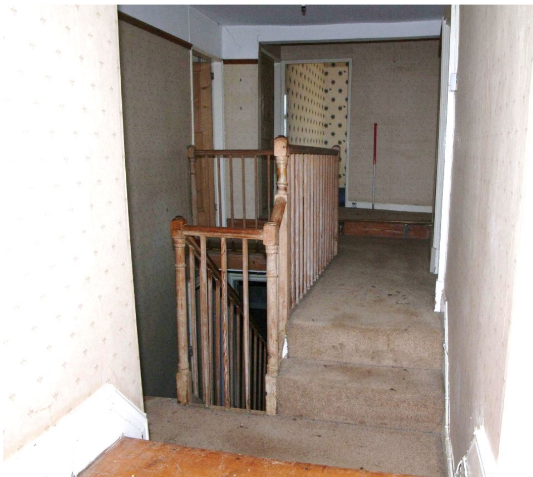
Figure 70 Room 12/landing Looking west. 1m scale
