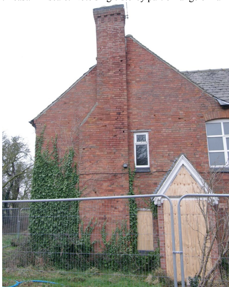
Figure 15 Close-up of south facing gable end Looking north
