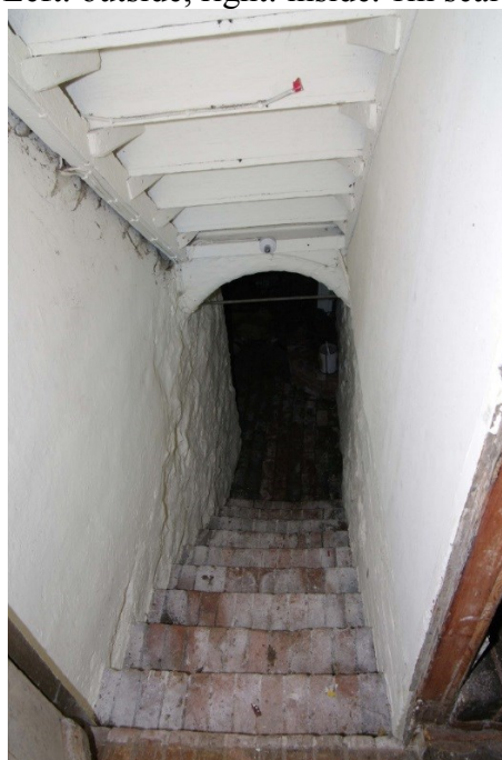
Figure 56 Cellar steps Looking west. Note staircase construction at top of picture
