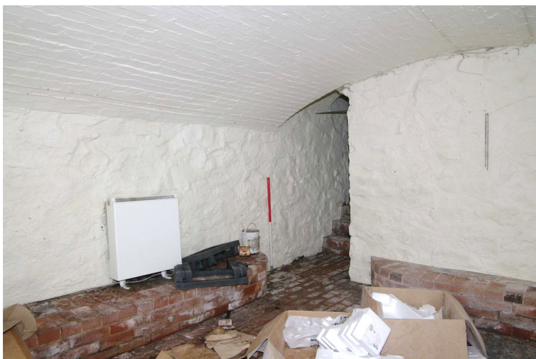
Figure 58 Cellar Looking north-east towards steps. 1m scale
