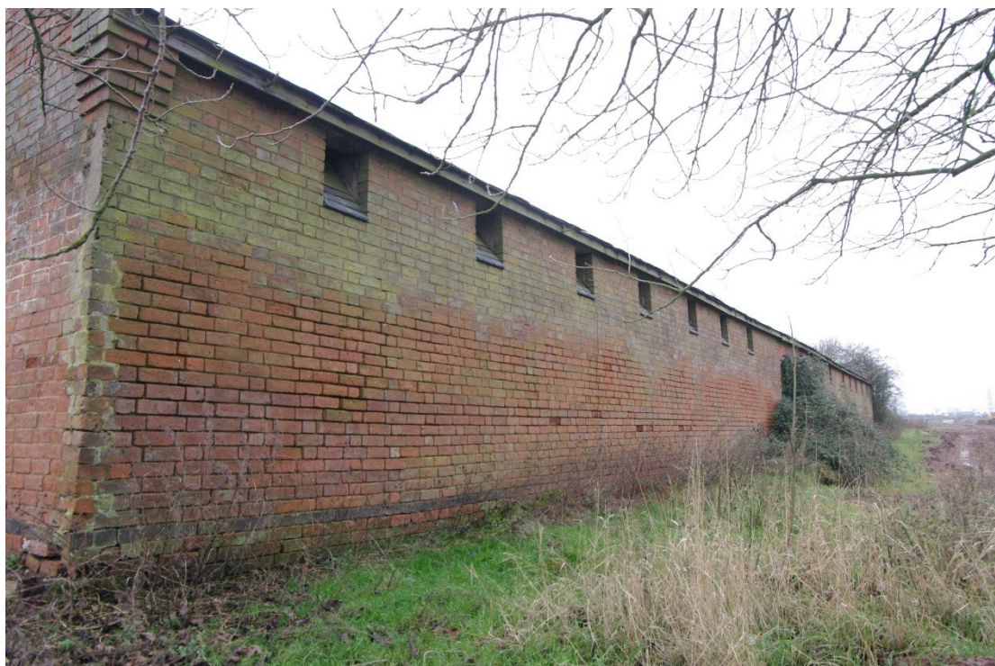
Figure 110 East to west barn, north facing elevation. Eastern end Looking south-west
