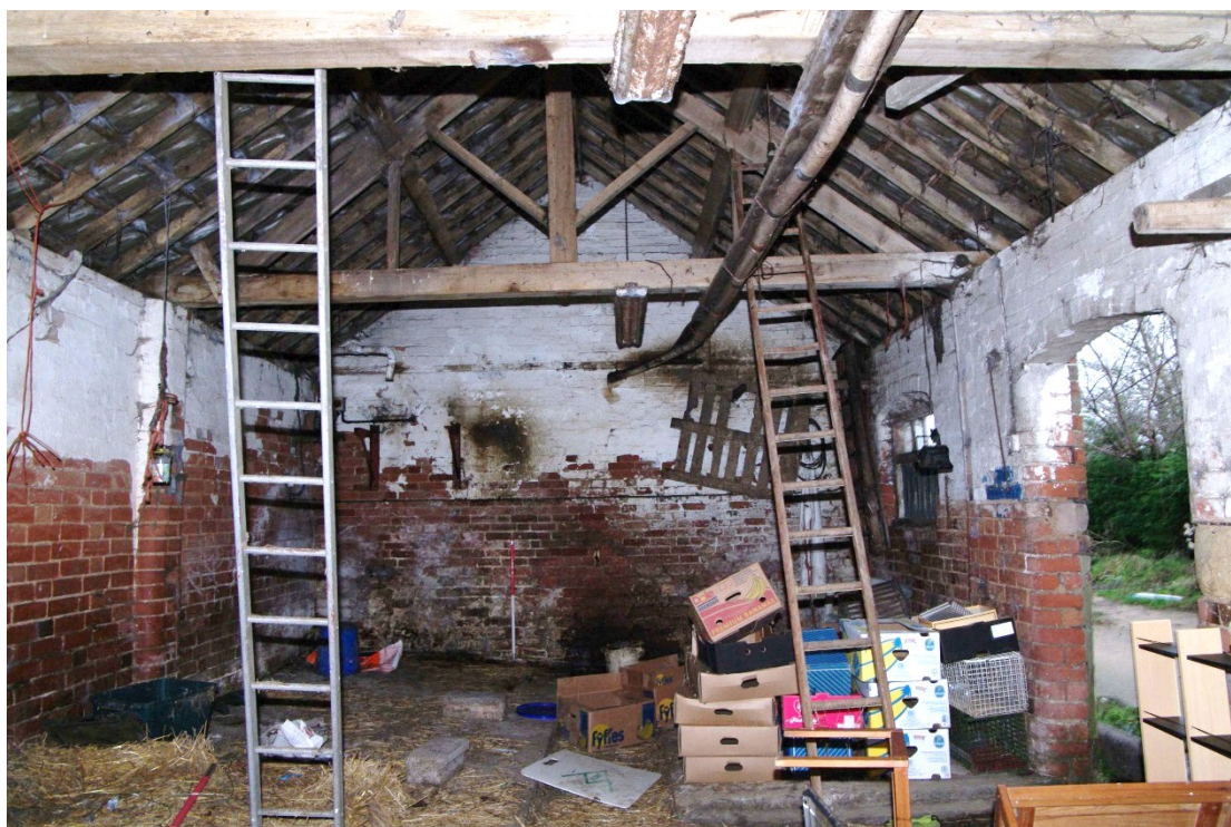
Figure 99 North to south barn. Room 3 Looking south. 1m scale
