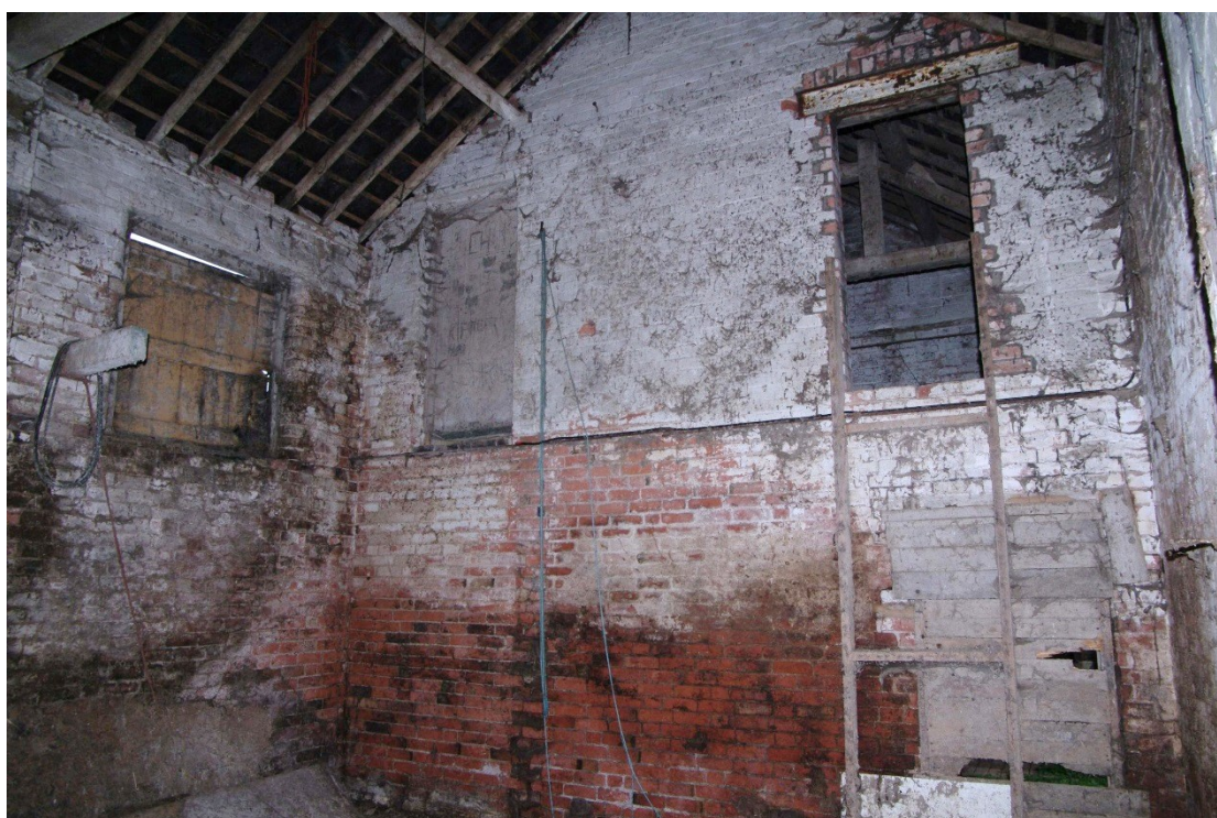
Figure 96 North to south barn. Room 1 south end wall Looking south-east
