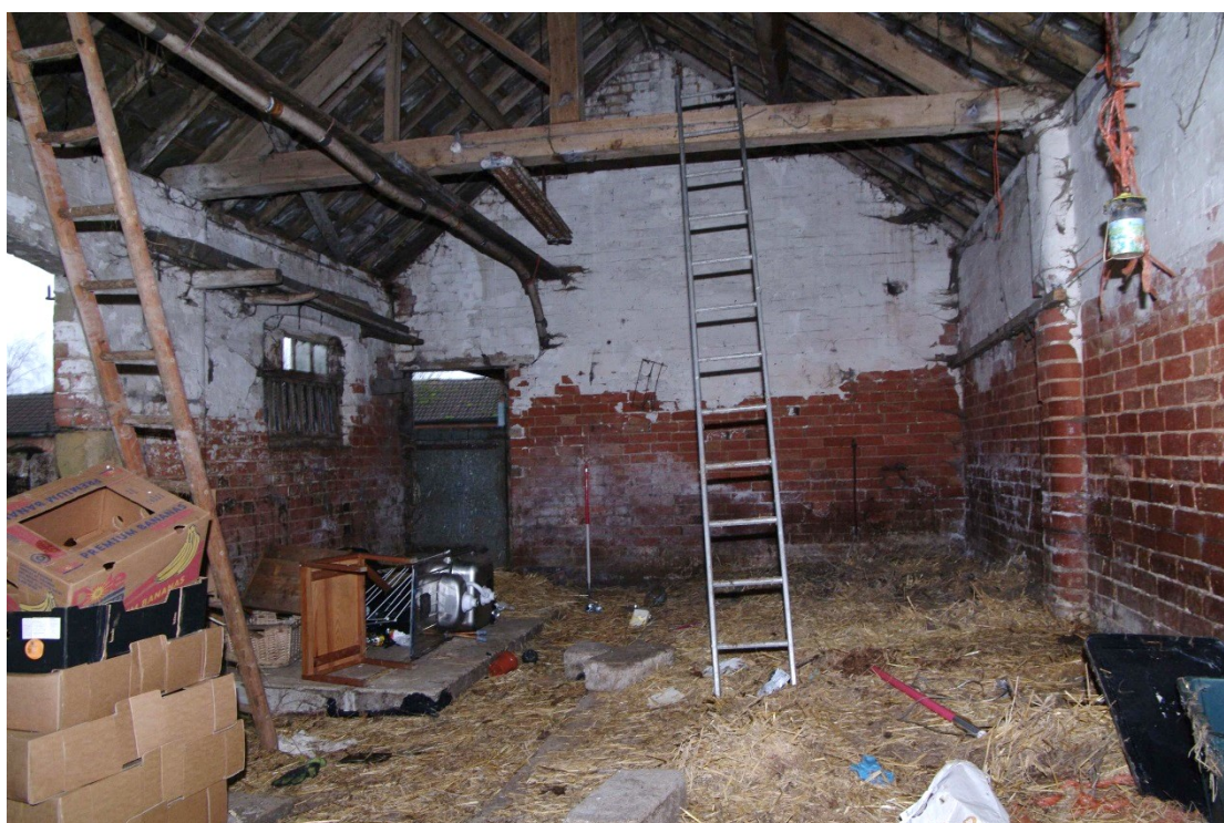
Figure 98 North to south barn. Room 3 Looking north. 1m scale
