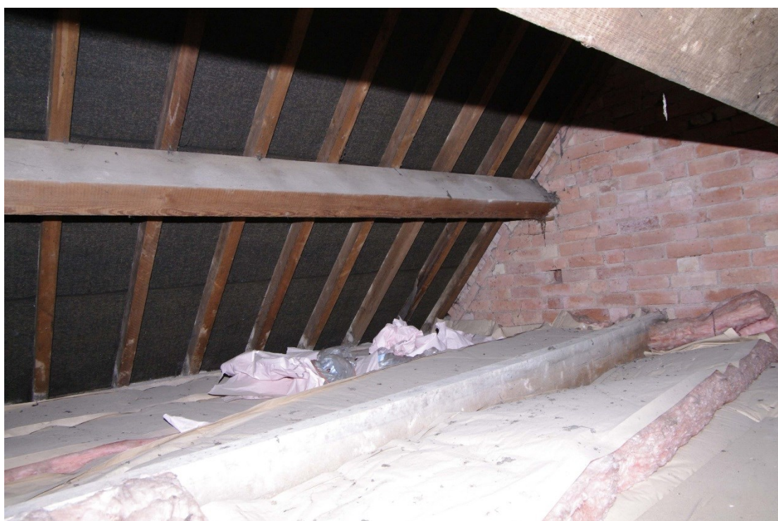
Figure 77 Roof structure above Room 14 Looking south-west
