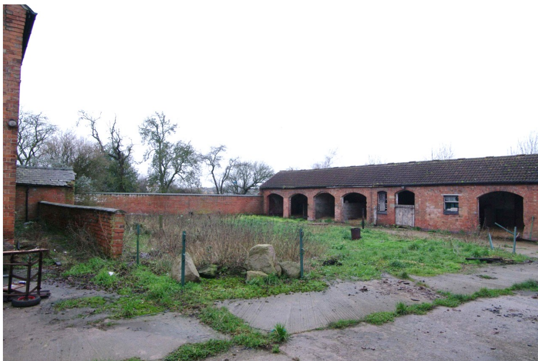
Figure 104 East to west barn and foldyard Looking north-west
