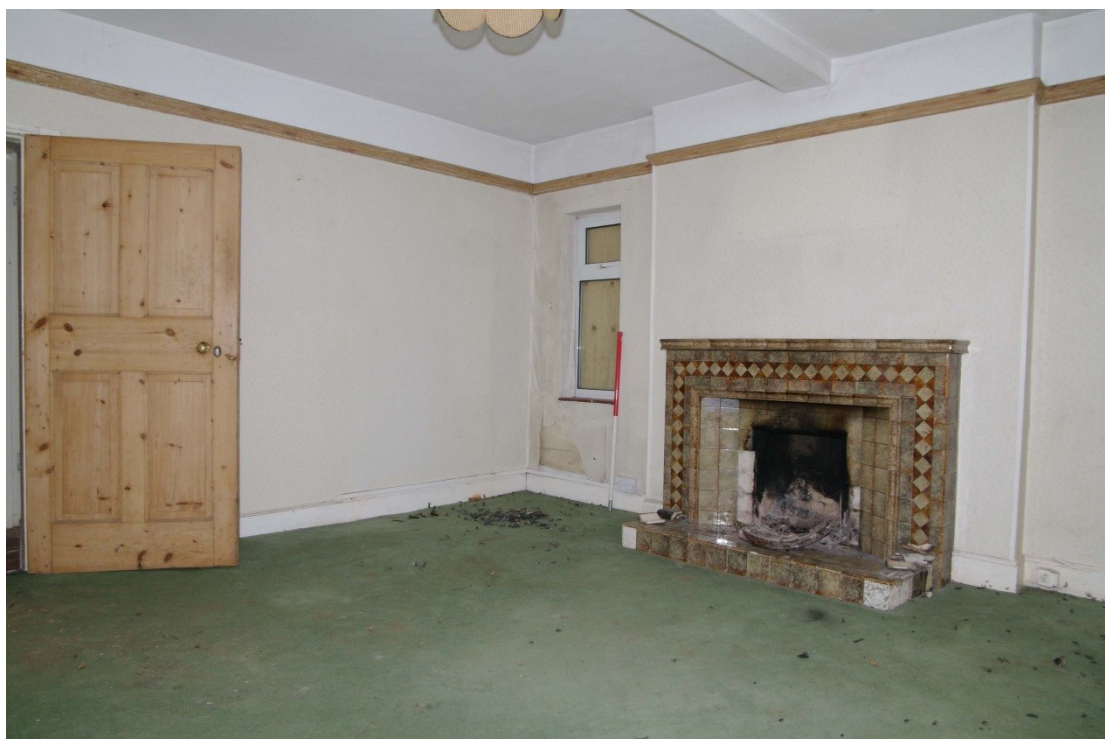
Figure 40 Room 2 general view Looking south-east. 1m scale
