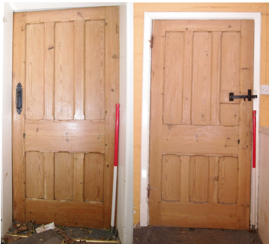
Figure 51 Room 6 door detail Left: outside, right: inside. 1m scale
