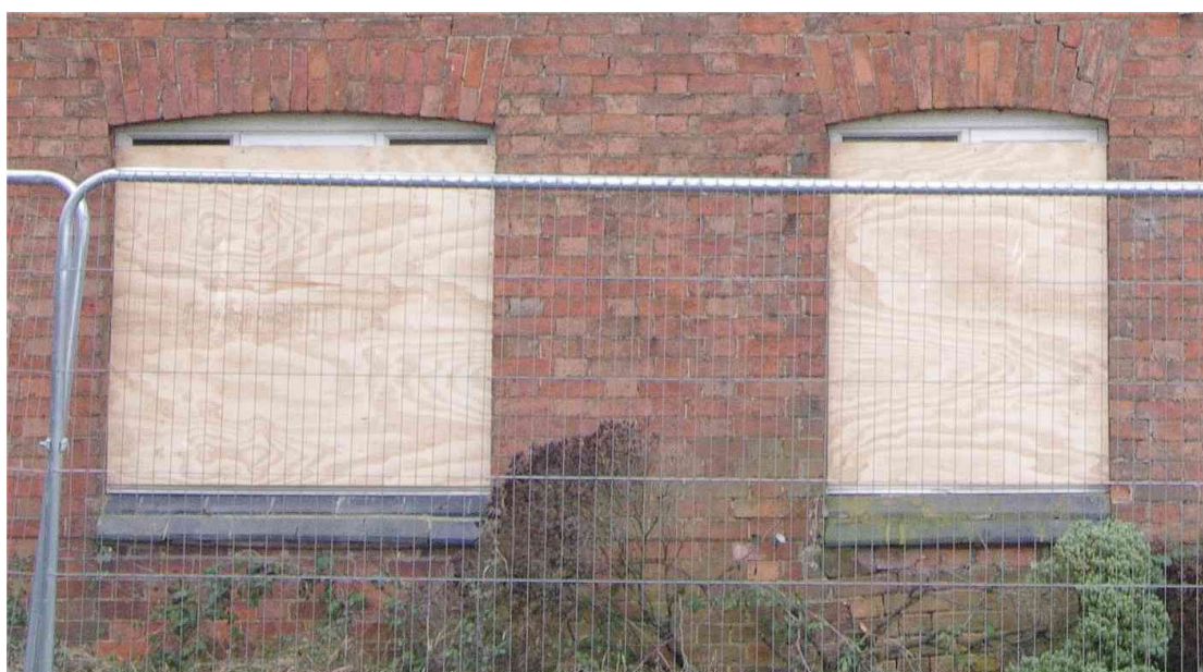
Figure 11 Farmhouse west facing elevation ground floor window detail Looking east
