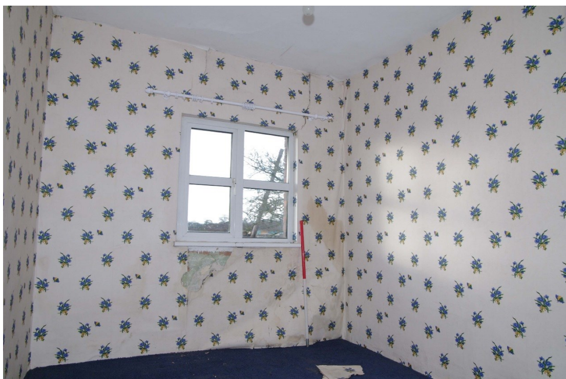
Figure 63 Room 9 Looking north-west. 1m scale
