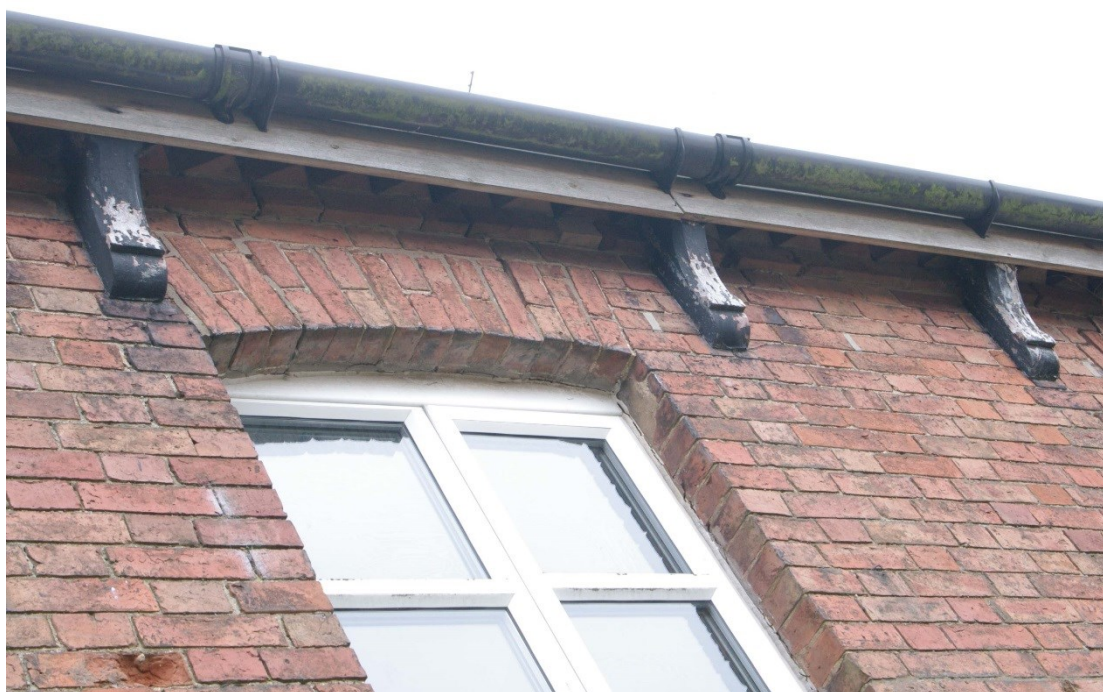
Figure 13 Farmhouse west facing elevation eaves detail
