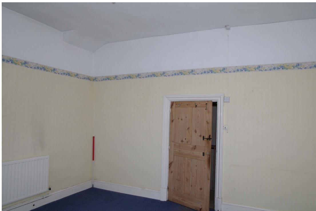
Figure 74 Room 13 Looking south-east. 1m scale. Note step in ceiling, top left
