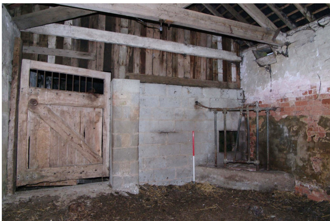
Figure 123 East to west barn. Room 6 Looking north-west. 1m scale
