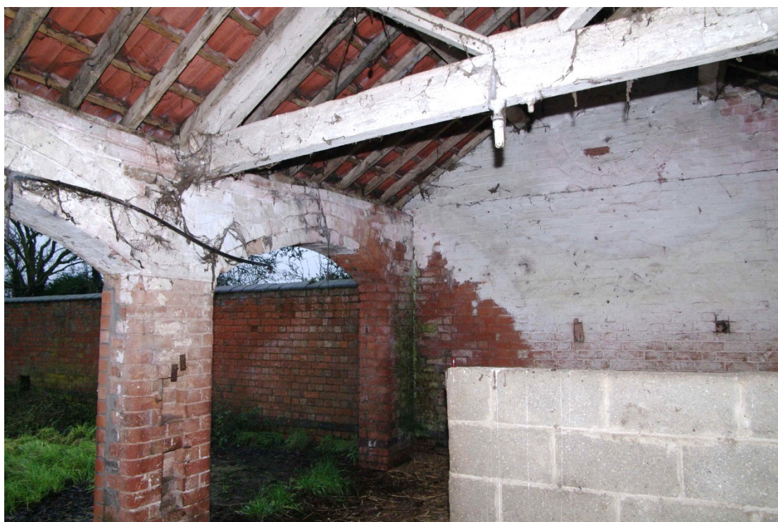
Figure 115 East to west barn, Room 1 Looking south-west
