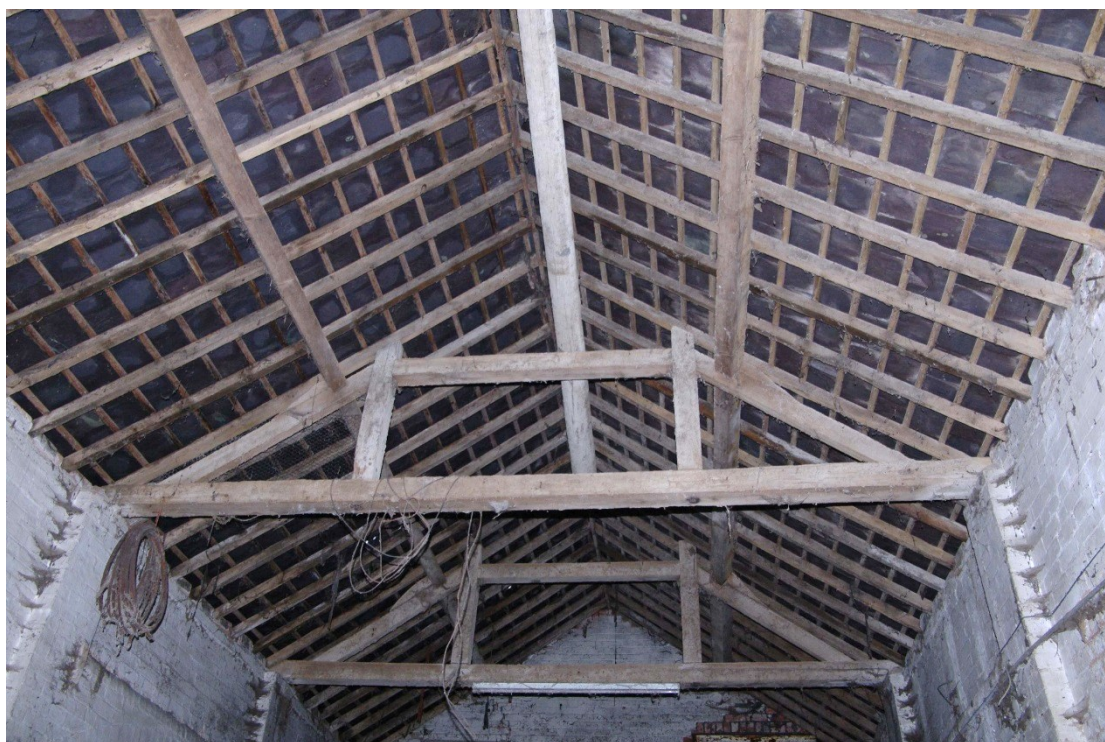
Figure 95 North to south barn. Room 1 roof structure Looking north
