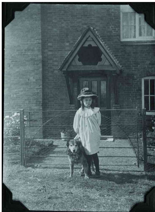
Figure 16 The porch in 1926 Looking north. Note lack of windows on left side of porch, compare with Figure 15 above. Photo courtesy of Carole Frost
