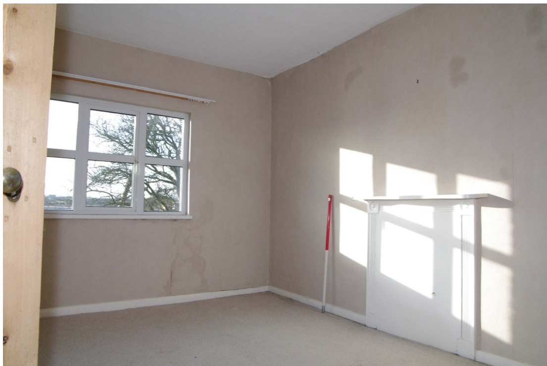
Figure 64 Room 10 Looking north-west. 1m scale
