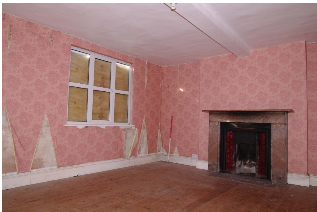
Figure 41 Room 3 Looking north-west. 1m scale
