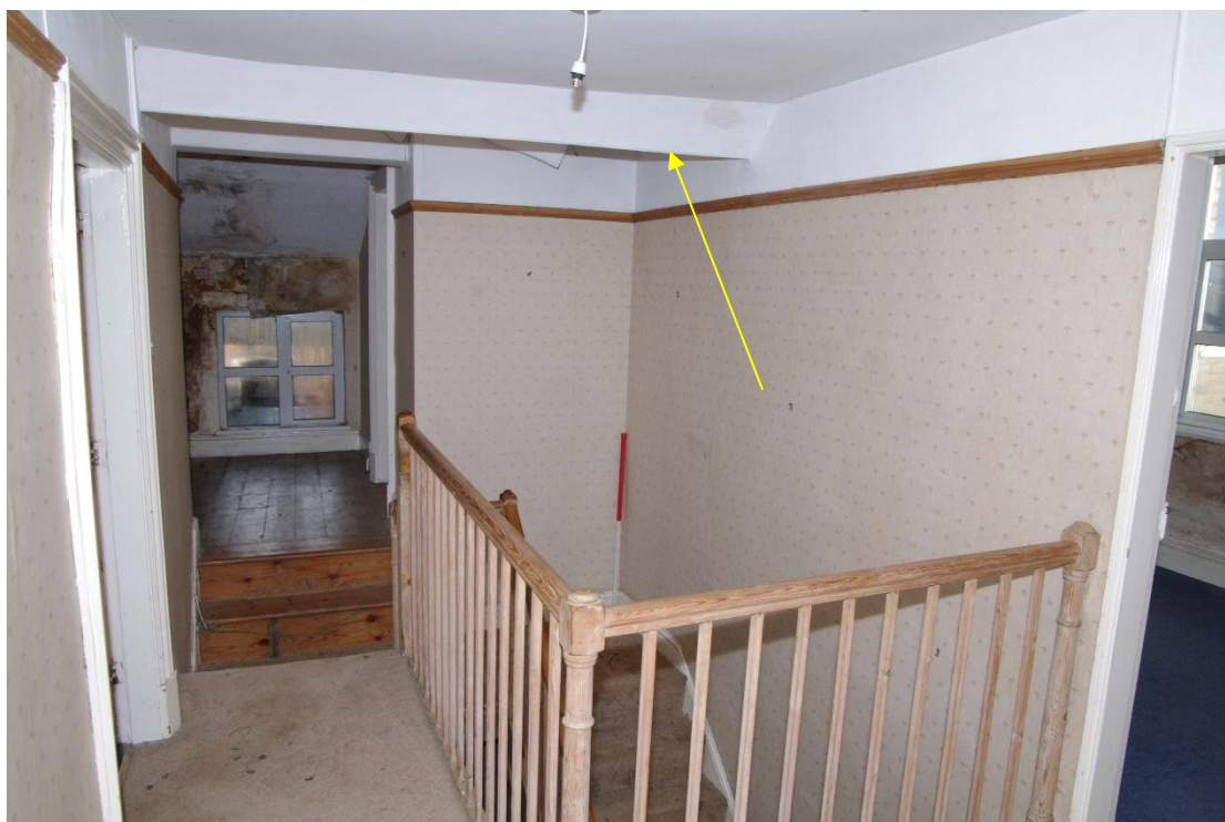
Figure 69 Room 12/landing Looking south-east. 1m scale. Doorway to Room 11 on right. Note purlin (arrowed)
