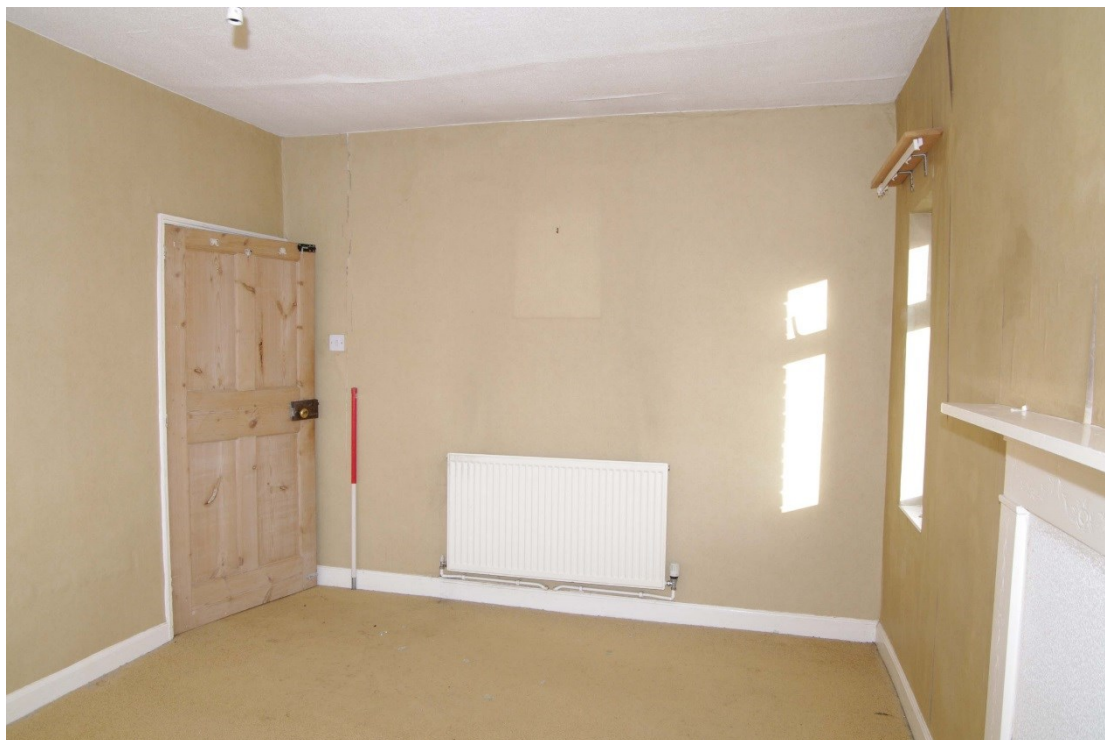
Figure 60 Room 8 Looking north-east. 1m scale
