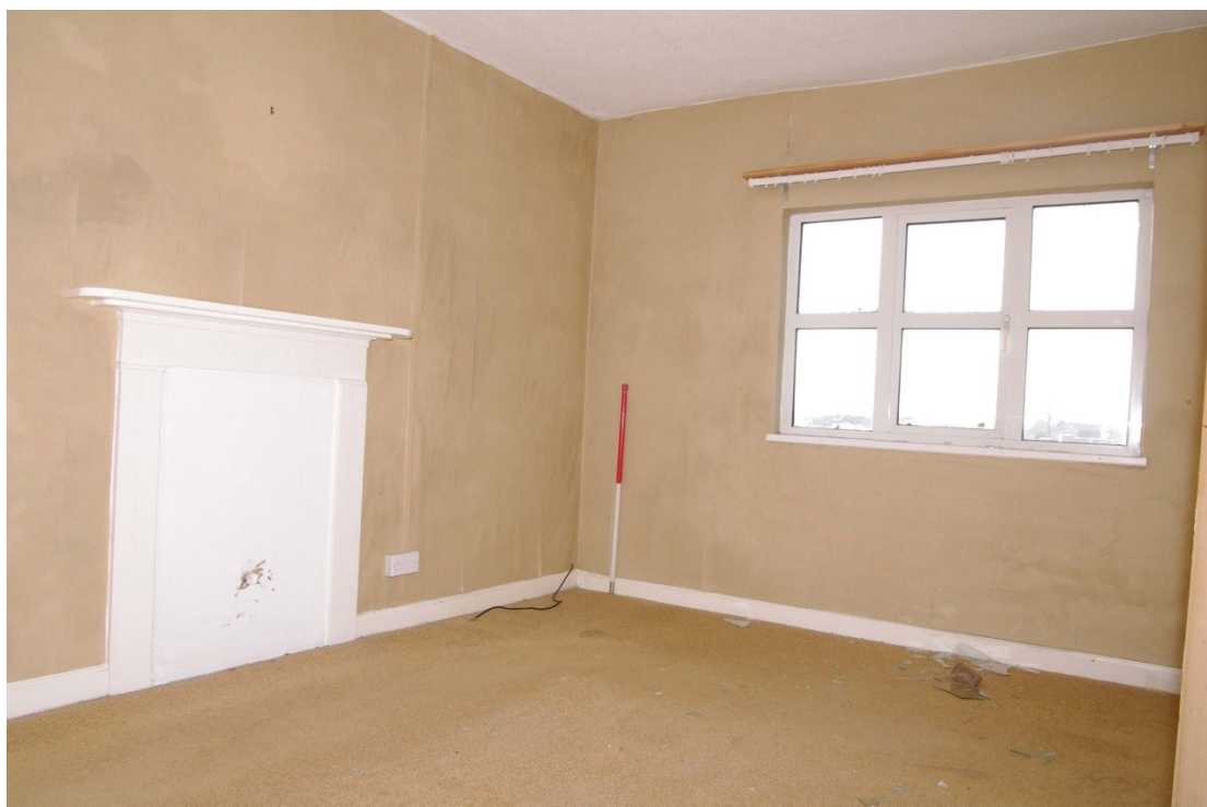
Figure 61 Room 8 Looking south-west. 1m scale
