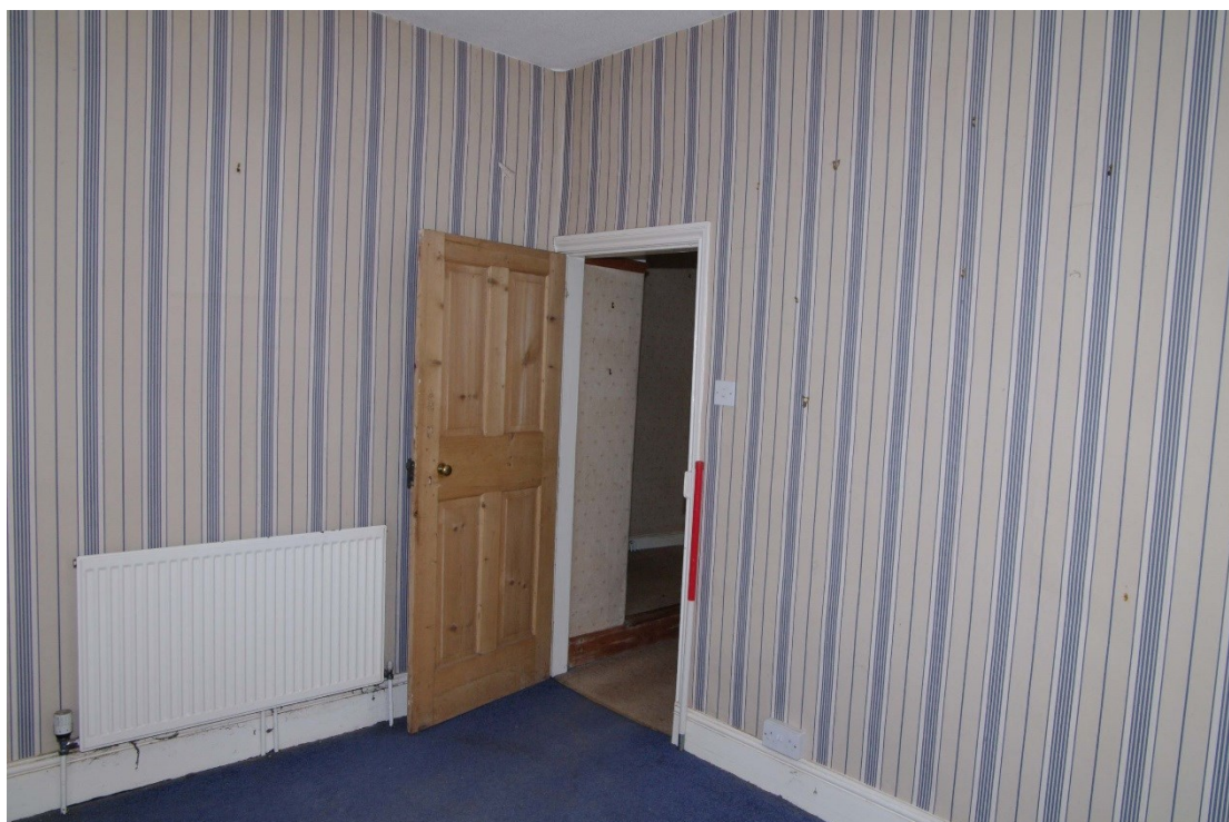
Figure 65 Room 11 doorway Looking north-west. 1m scale
