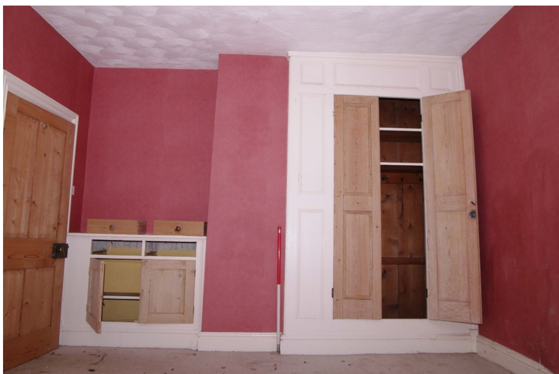
Figure 79 Room 15 Looking west. 1m scale. Door to landing on left
