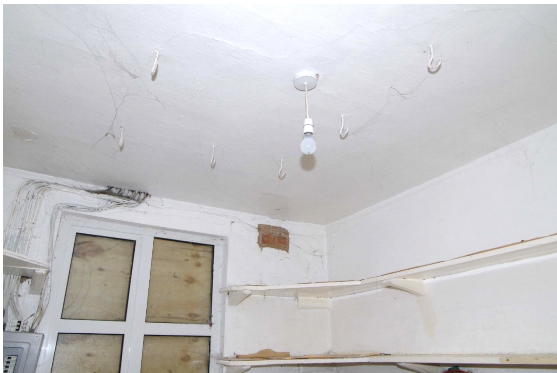
Figure 45 Room 4 hooks in ceiling Looking south-west
