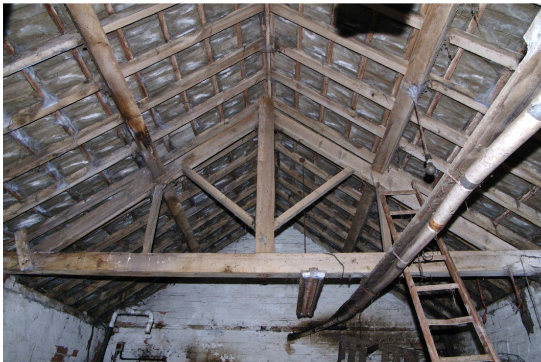
Figure 101 North to south barn. Room 3 roof detail Looking south
