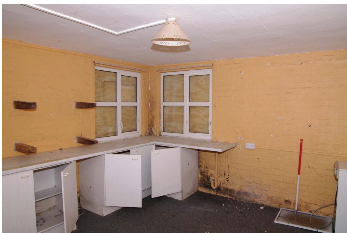
Figure 50 Room 6 Looking north-east. 1m scale
