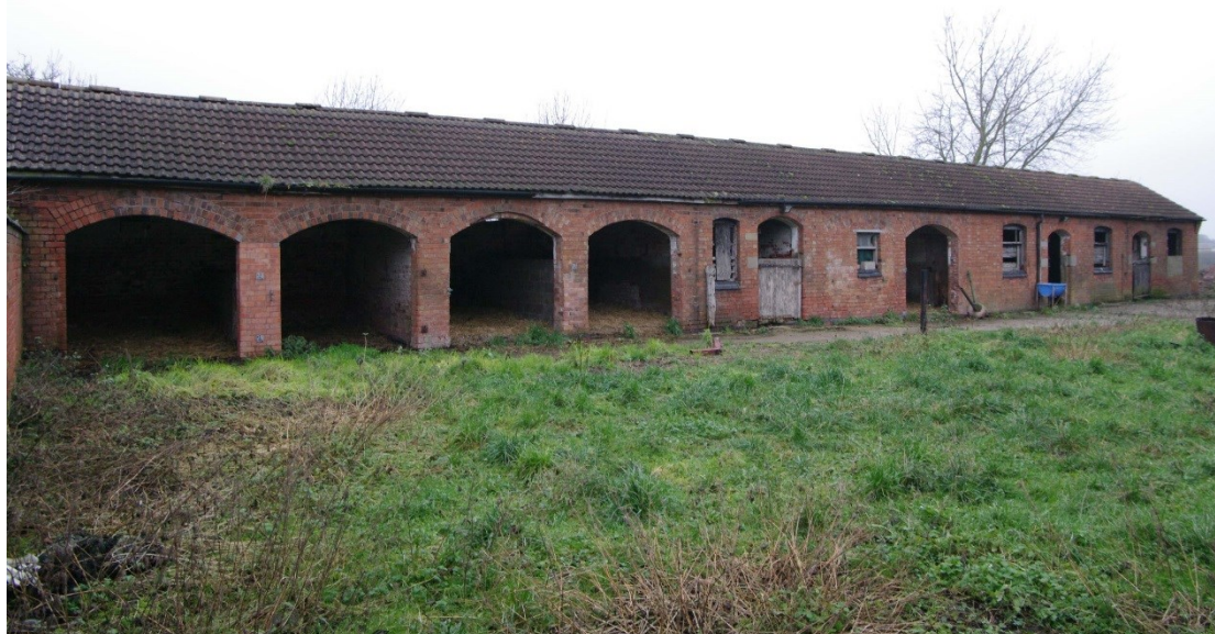
Figure 105 East to west barn. South facing elevation Looking north-east
