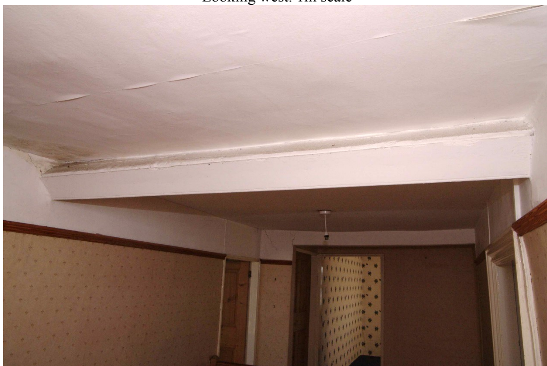
Figure 71 Room 12/landing Purlin detail above staircase
