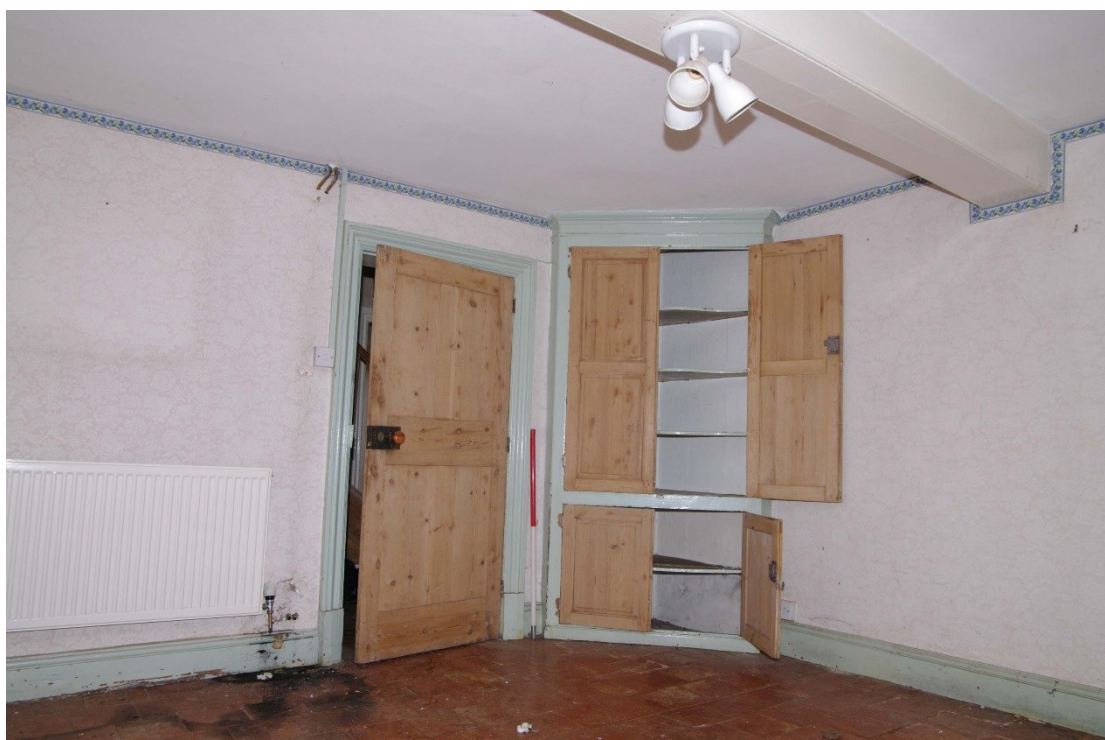
Figure 47 Room 5 Looking south-west. 1m scale
