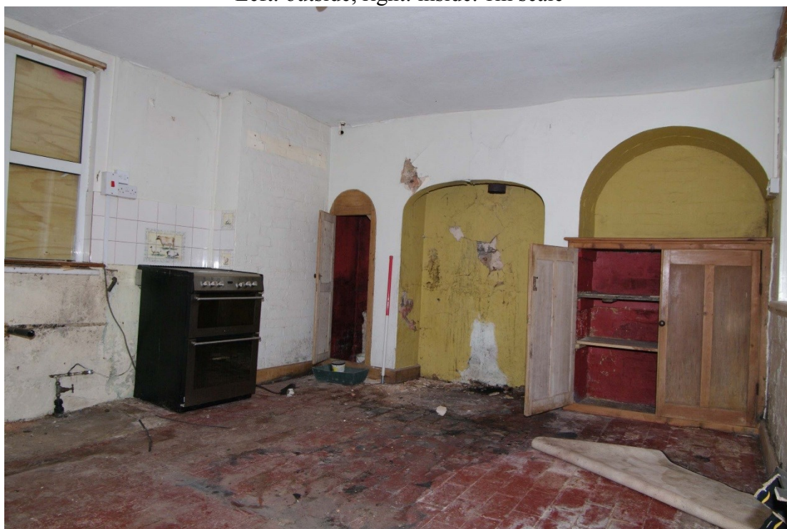
Figure 52 Room 7 Looking north-east. 1m scale
