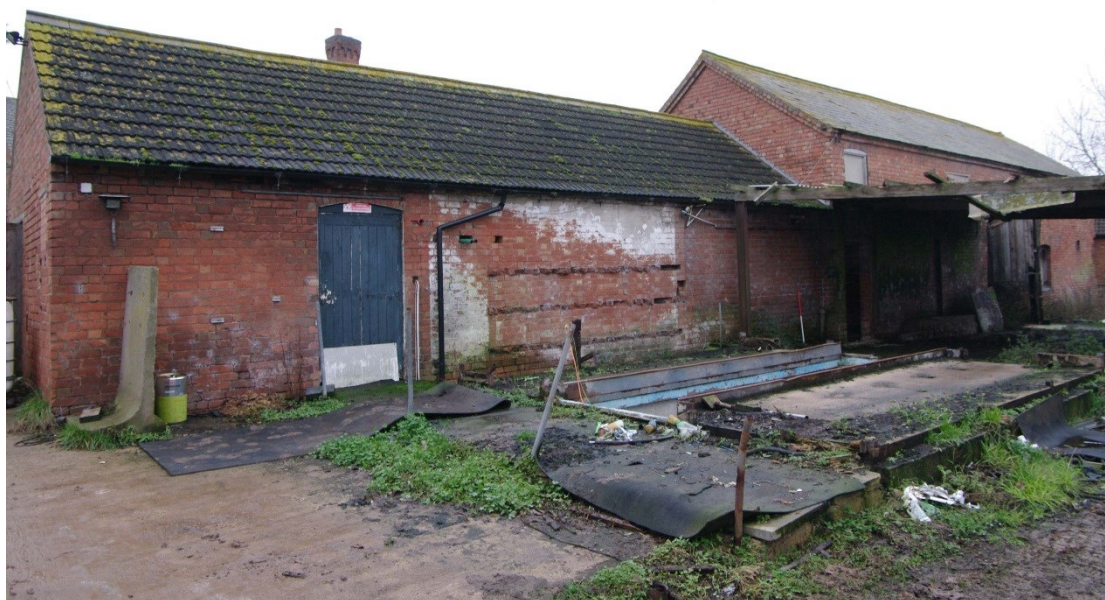
Figure 87 North to south barn. East facing elevation Looking north-west. 1m scale
