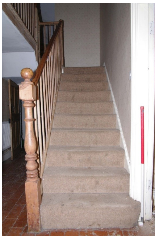
Figure 37 Staircase in hall Looking east. 1m scale
