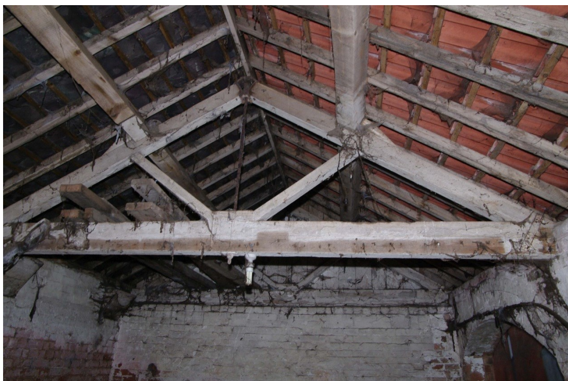
Figure 116 East to west barn. Roof detail Looking east
