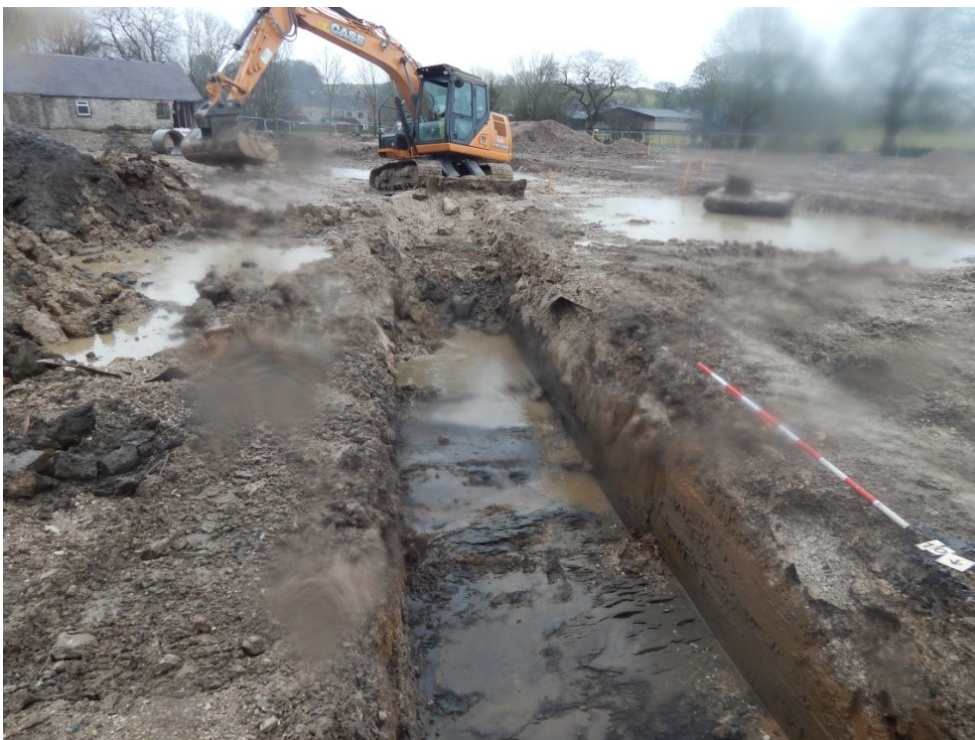
Figure 6: Excavation of the trenches
