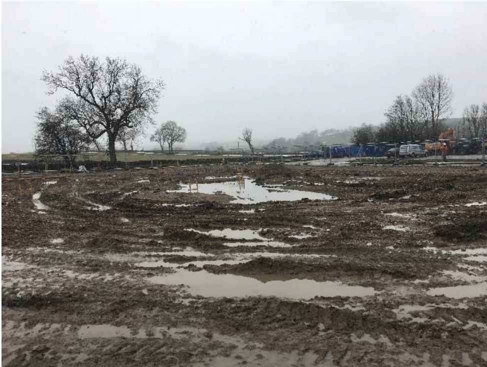
Figure 5: Application area, looking South- West
