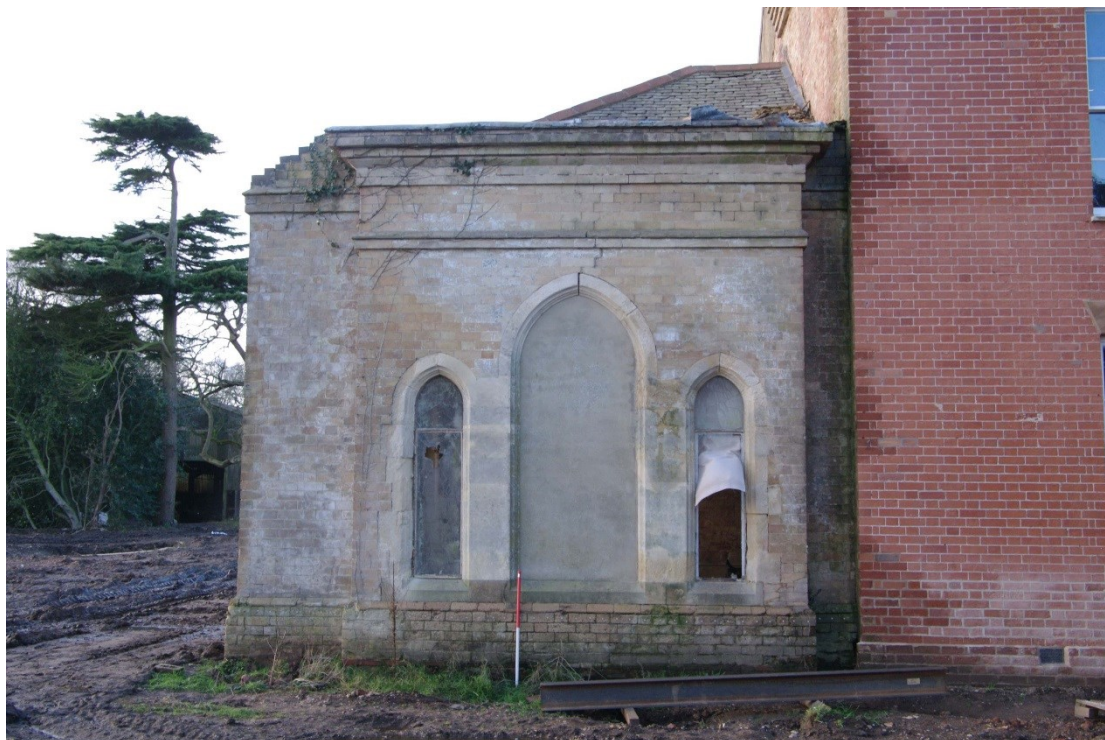
Figure 7 East facing elevation of morning room Looking west. 1m scale
