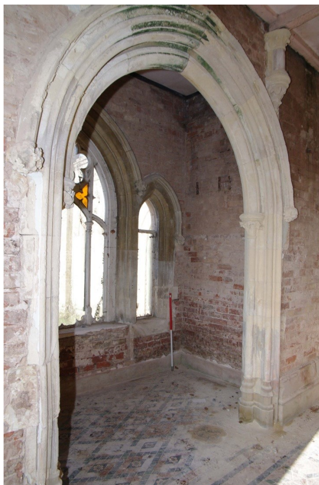
Figure 29 West end of morning room Looking north-west. 1m scale
