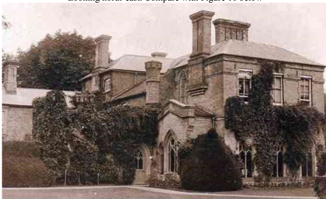
Figure 10 West and south facing elevations of morning room c1900 Looking north-east
