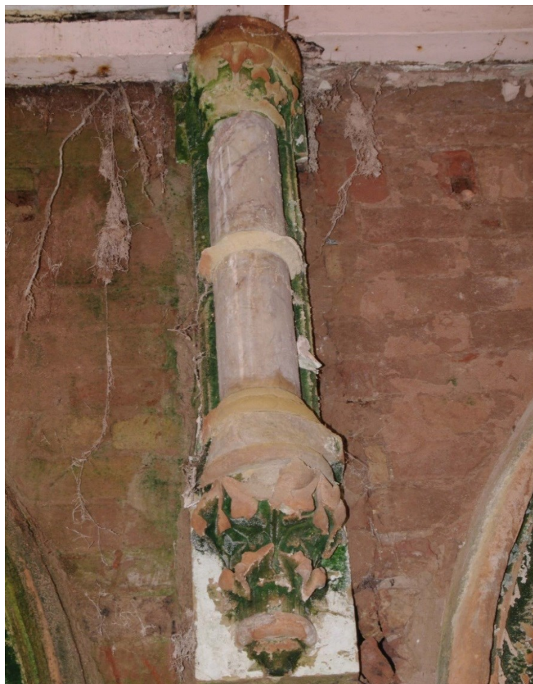
Figure 17 Original stone and marble ceiling support North-east corner of room
