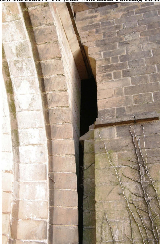
Figure 12 Close up of joint on west facing elevation Looking east
