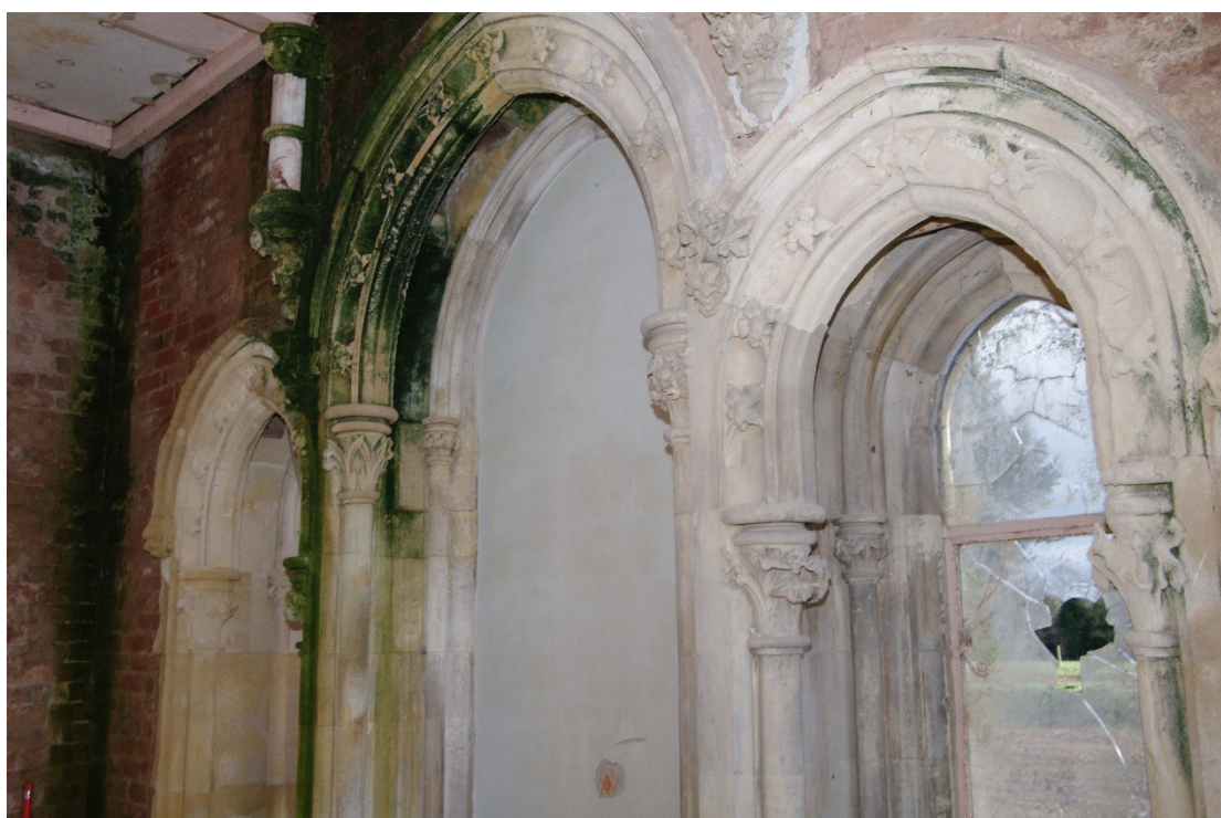
Figure 22 East wall close up of detail around lancet windows Looking north
