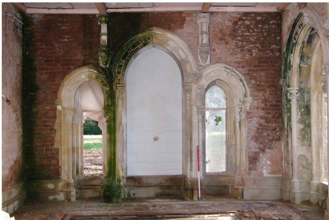
Figure 21 East internal wall of morning room Looking east. 1m scale. The centre window will be unblocked
