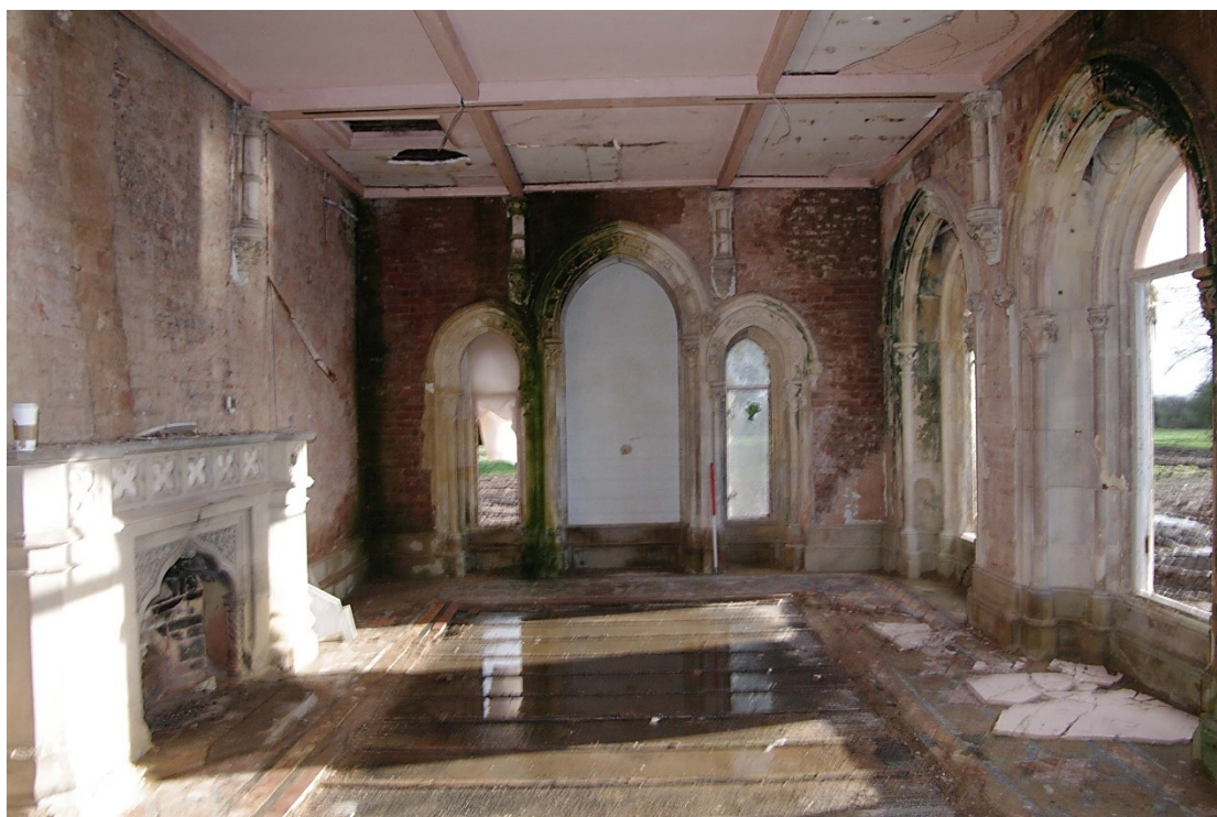
Figure 14 Morning room general view Looking east. 1m scale
