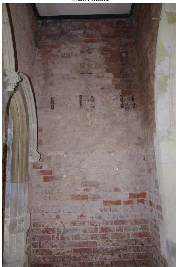
Figure 32 Brackets on south wall of recessed orangery Brackets show where vaulted ceiling was supported
