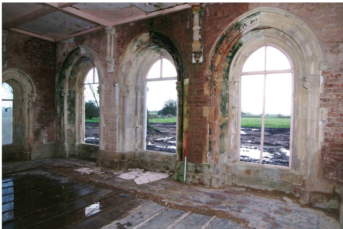
Figure 23 South wall general internal view Looking south-east. 1m scale
