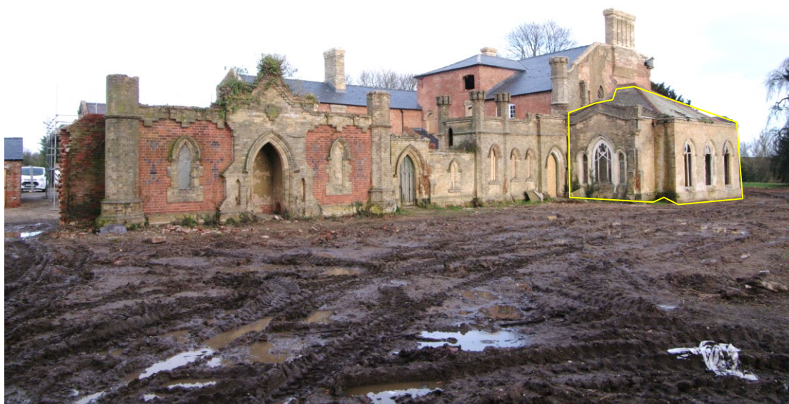
Figure 5 West facing elevations of morning room and rear outbuildings Looking south-east. Morning room on right of picture (outlined)
