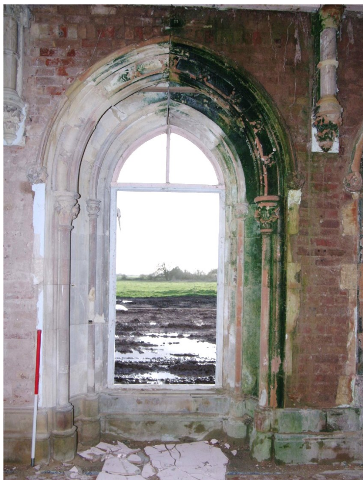
Figure 25 South wall, centre window internal detail Looking south. 1m scale
