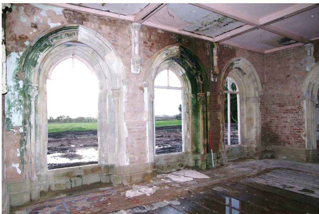
Figure 24 South wall general internal view Looking south-west. 1m scale
