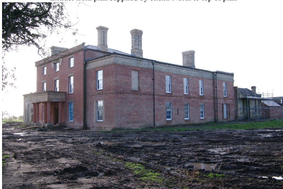
Figure 3 Heather Hall north and east facing elevations Looking south-west. Morning room on far left behind added-on porch. Original 18th century farmhouse core in centre with later added wing to right. Part of stable block on far right of picture
