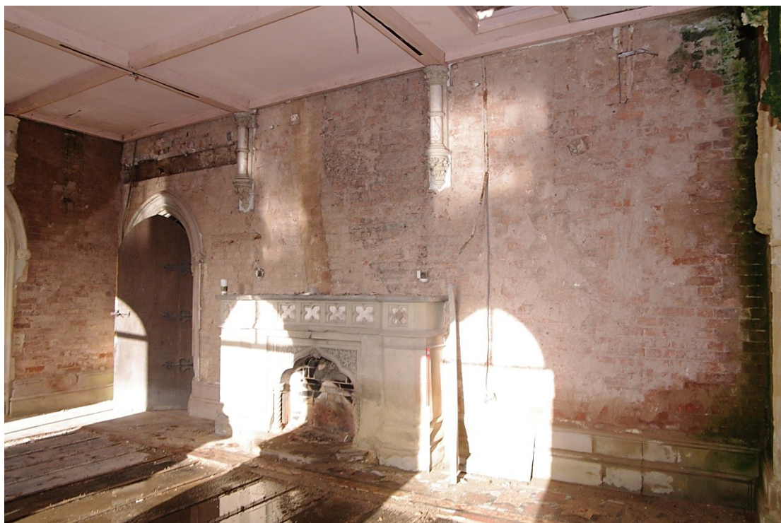
Figure 19 North internal wall of morning room Looking north-west
