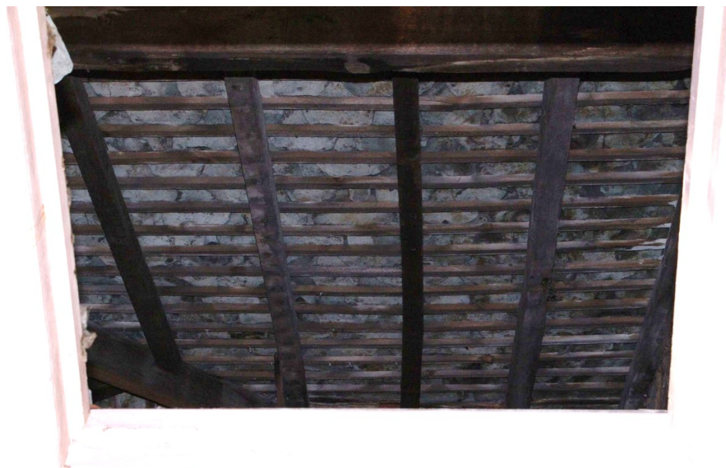
Figure 16 Underside of slates seen through hatch in ceiling
