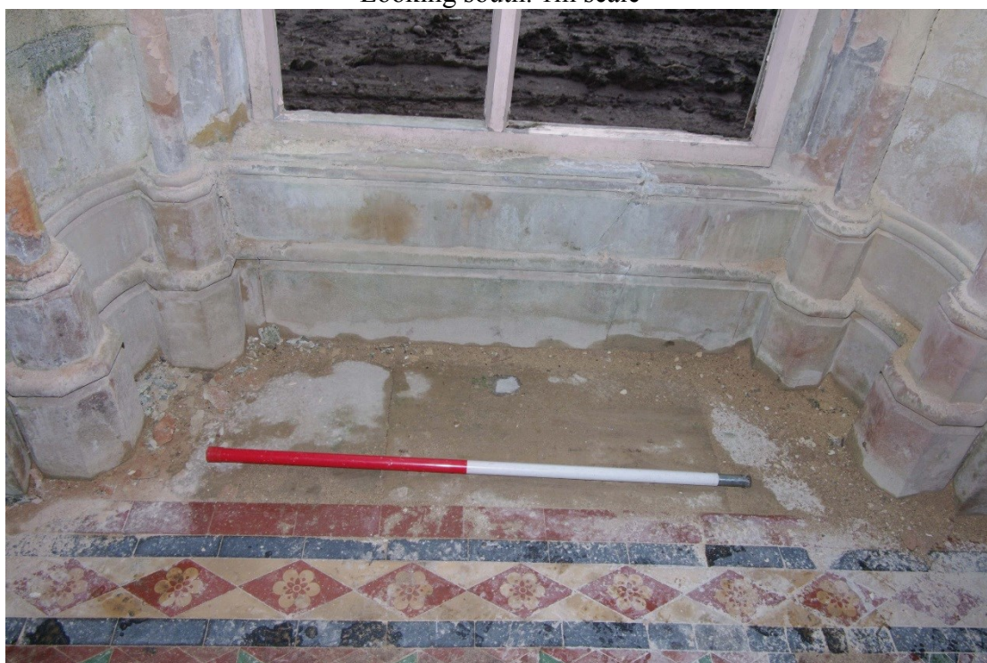
Figure 26 South wall window moulding detail 1m scale
