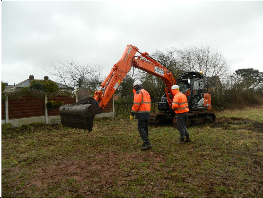
Figure 7: Mechanical excavator looking north
