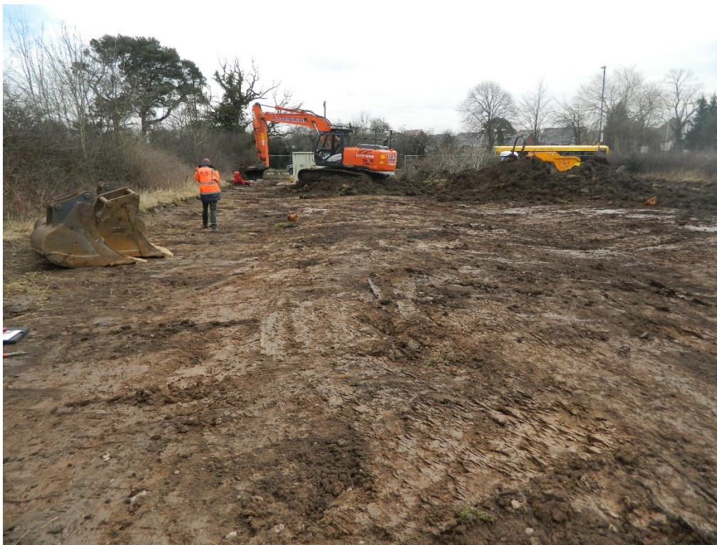
Figure 10: Site stripped of overburden looking south-east.
