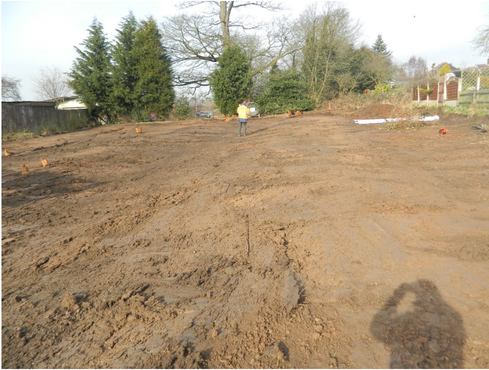
Figure 9: Site stripped of overburden apart from made ground remaining in furrows as dark 'stripes'. Looking north-west.
