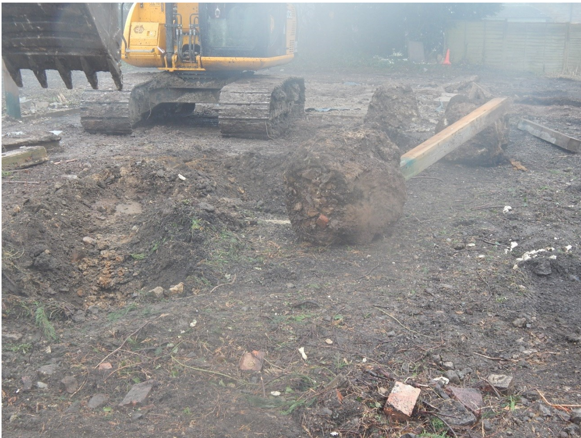
Figure 7: Posts with large concrete plugs being removed
