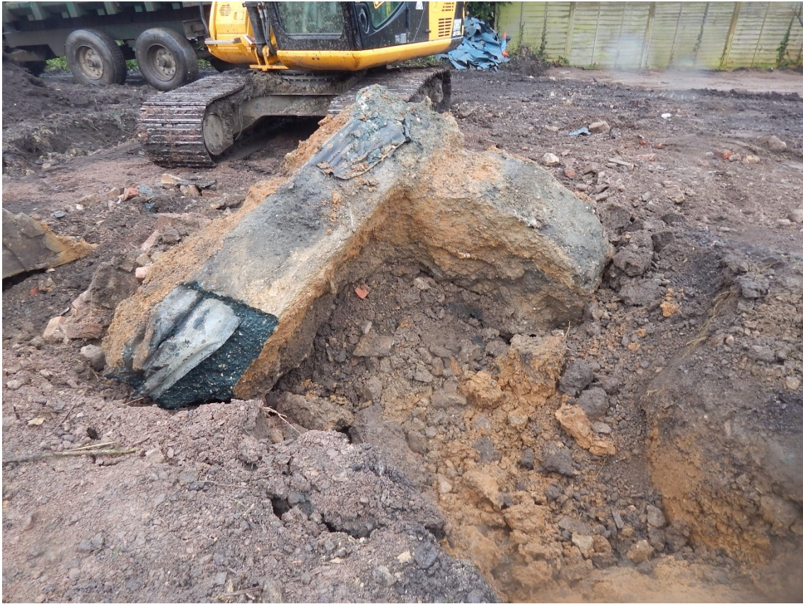
Figure 6: Concrete footings being removed from northern half of development area.
