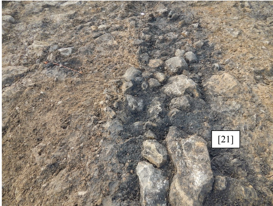
Figure 19: Pipe trench containing large masonry blocks of sandstone.
