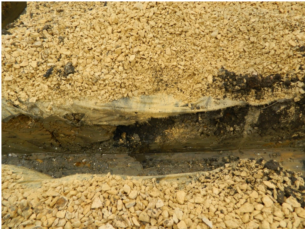
Figure 26: Dark top soil marks the site of previous 20th century concrete footings. Facing north.
