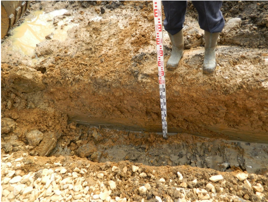
Figure 25: Depth of foundation trenches, looking east.
