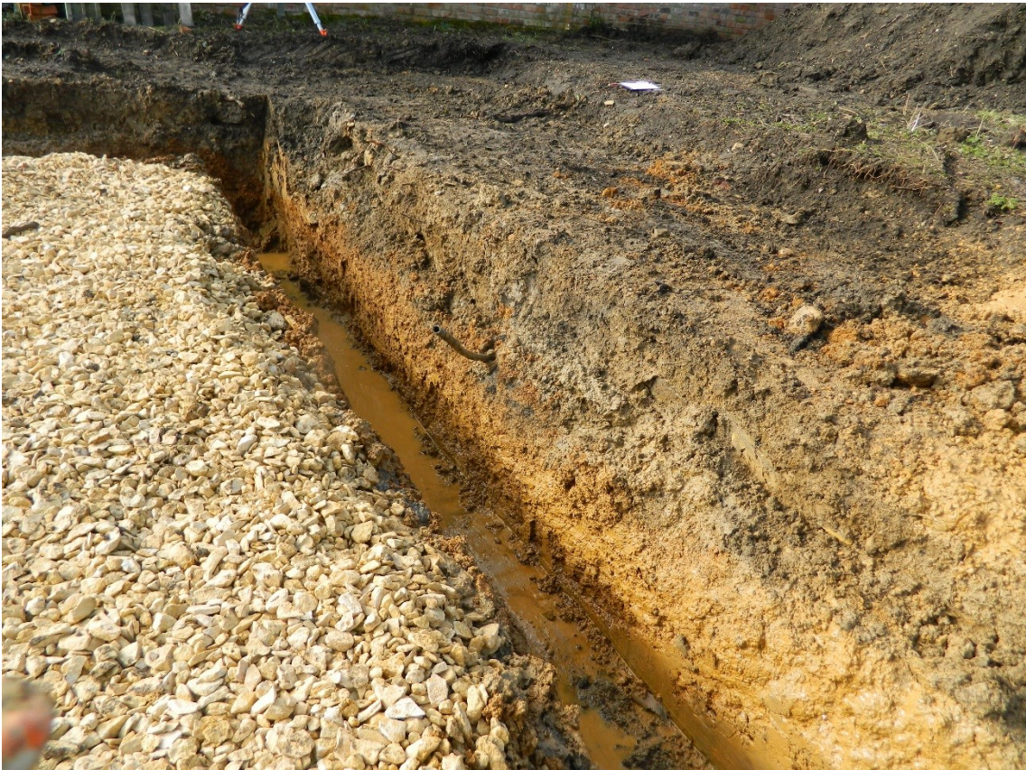
Figure 10: Foundation trenches. Looking south.
