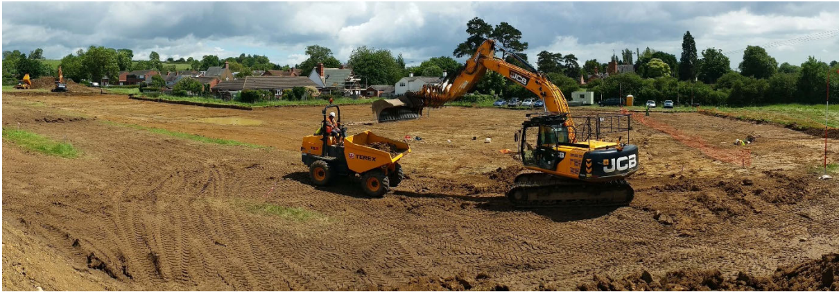
Figure 4: General view east of machine strip in progress
