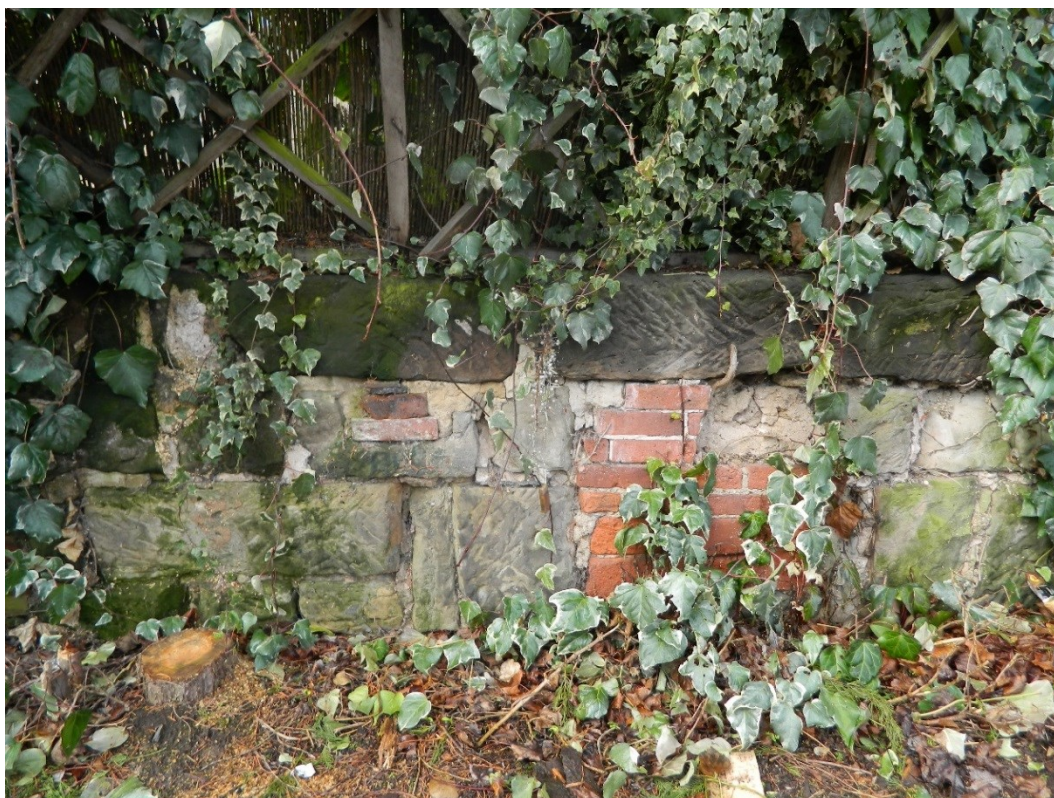
Figure 19: The western boundary wall including dressed stones probably from the castle, looking west
