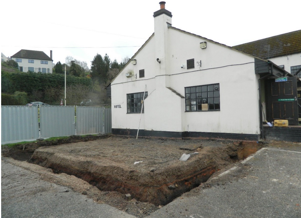
Figure 7: Post excavation shot of Area 1, looking south east
