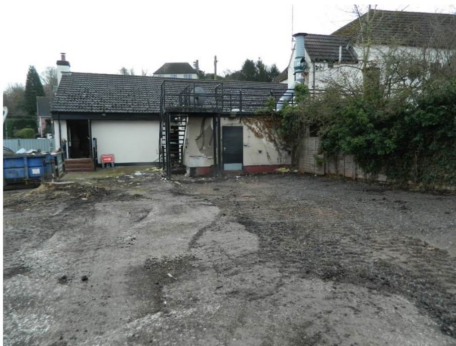
Figure 15: Pre-excitation shot of Area 2, looking south-east
