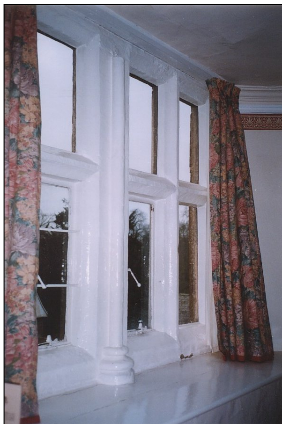
Plate 22. First floor C16 window in the south-east gable showing the capital detail missing.
