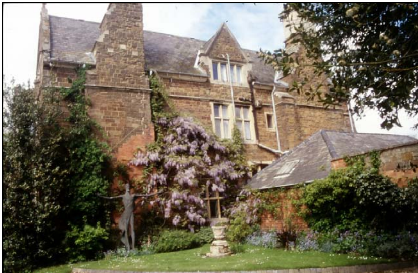
Plate 5. Launde Abbey: South elevation & brickwork scar of demolished C19 range at SW corner (behind statue)
