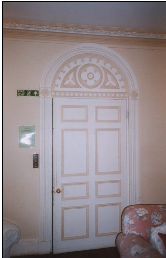
Plate 29. Sitting Room 1 door showing eight panelled door with reeded detailing, decorative paterae and Gothic decoration in the rounded head above the door.
