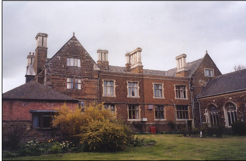
Plate 28. East (rear) elevation of house, showing the two distinct types of stone and chimneys in the work attributed to Thomas Rickman, 1829.
