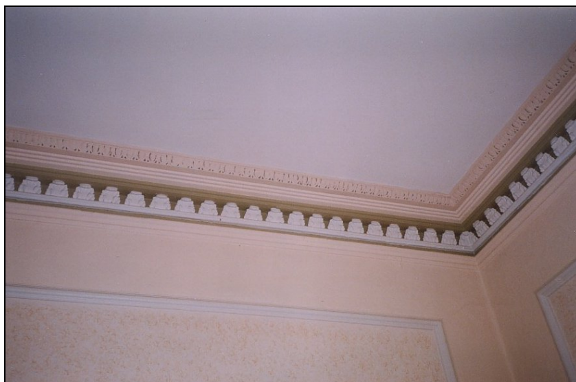
Plate 30. Detail of the plaster moulding in the south-west ground floor room ( Seminar Room 2 ).
