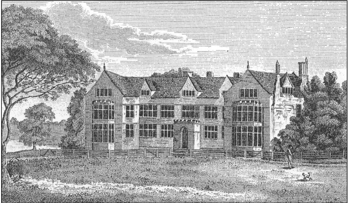
Figure 5. Launde Abbey: West front, from the SW. Illustrated in Nichols 1800 (at top of Plate XLV). Note the discrepancy in sill height between the windows of the centre range and canted bays of the cross wings.
