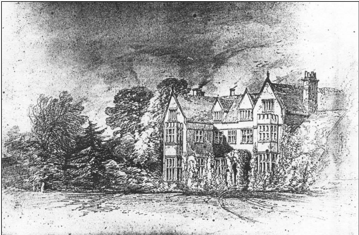
Figure 7. Undated 19th Century engraving in the possession of Launde Abbey. Note the two-storey addition to the SW corner of the house, with first floor window just visible in the gable end. This must have been built after c. 1800 and was demolished some time between 1884 and 1904.
