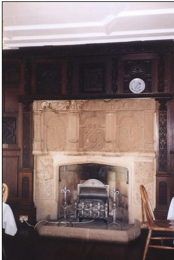
Plate 33. Fireplace in Dining Room showing as two distinct sections with the lower section, including the 4-centred arch being a C19 Gothic replication and the section dated 1689 which has frieze detailing at its top, wrongly relocated to its present low level.
