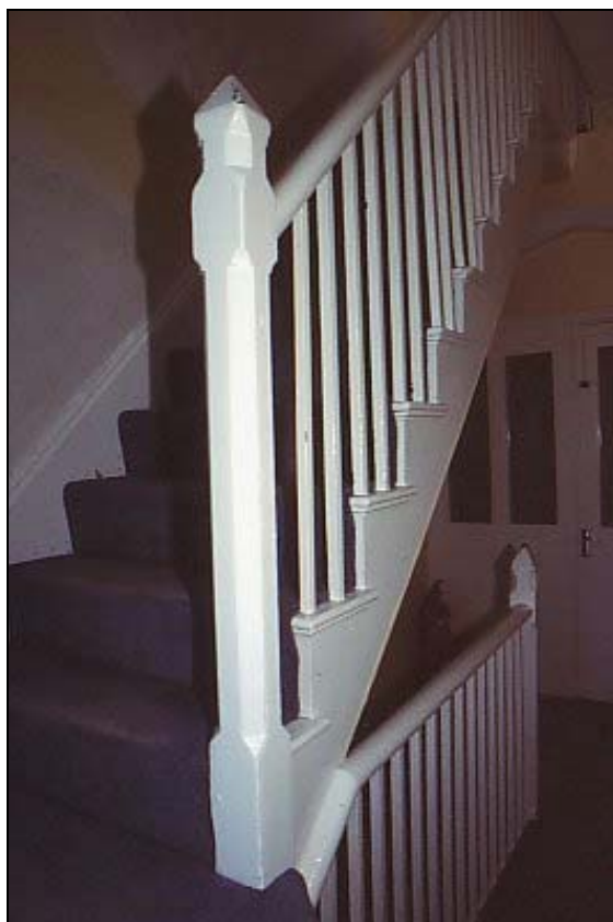
Plate 34. Service staircase with stick balusters and cut and chamfered newels with faceted finials.
