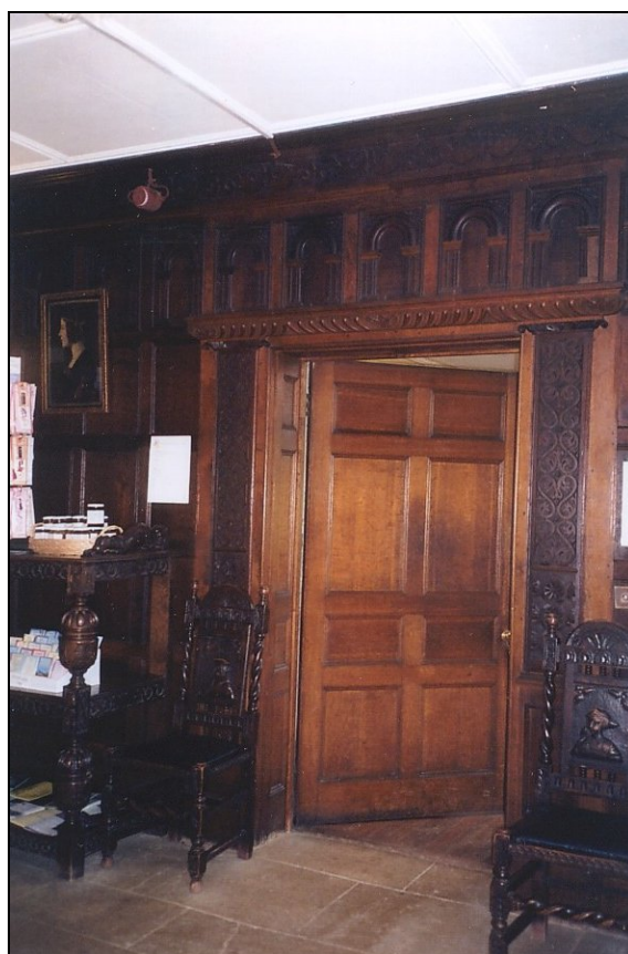
Plate 31. Section of the Entrance hall panelling showing mixture of strap motif panels with arcading, gadrooning and serpent motifs at frieze level.
