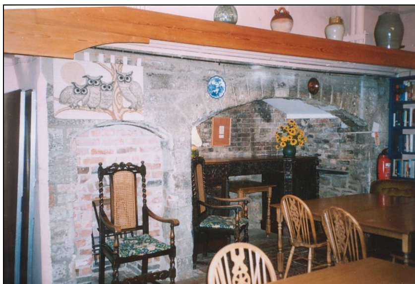
Plate 21. Fireplace with extended, low arch form, of characteristic late C16 form in the present Library , which is identified as the Kitchen on earlier plans.
