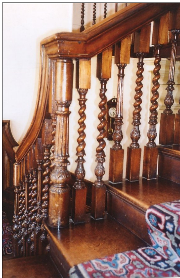
Plate 26. Detail showing staircase with two twisted and one fluted baluster to each tread, carved newel and ramped handrail.
