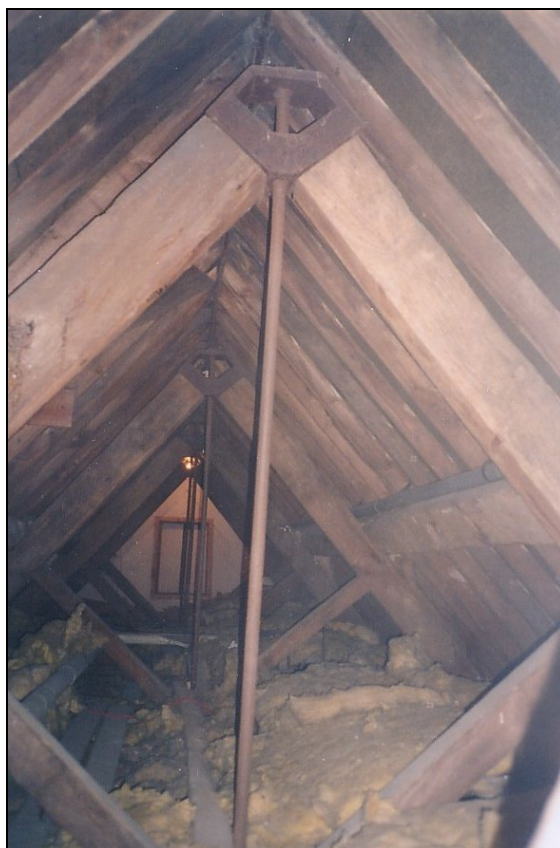
Plate 36. View through the roof of the main front of the house, showing the bolted, deal trusses with cast-iron yoke at the apex.
