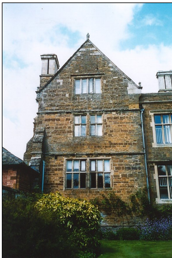
Plate 20. South-east gable showing the rising series of early C16 windows, particularly the paired, six-light ground floor window.
