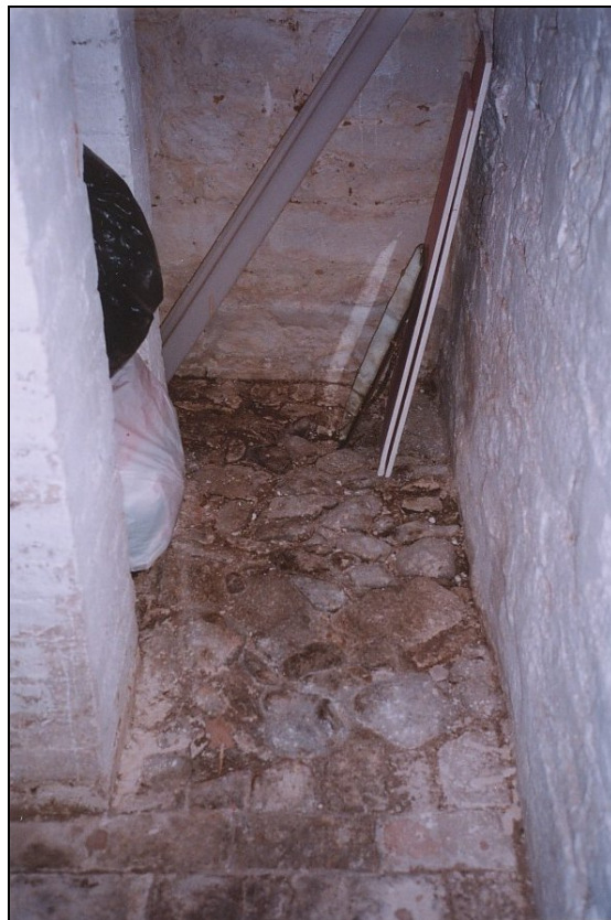
Plate 19. Detail showing section of roundstone cobbling in cellar floor adjacent to 'spine wall' ( Library Area ).
