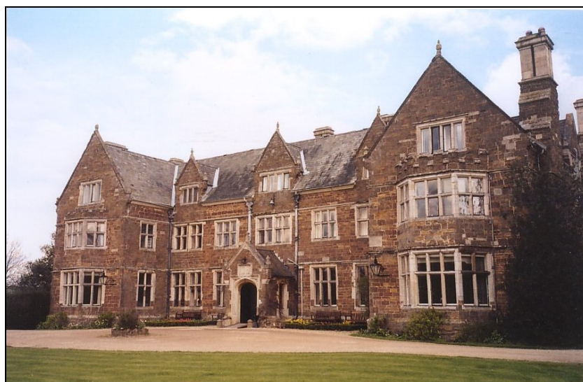
Plate 23. West front of Launde Abbey from SW. The ironstone sections set into the lower part of the ground floor windows of the main range can be seen as a dark band at the base of the windows.
