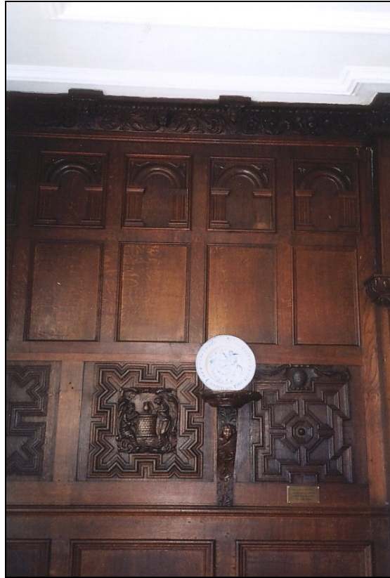
Plate 32. Detail of C19 rails and stiles with sections of C17 set into them and C19 Flemish carved vignettes planted on them. The arcading and the carved frieze are also C19 compilations.
