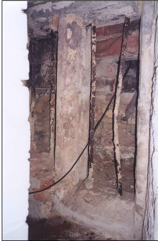
Plate 18. Detail of splay mullion window in 'spine wall' of the house in lower ground floor Library Area . Showing glazing bars still in situ and rubble fill behind.
