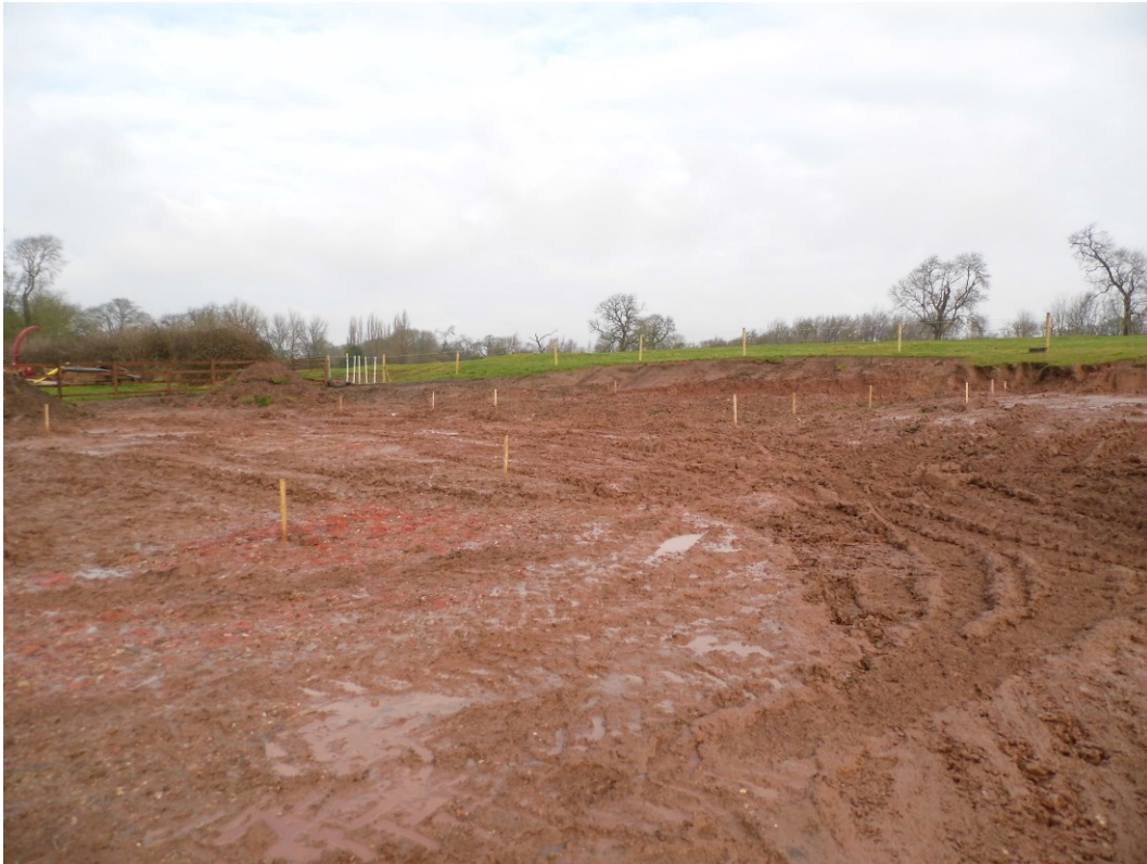
Figure 5: Photograph of the site (looking north-west) prior to trenching.
