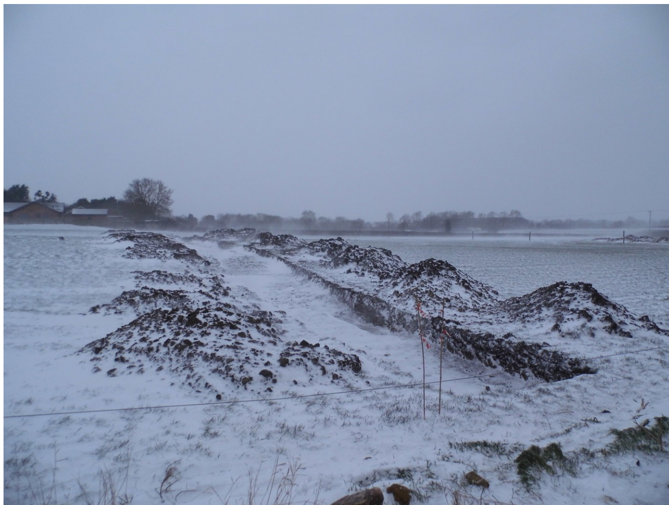
Figure 5: Challenging weather conditions encountered during trenching.
