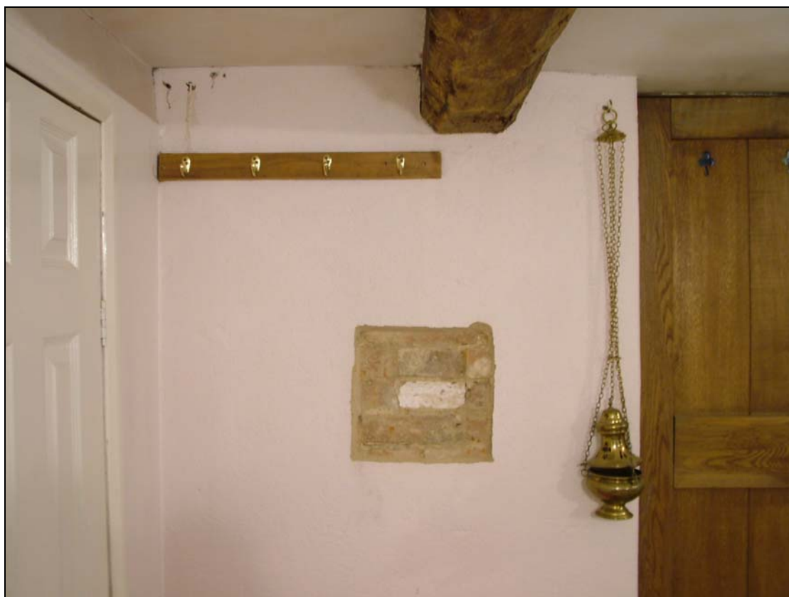
Plate 4. Opening in east Vestry wall to assess underlying fabric (5 on Figure 2)
