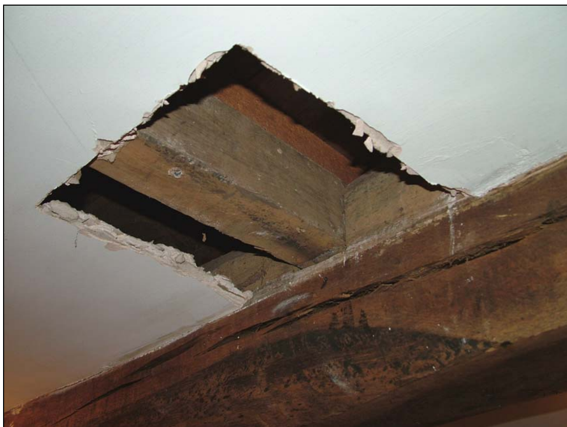
Plate 3. Opening to expose underside of Served floor structure (3 on Figure 2)
