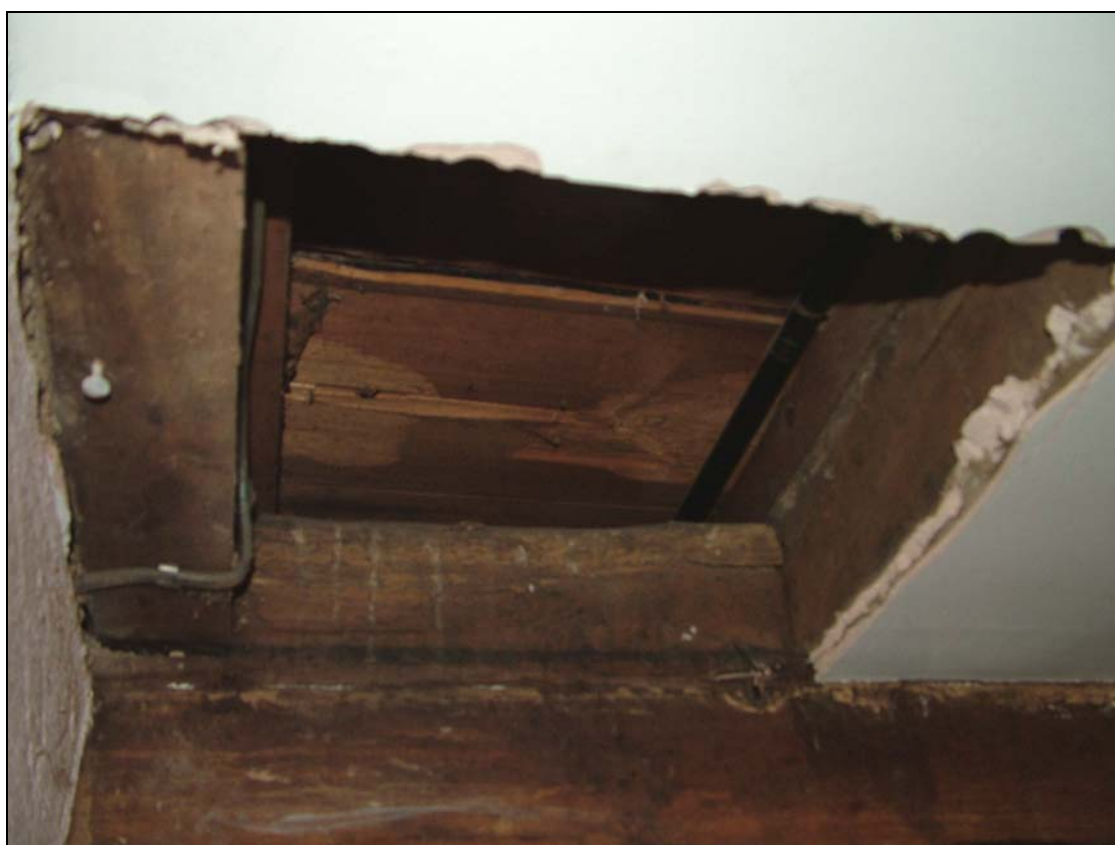
Plate 2. Opening to expose underside of Served floor structure (2 on Figure 2)
