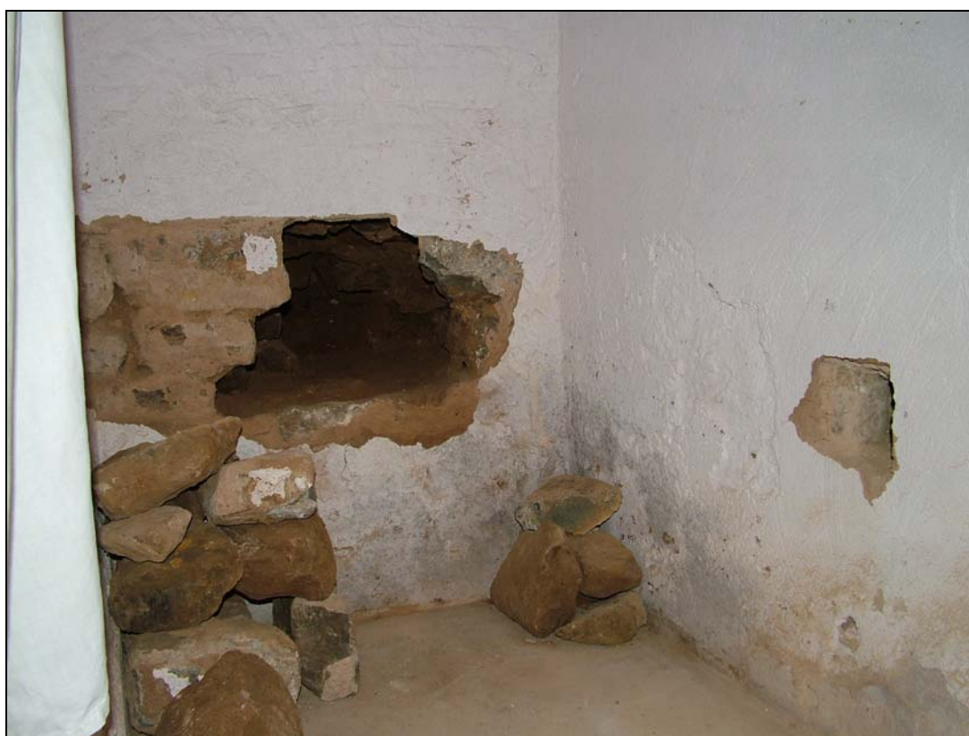
Plate 6. Small opening (on right) exposing moulding on north side, east face of Perpendicular arch within Vestry (illustrated on Figure 2)
