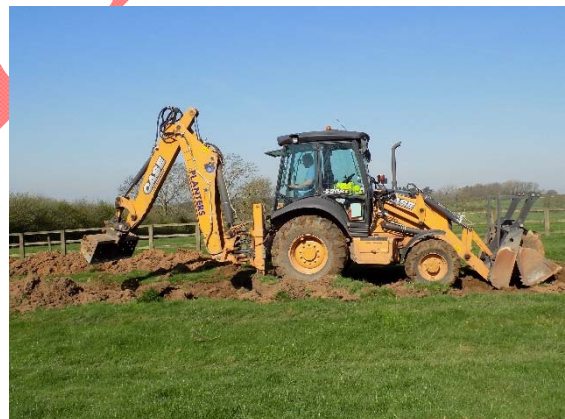
Mechanical excavator used on site
