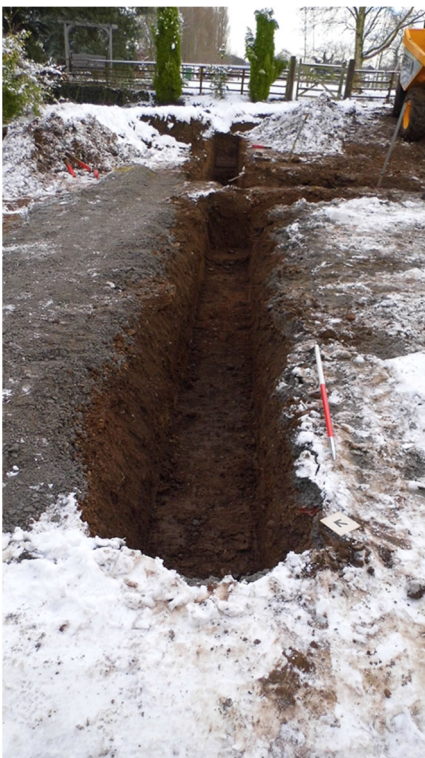
c. East facing view of retaining wall of garage (Scale: 1.00m)
