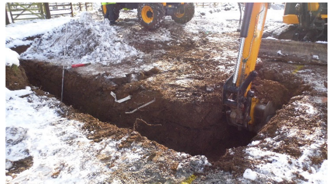
b. Southeast view of excavation of garage footings
