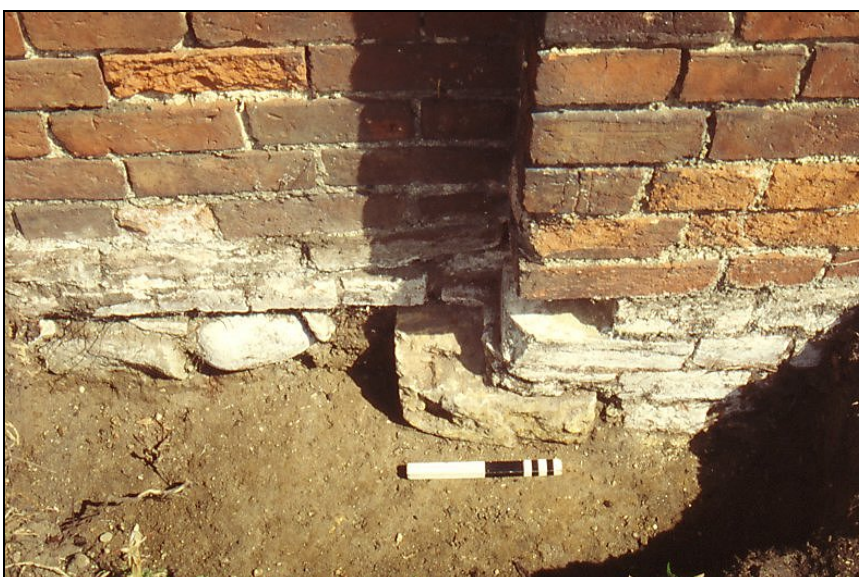
Plate 3. Truss T2 post-pad as revealed by excavation. Scale: 20cm
