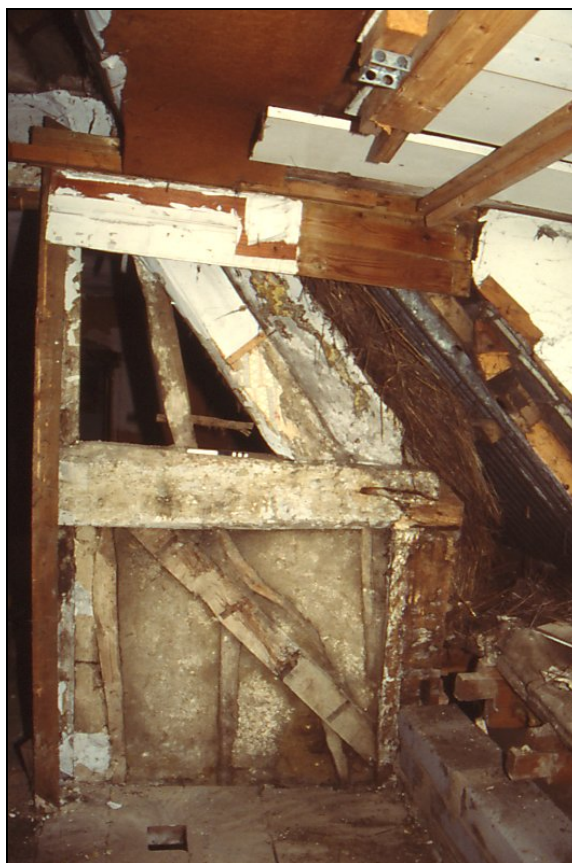
Plate 7. Detail of Truss T2 intact mud on lath infill below tie-beam, note reused timber for brace.
