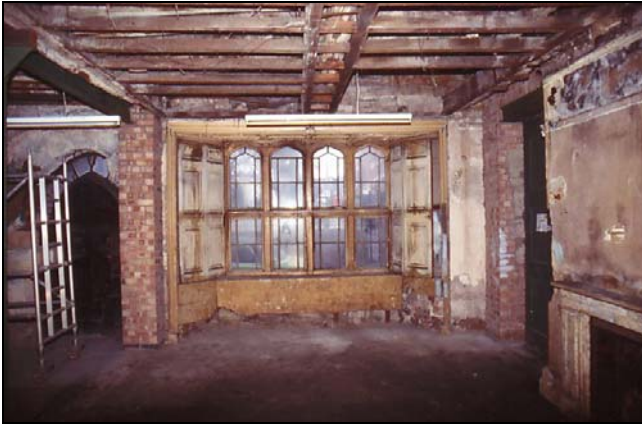
Plate 9. Interior of S end of former vicarage, looking E.
