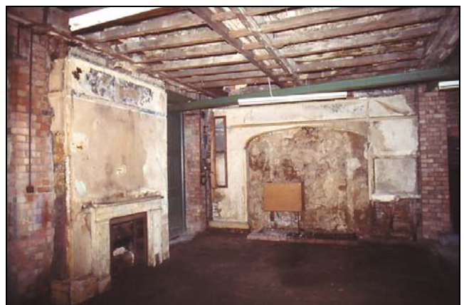
Plate 8. Interior of S end of former vicarage, looking W.
