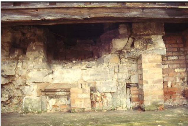
Plate 7. Window head & stair turret remnant N end of W elevation.
