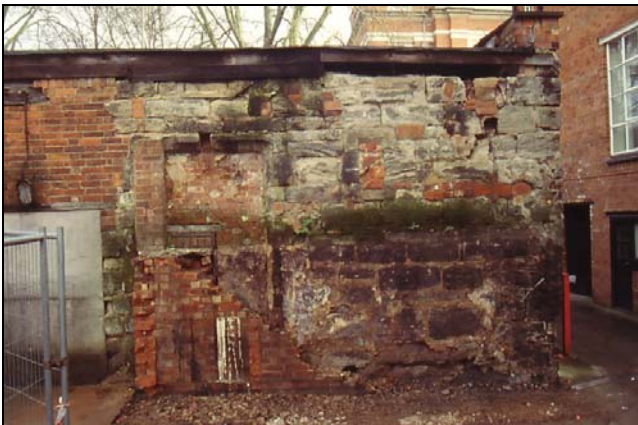
Plate 5. S end of W elevation after demolition of chemical store.
