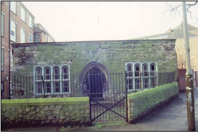
Plate 1. Former St. Mary's Vicarage: East elevation.
