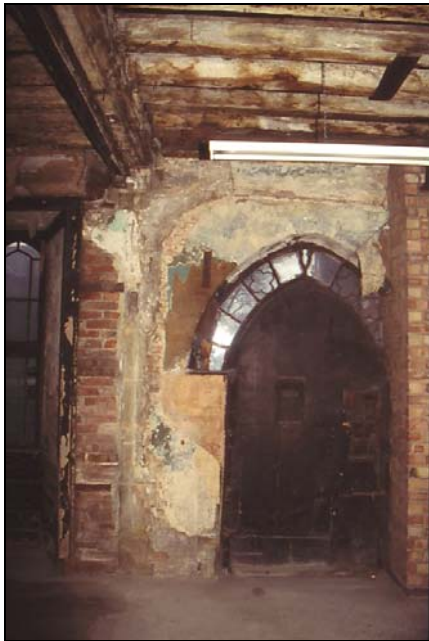
Plate 13. Blocked medieval openings on inner face of E wall.
