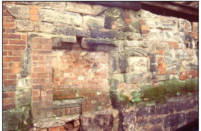
Plate 6. Detail of brick-blocked windows at S end of W elevation.
