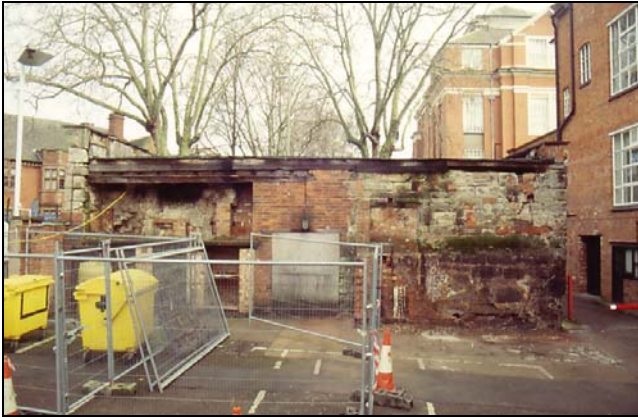
Plate 3. Former St. Mary's Vicarage: West elevation.
