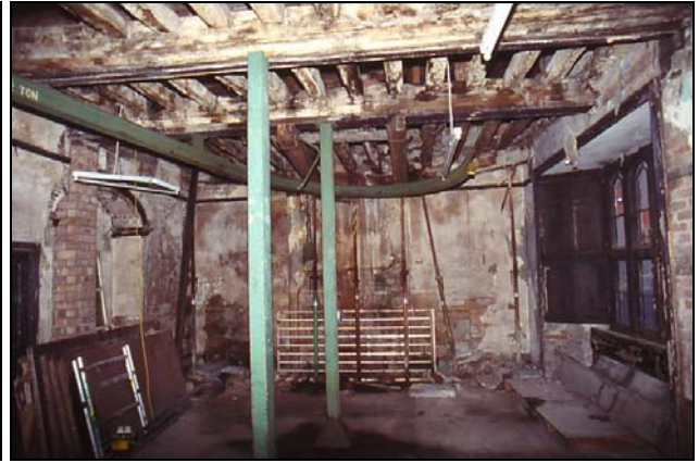
Plate 10. Interior of N end of former vicarage, looking N.
