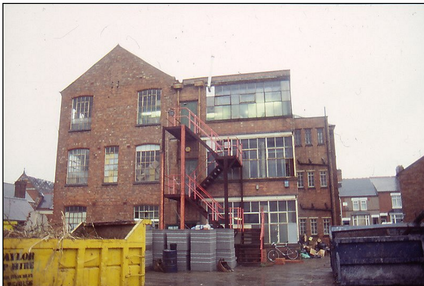
Plate 4. 30-44 Shilton Road. Rear (south) elevation, from left to right gabled Block B, Block C and Block G (C7)
