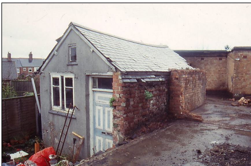
Plate 5. Former bakehouse to the rear of 12 Queen Street, Barwell, shortly before demolition (C11)
