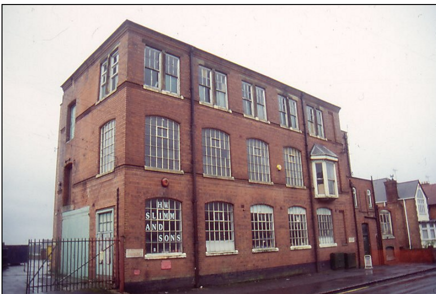
Plate 2. 30-44 Shilton Road. Frontage range, from the north-east (C5)
