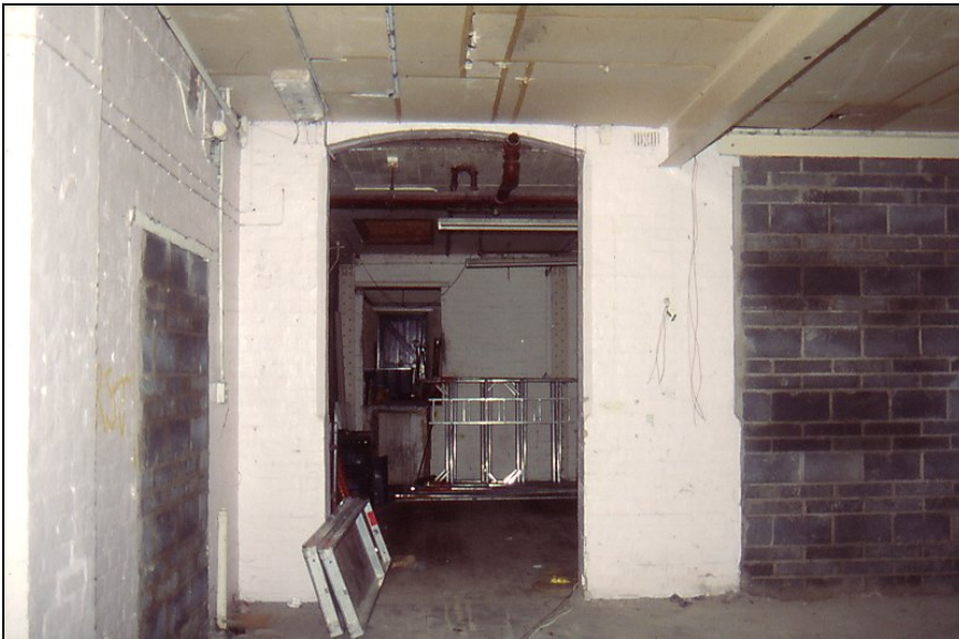
Plate 14. Ground floor interior Block B, former window in E wall converted to door into Block C beyond (C18)
