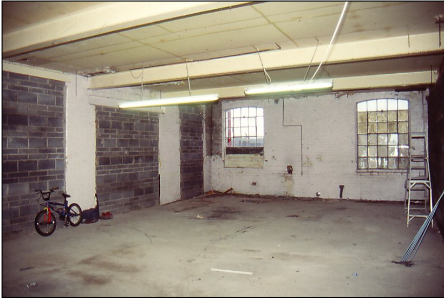
Plate 13. Ground floor interior of Block B, looking S (C14)
