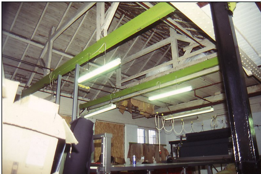
Plate 17. Second floor interior of Block B showing queen-post roof structure (C42)
