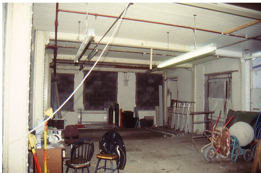
Plate 18. Ground floor interior of Block C, looking N to infilled windows in rear elevation of Block A (C20)
