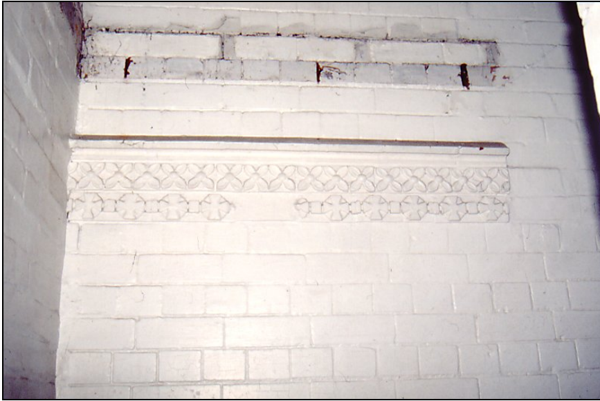
Plate 7. Terracotta decoration to external W elevation of Block A, now within Block D staircase (C26)
