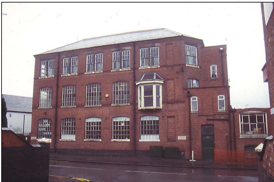
Plate 1. 30-44 Shilton Road. Frontage range, principal (north) elevation (C1)
