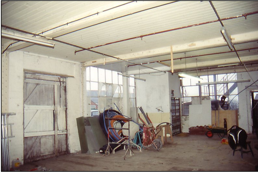
Plate 19. Ground floor interior of Block C, looking towards lift shaft in SE corner (C22)
