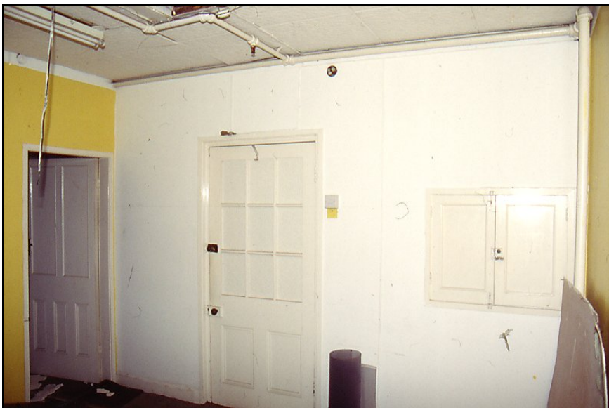
Plate 21. Single storey Block E, interior of former reception/office, looking E (C24)
