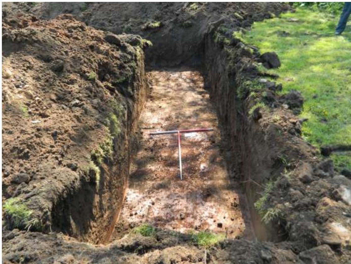
Figure 10: Trench 1, looking west (post excavation of east-west area)
