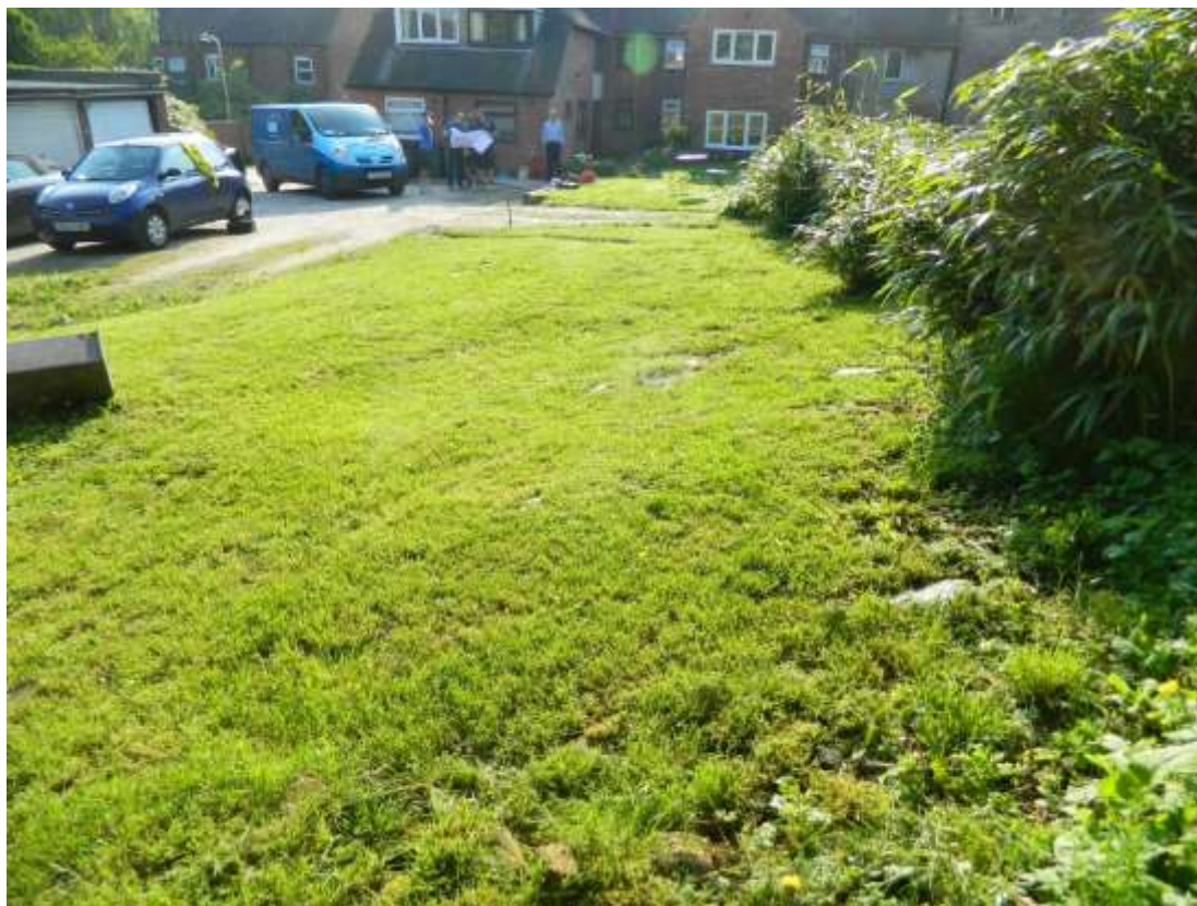
Figure 4: General view of site, looking south. Area to contain a single bungalow with an associated driveway and parking.
