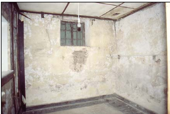
Photo 7. Interior of suspected schoolroom (B).
