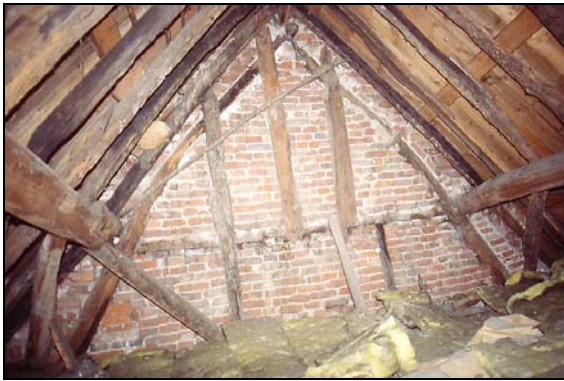
Photo 5. Roof structure of A, looking towards east gable.
