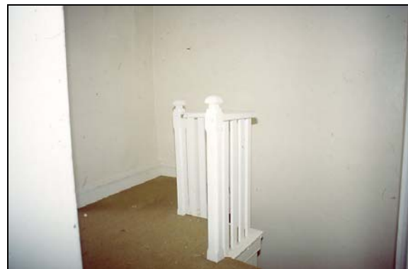
Photo 8. Landing area showing faceted newels to staircase.
