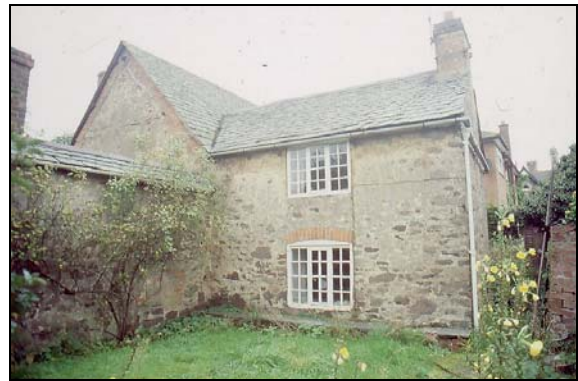
Photo 4. Two-storey rear (north) range C
