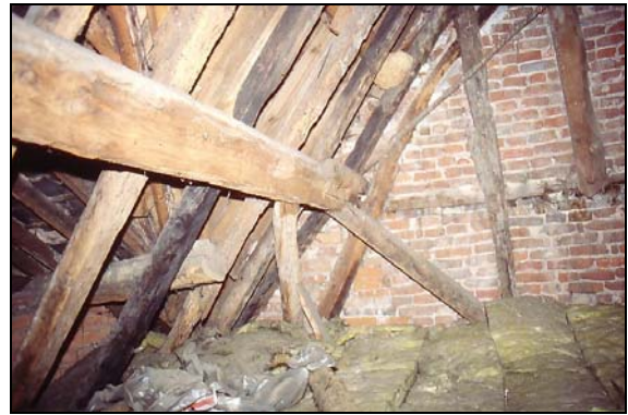
Photo 6. Detail: roof structure of A showing scarfed purlin.
