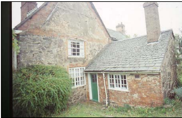
Photo 3. Range A to left and single-storey kitchen D.
