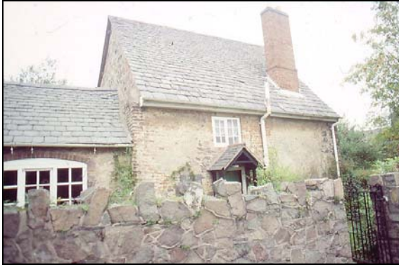
Photo 1. Front elevation of 57 Leicester Road (A to right).
