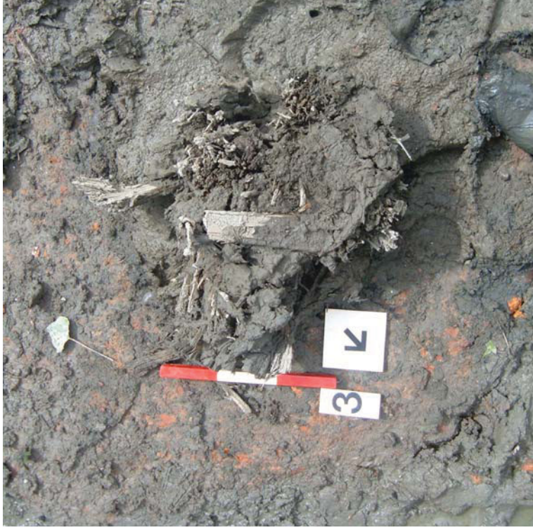
Figure 6: Condition of post 3. The timber has been badly damaged after being shortened. Part of the brick rubble and concrete plinth is visible.
