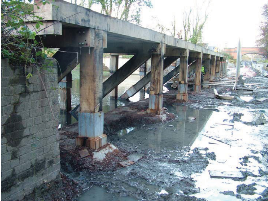
Figure 12: Completed structural restoration from south-east.
