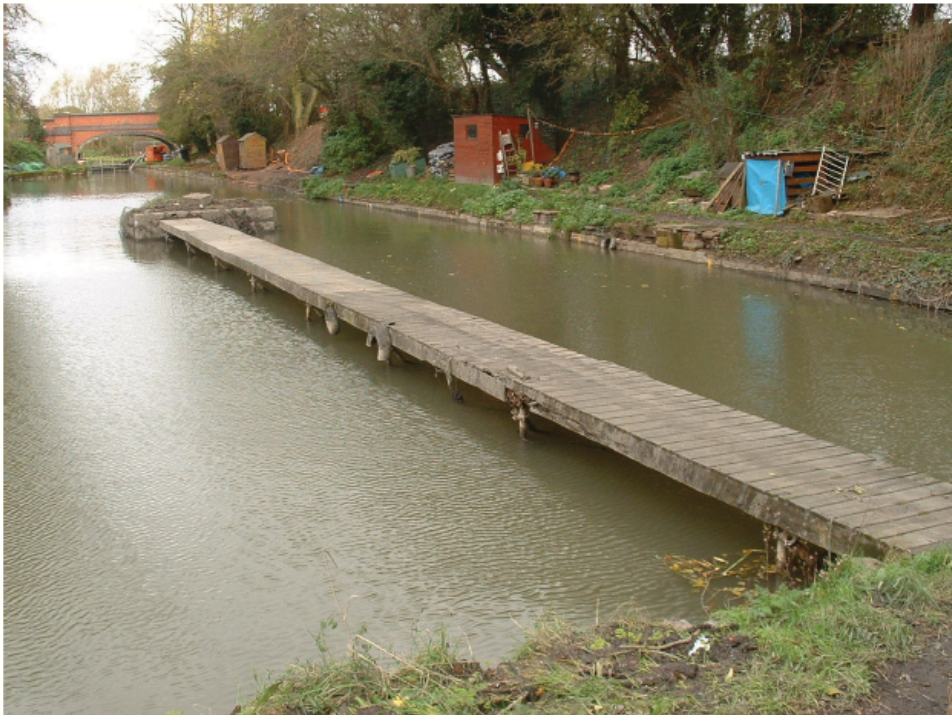
Photo 30 General view of timber walkway and island, looking north
