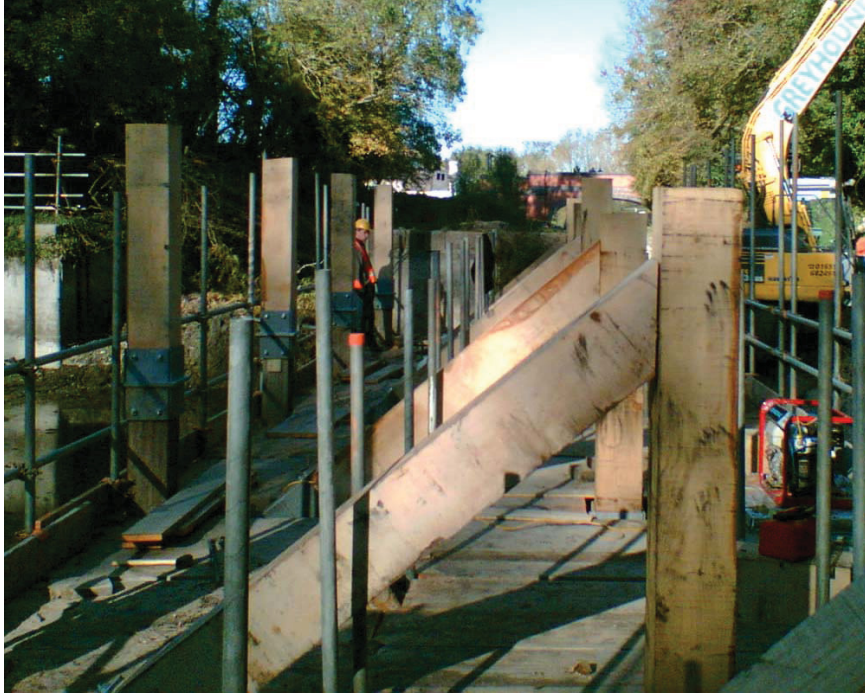
Figure 10: Reconstructed diagonal braces
