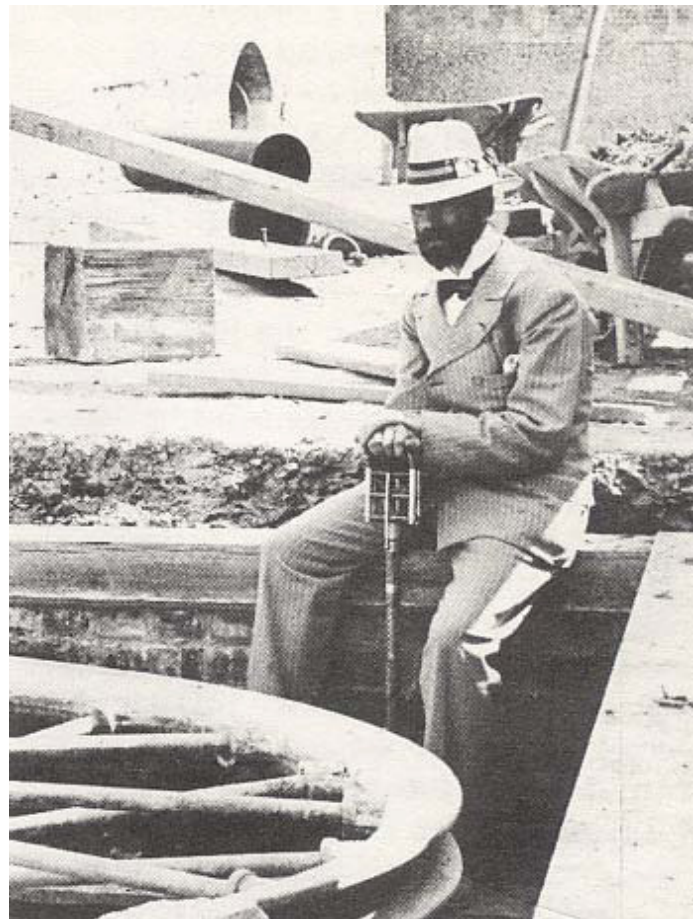
Figure 14: Gordon Cale Thomas sat within the wheel-pit.
