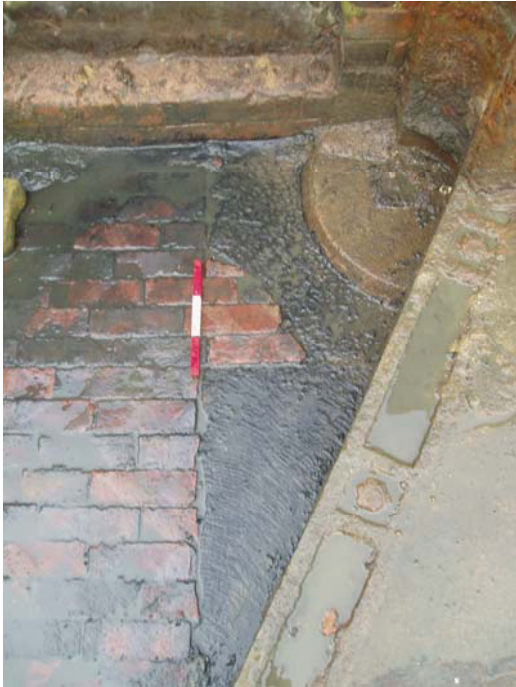
Figure 11: Detail of brick repair to sandstone flag
