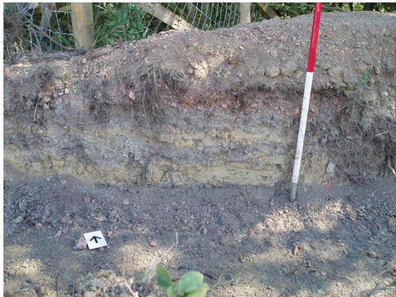
Figure 3: Section through eastern towpath showing reddened shale.
