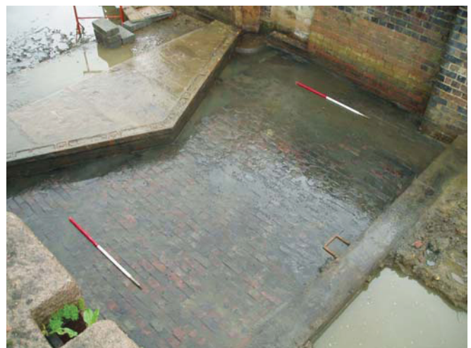
Figure 14: General view of Stop Lock floor
