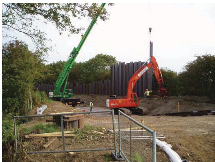
Figure 16: Piling of eastern bank
