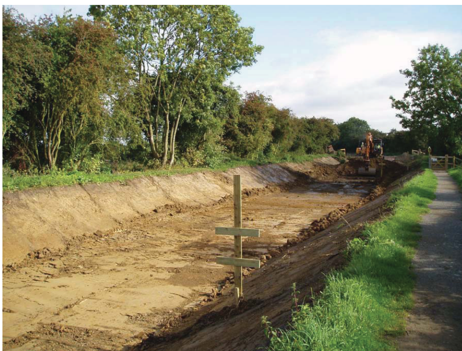
Figure 2: Re-excavated Upper Arm
