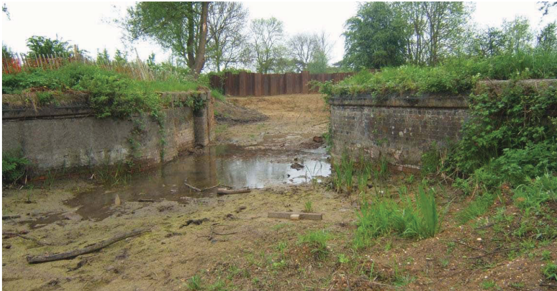
Figure 6: Stop Lock from the North 15/05/2006
