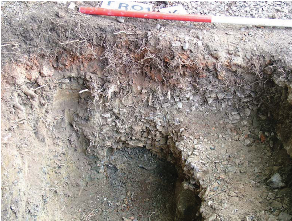
Colour Photo 1 North West Facing Section of Trench 1. The burnt shale or clay is probably original towpath material. The rubble wall is to the right, and the dry-mix can be seen in the exposed section.
