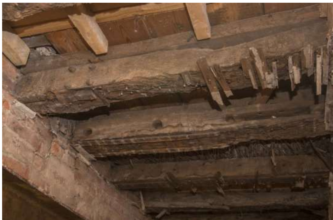
Figure 21 Re-used timber joists above former corridor Looking east
