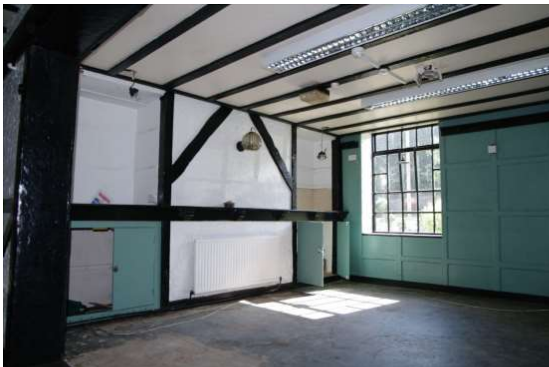
Figure 14 Lounge 1 Looking south. Before soft-strip. Stub of corridor wall on left
