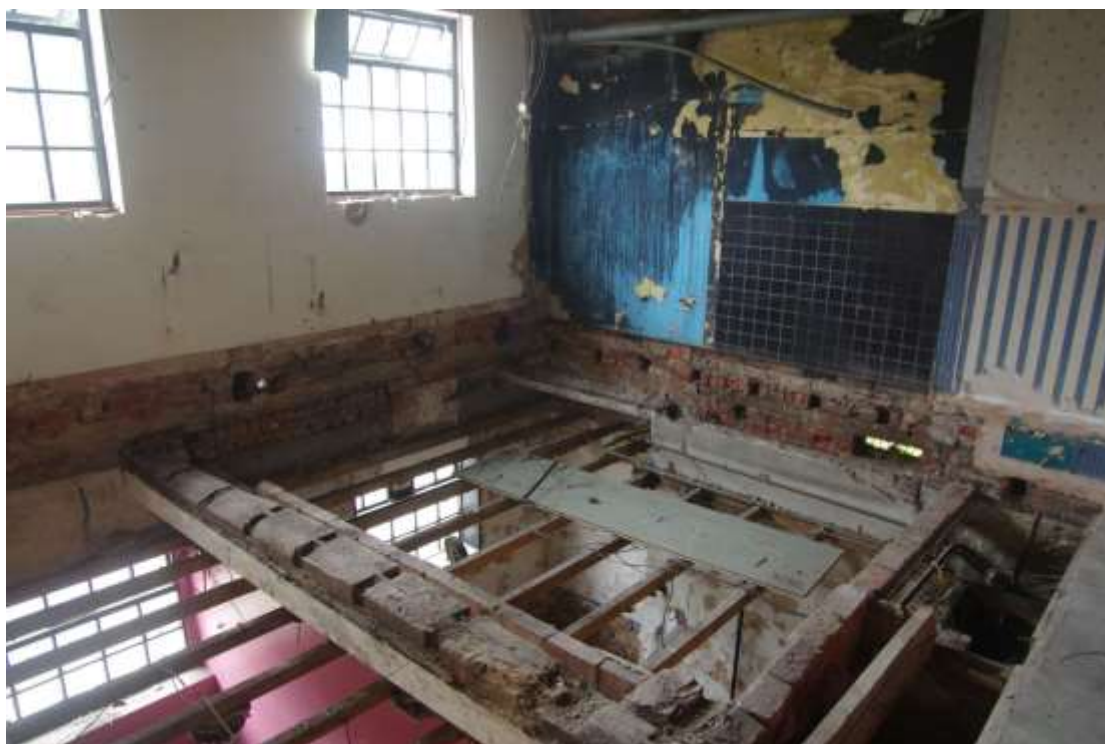
Figure 25 Exposed floor structure in former Bedroom 10 Looking south-west
