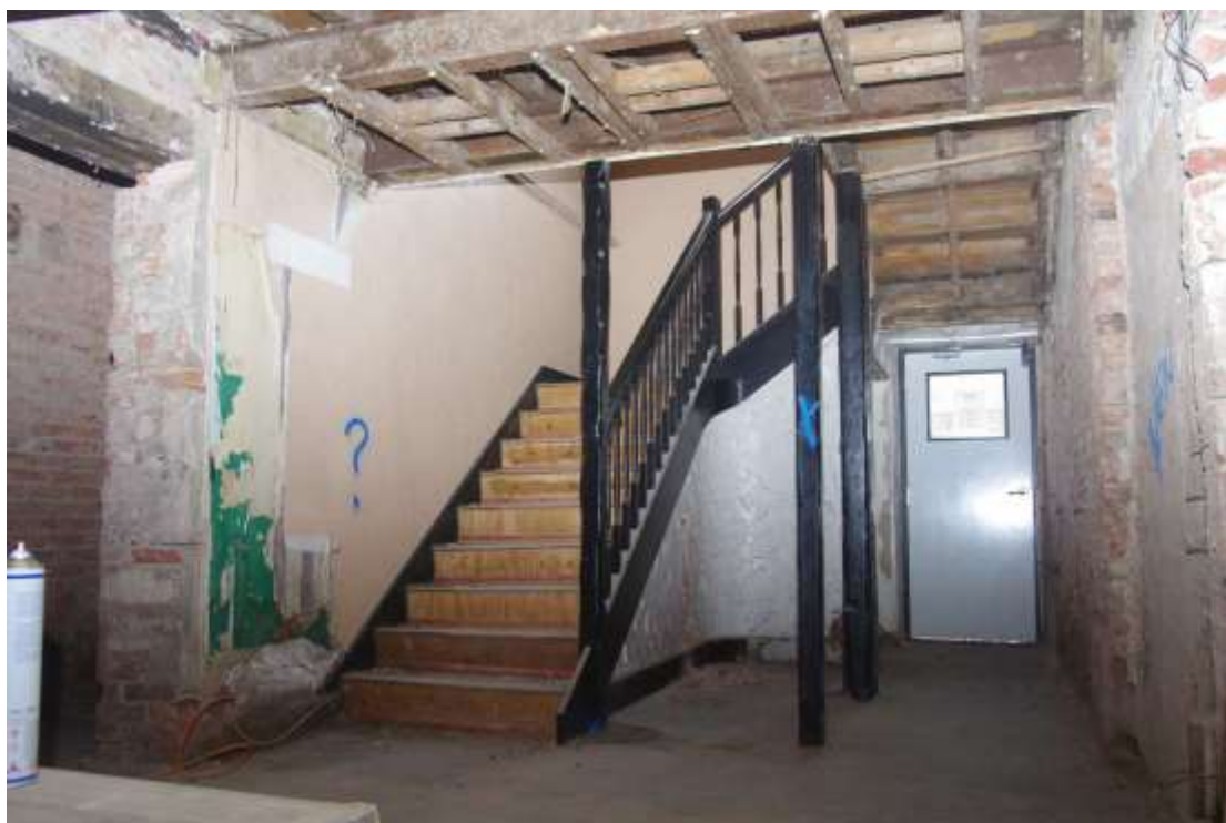
Figure 22 Hallway Looking south. Doorway to Bondgate on right of stairs
