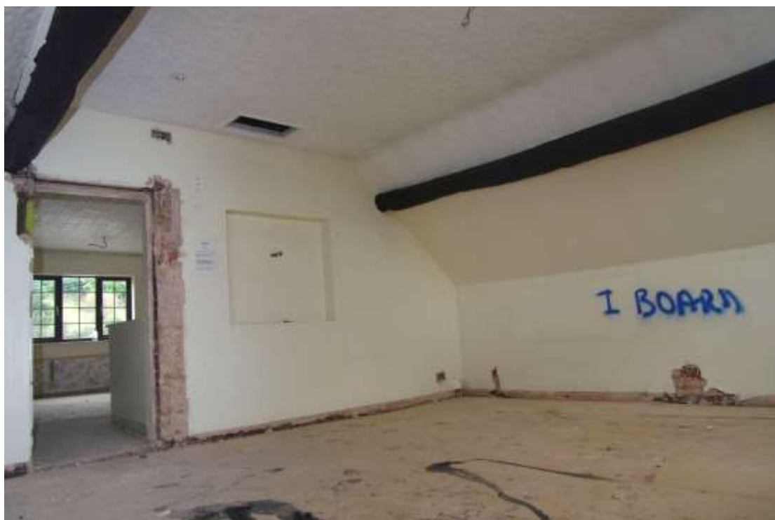
Figure 30 Bedroom 18 Looking south-west. Note recess on wall for possible internal window
