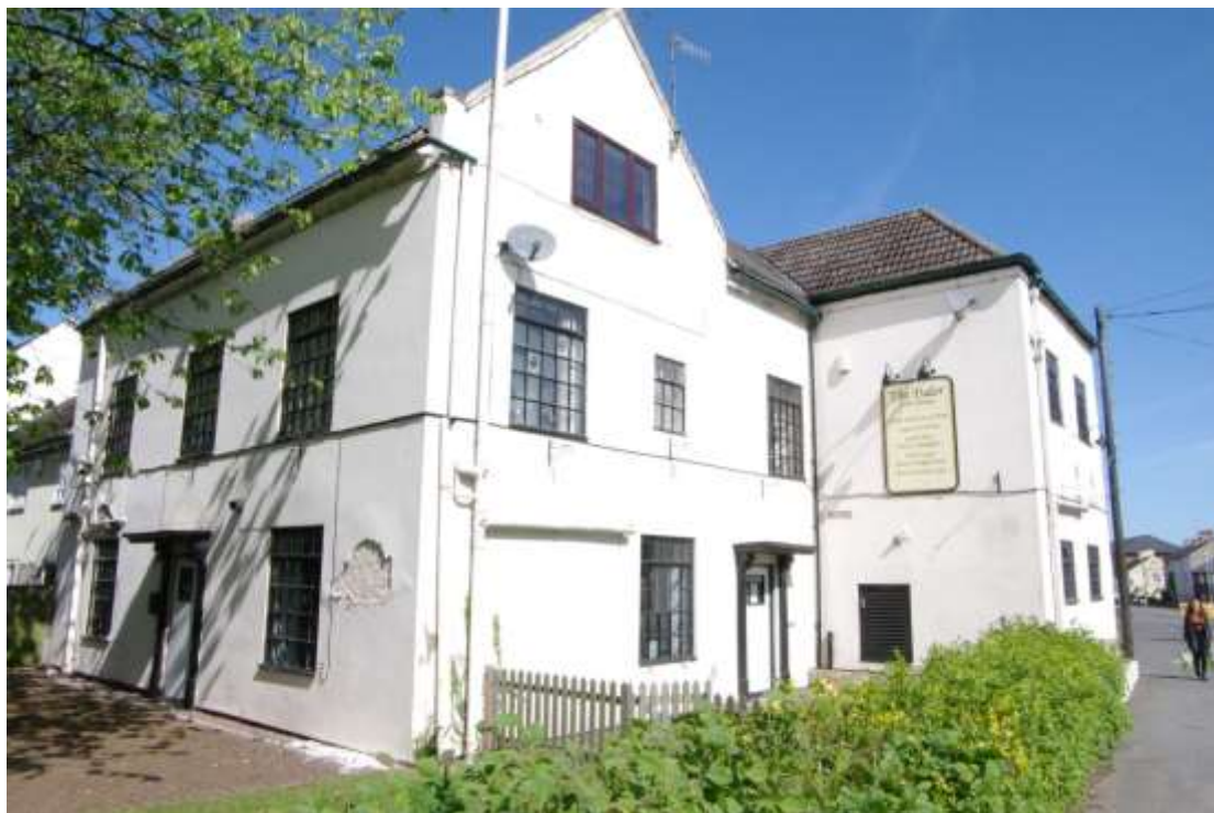
Figure 11 South-east corner of the Tudor Inn Looking north-east
