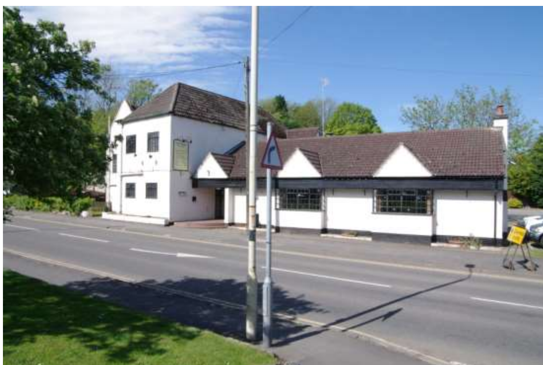
Figure 10 South-west facing elevation Looking north.
