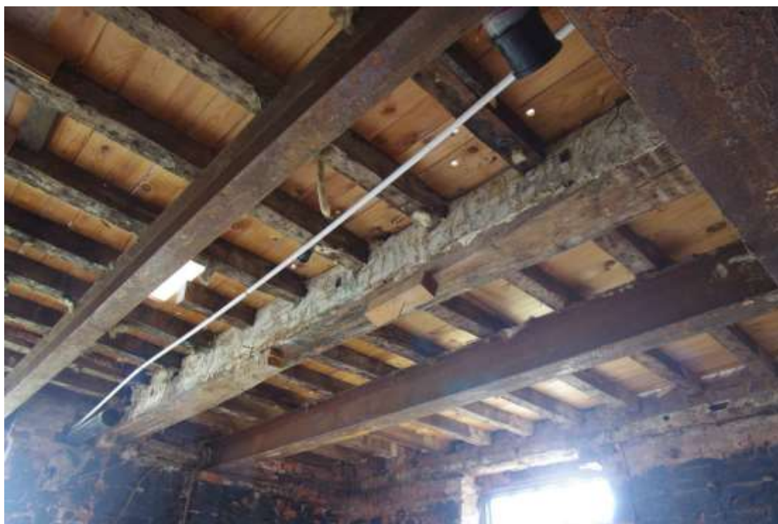
Figure 19 Lounge 1 ceiling detail Looking towards south-west corner of the room
