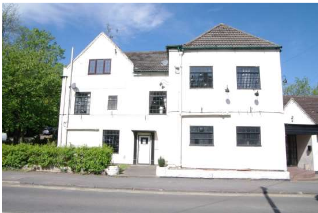
Figure 9 South-west facing elevation Looking north-east. Modern function room on right
