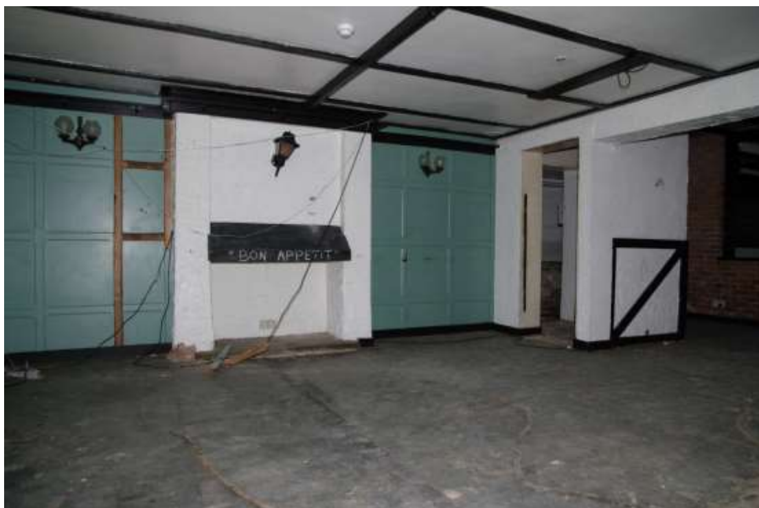
Figure 18 Lounge 2 fireplace Looking north-east. Entrance to Lounge 3 on right
