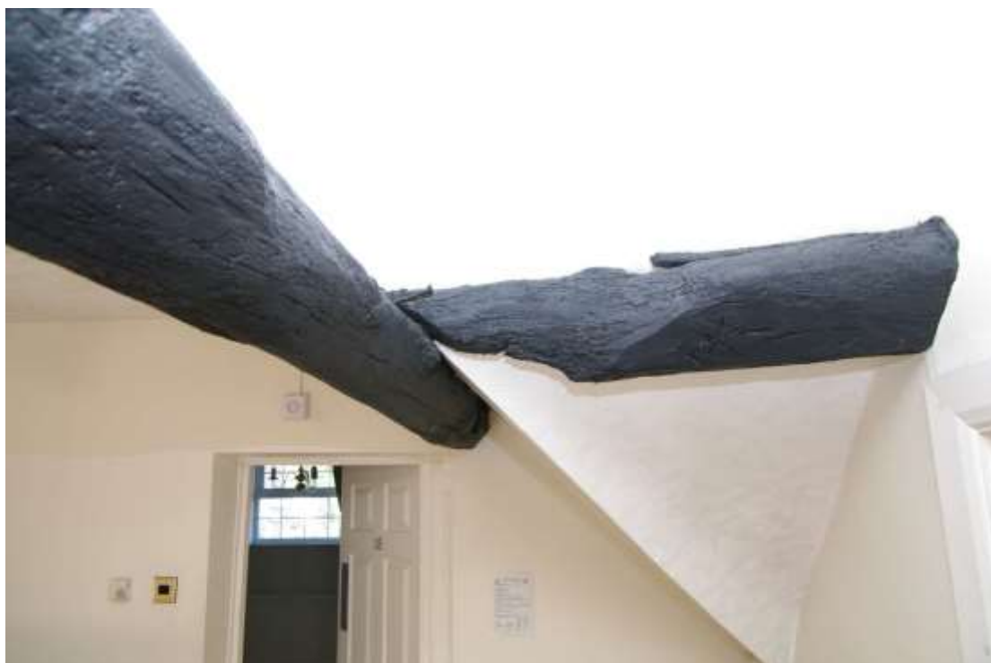
Figure 29 Joint of purlins on former second floor lounge Looking north-east
