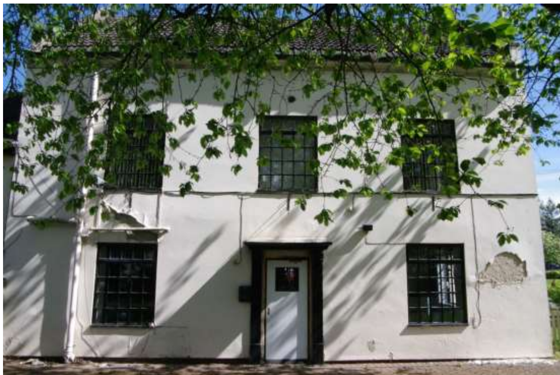
Figure 7 North-west facing elevation Looking south-east
