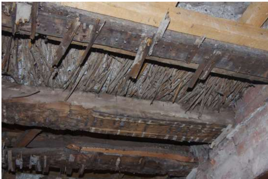
Figure 20 Ceiling above former corridor Plaster floor above corridor
