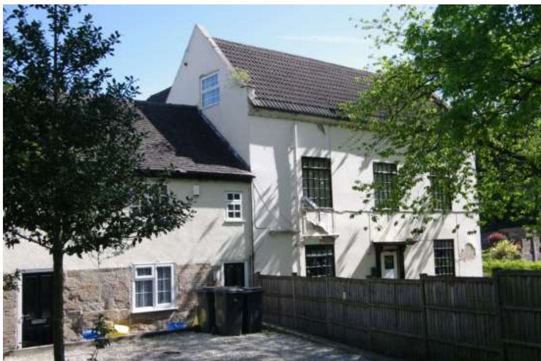
Figure 8 North-west facing elevation and adjacent cottages Looking south
