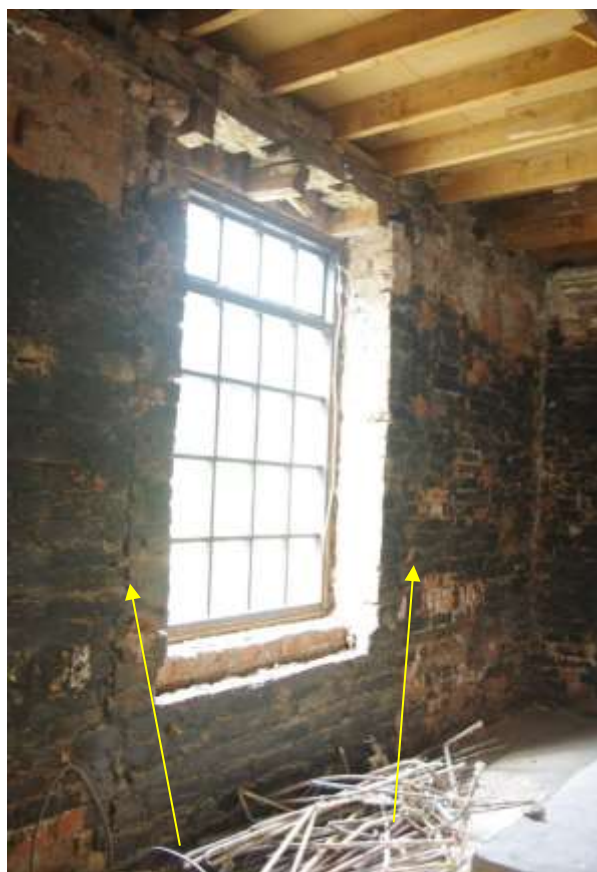
Figure 16 Lounge 2 north-west facing window Looking north. Note infilled brickwork around window
