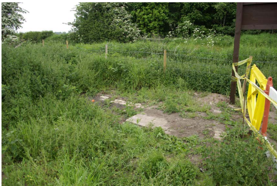
Figure 4 Brickwork exposed by machine prior to the evaluation Looking north. Former railway line ran across the road in the gap between the hedge lines on left of picture
