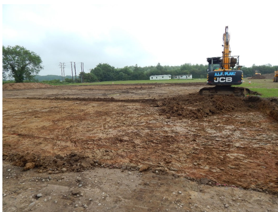
Figure 6: Sub-soil stripping for structure foundation. Looking east.
