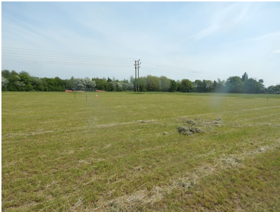
Figure 4: Area prior to ground-works looking east, to new Farm house construction from proposed farm yard
