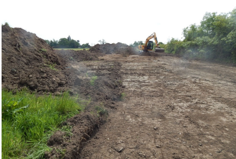
Figure 5: Topsoil stripping for Farmyard formation. Looking south.
