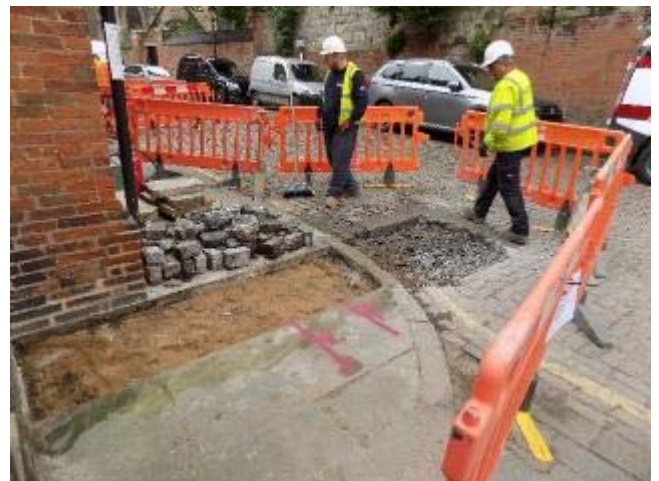
b. Slot in No. 9 after removal of stone slabs
