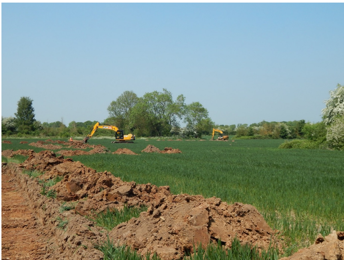
Figure 5: Work in progress in Field 881, looking north
