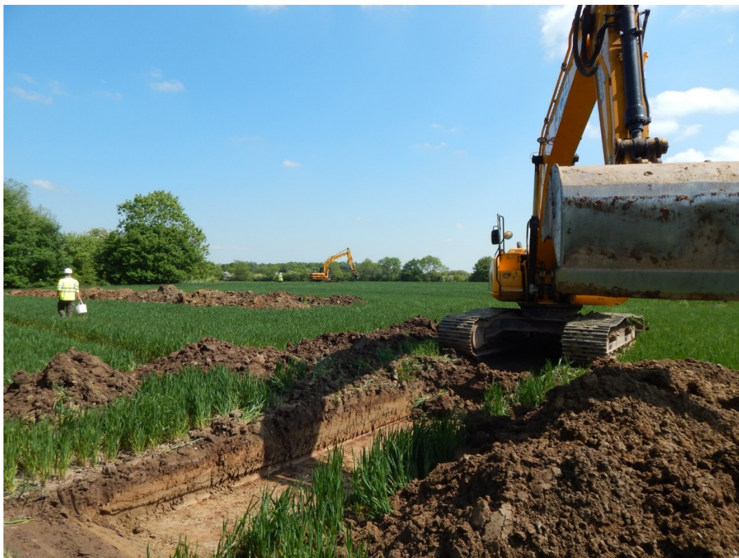
Figure 8: Work in progress in field 721, looking south-east
