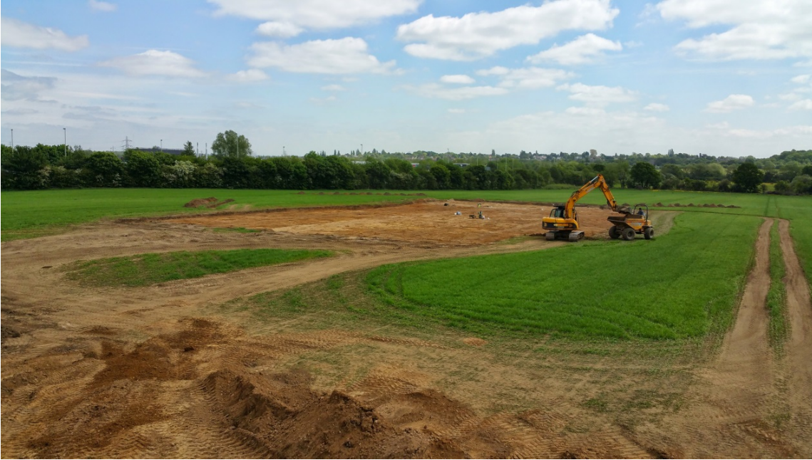
Figure 6: Machine strip in progress; view north-east
