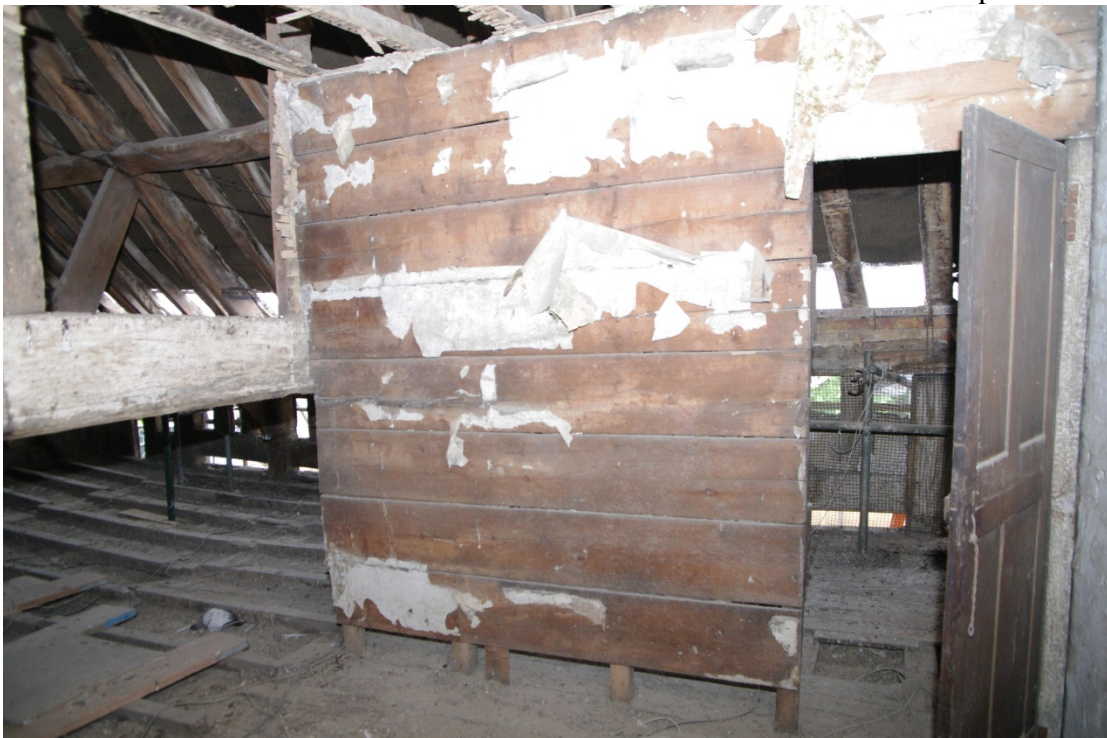
Figure 16 Servant's quarters in roof space Looking north-west
