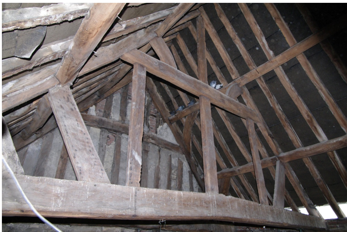
Figure 18 Trusses 1 and 2 from eastern side Looking north-west with Truss 2 in foreground
