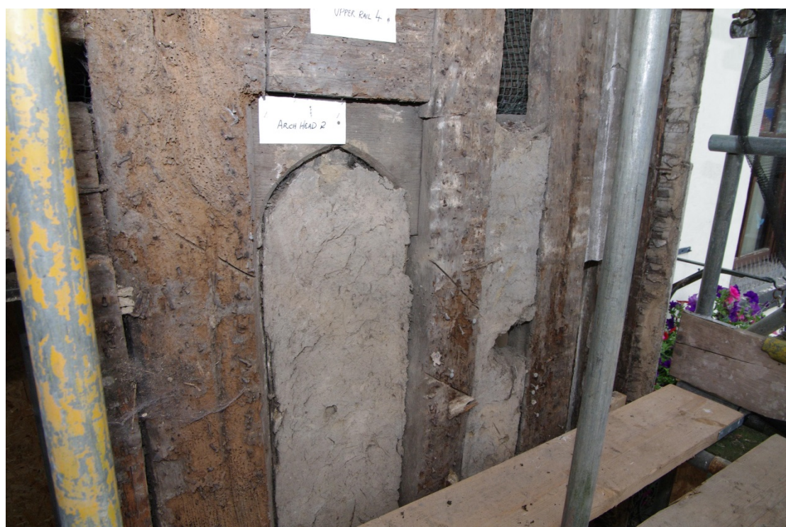
Figure 10 Decorative arch head between posts Westernmost arch. Note diagonal grooves in posts
