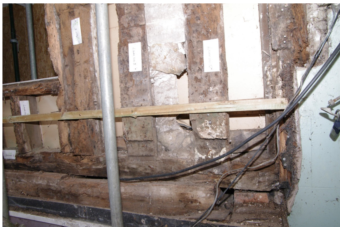
Figure 11 First floor, eastern side Remnants of plaster and stone infill between studs
