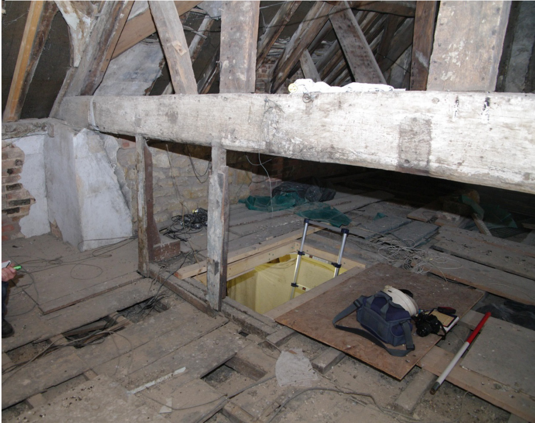
Figure 15 Roof space, east side of Truss 1
