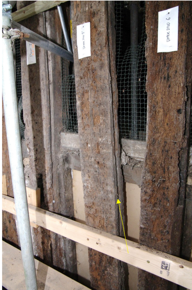
Figure 12 Close-up of groove for stones in timber post
