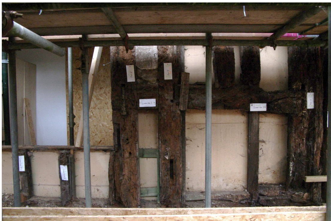
Figure 6 First floor window cutting across timbers Window on left of picture
