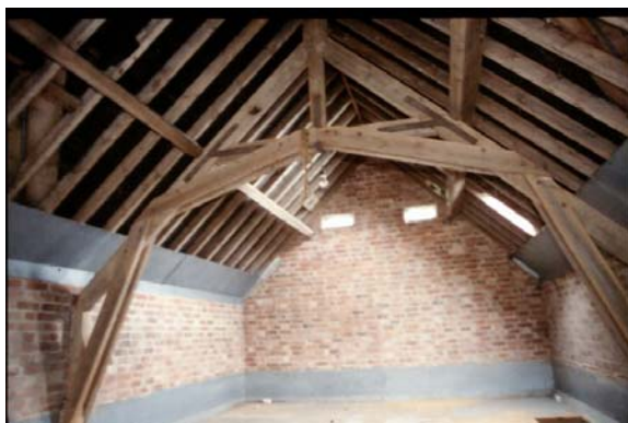
Photo 2 Roof Construction Within the Grain Loft
