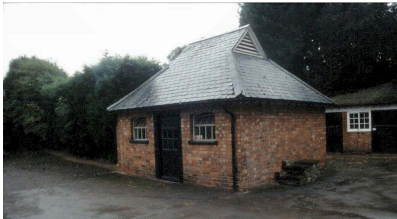
Photo 3 Building 5 Front & Right Elevation
