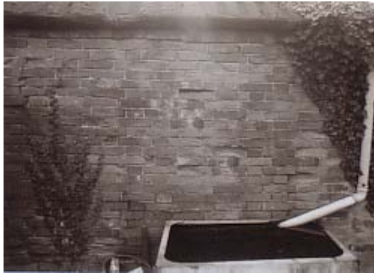
Photo 4 Earlier Brickwork, Building 2
