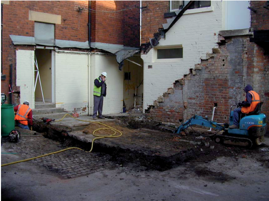
Colour Plate 1 Area of Watching Brief, Work in Progress.
