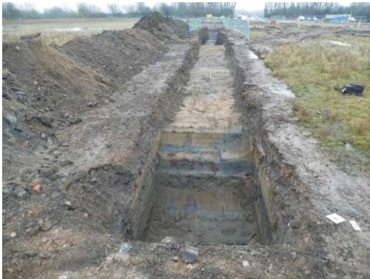
Figure 10: Trench 2, Looking South-east
