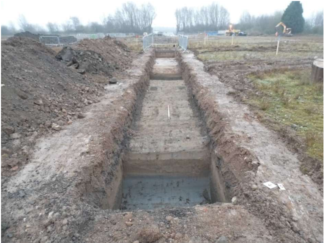
Figure 4: Trench 5, looking south-east
