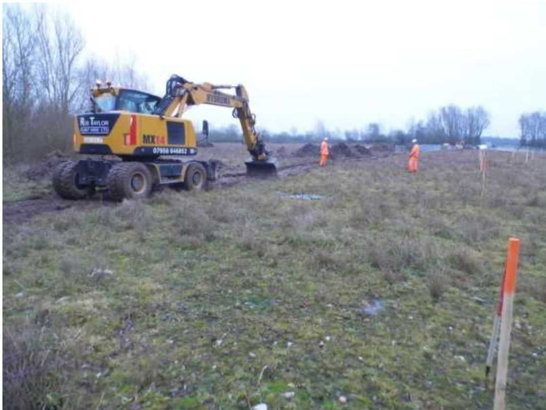
Figure 7: Removing hardcore in Trench 4
