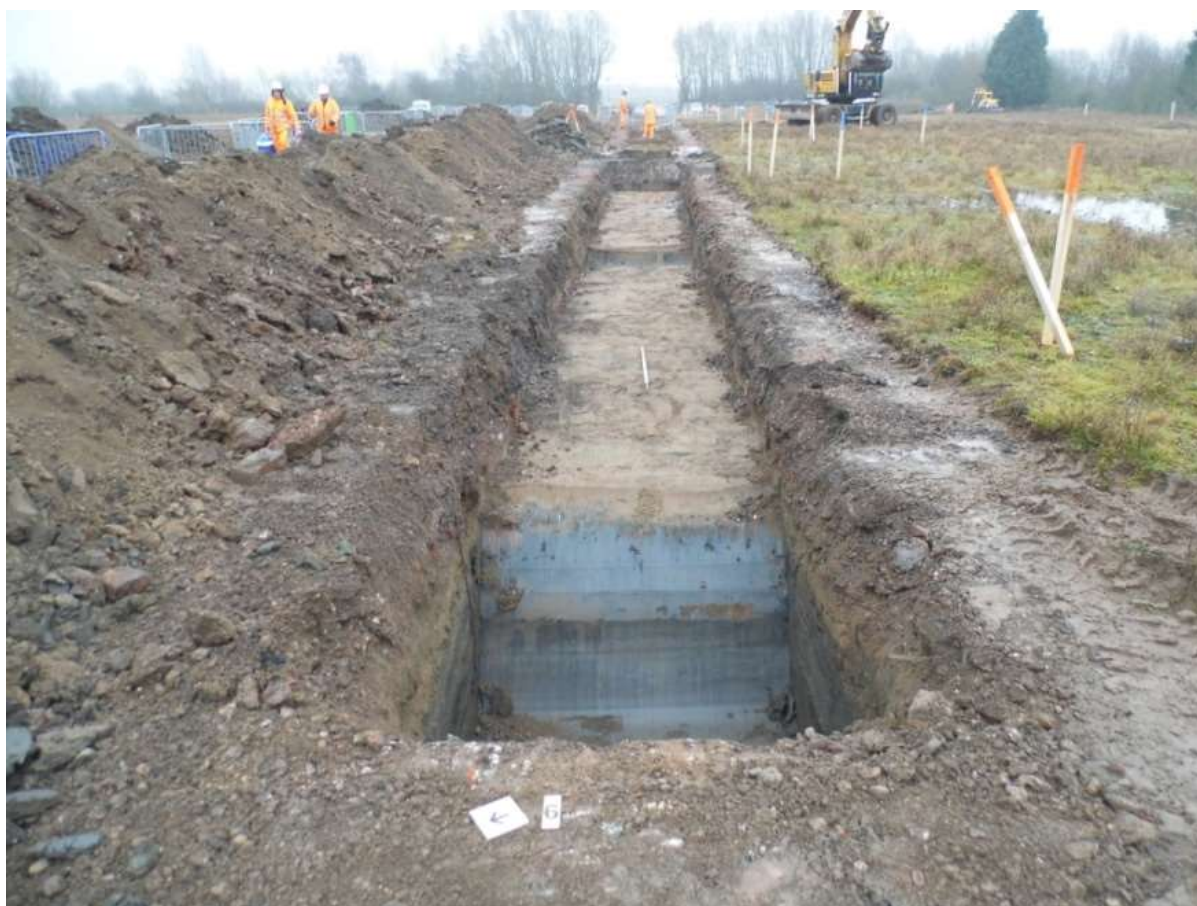
Figure 5: Trench 6, looking south-east
