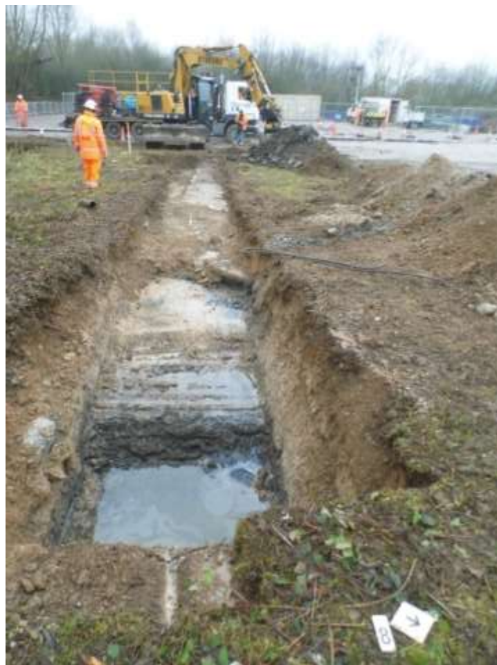
Figure 7: Trench 8, looking south-west
