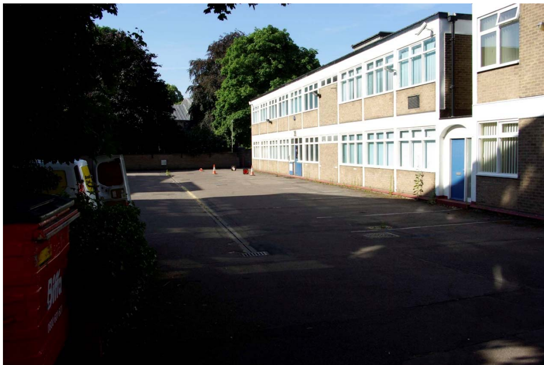
Figure 5 Car park Looking south
