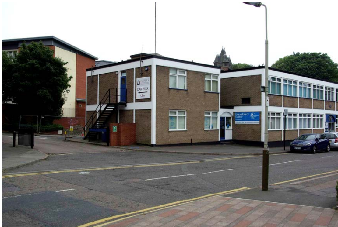
Figure 4 Site viewed from Castle Street Looking south-east. Entrance to site car park on left of picture
