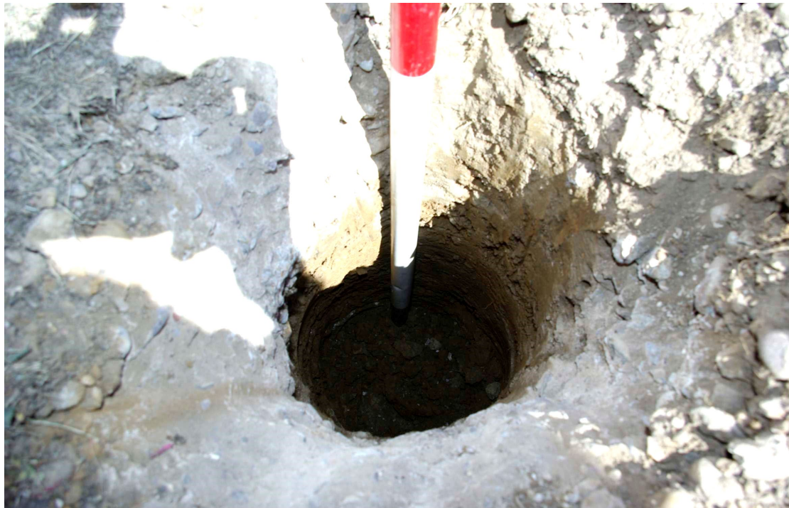
Figure 8 View into Gate Post hole 3 1m scale
