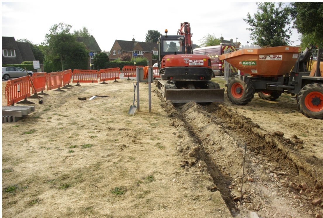
Figure 13 Pathway Stage 4 being completed Looking south-east towards car park
