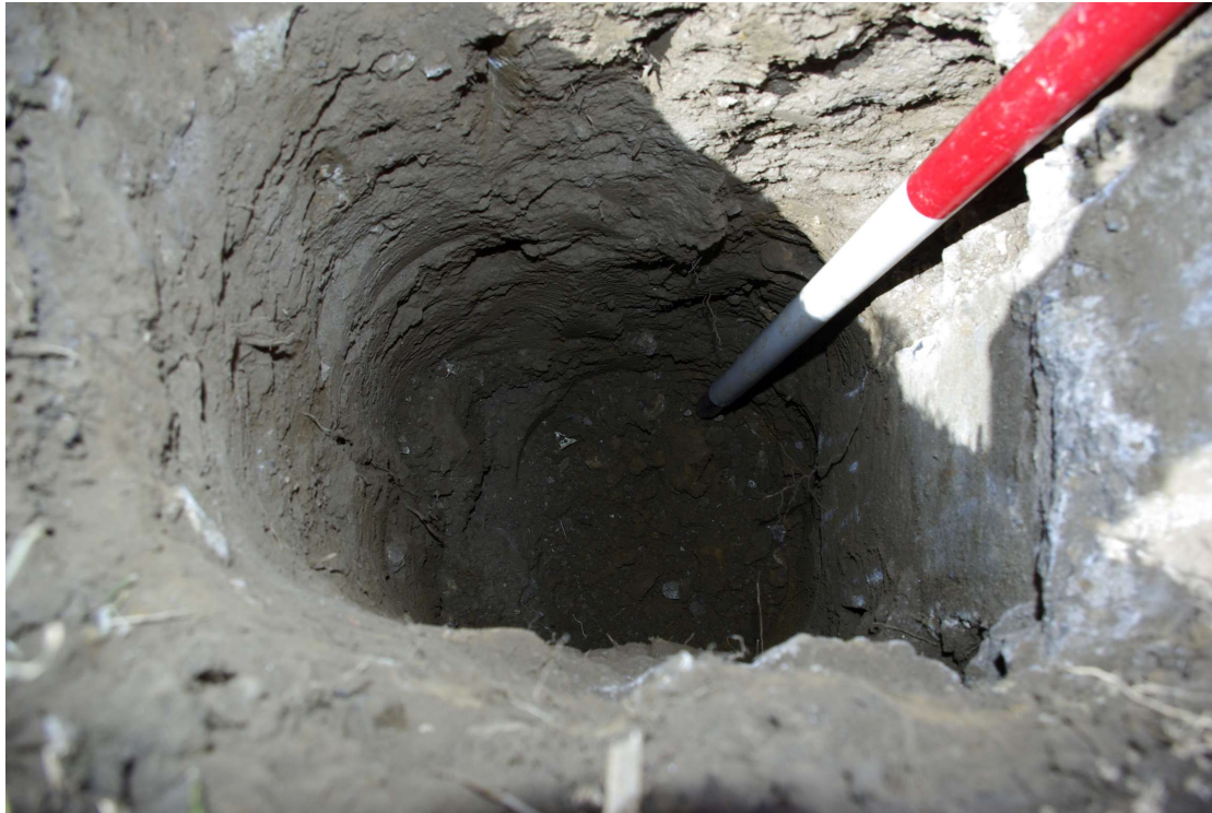
Figure 7 View into Gate Post hole 2 1m scale
