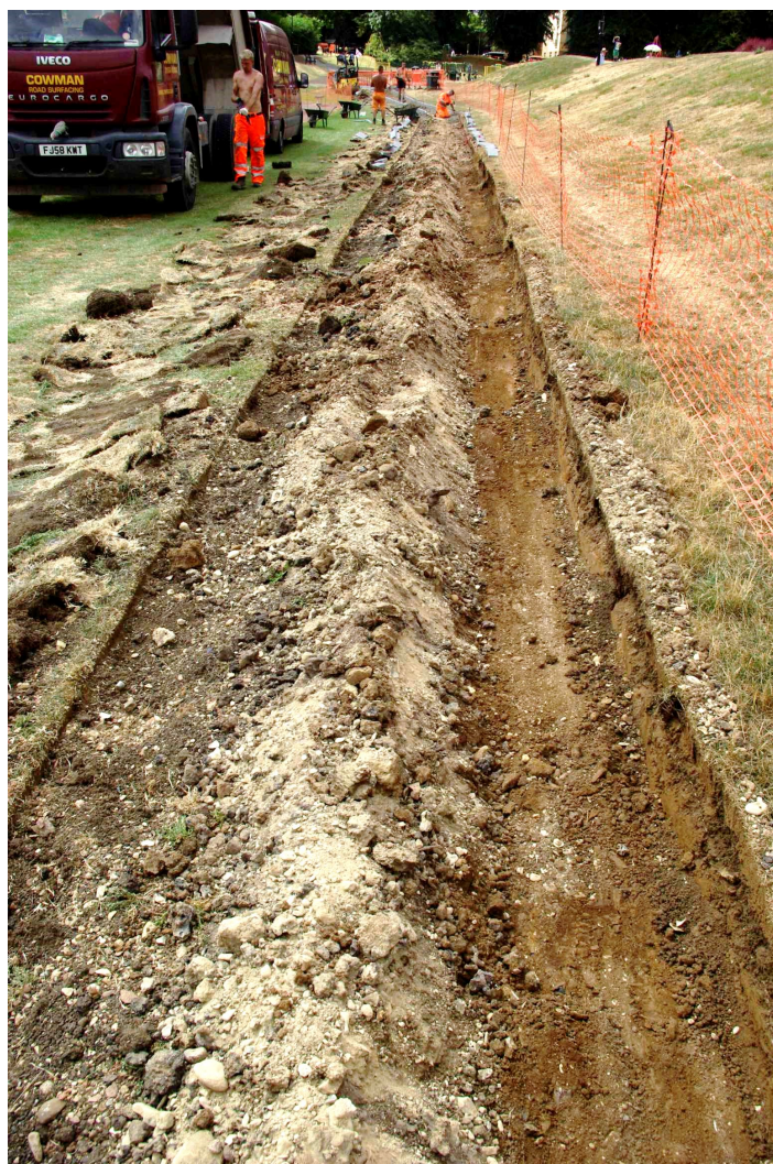
Figure 12 Pathway Stage 3, final excavated level Looking west
