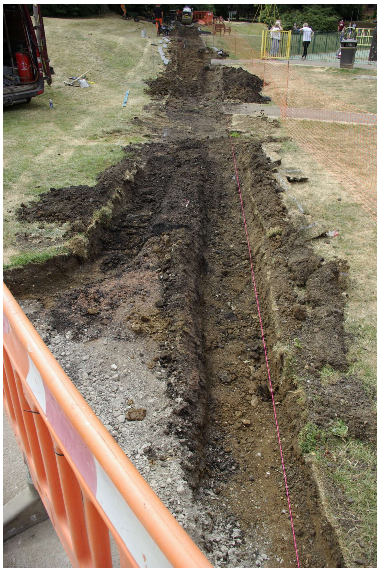
Figure 11 Pathway Stage 2, final excavated level Looking south-west
