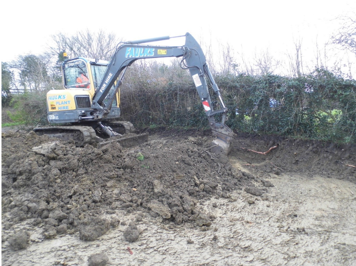
Figure 3: Removing topsoil/subsoil
