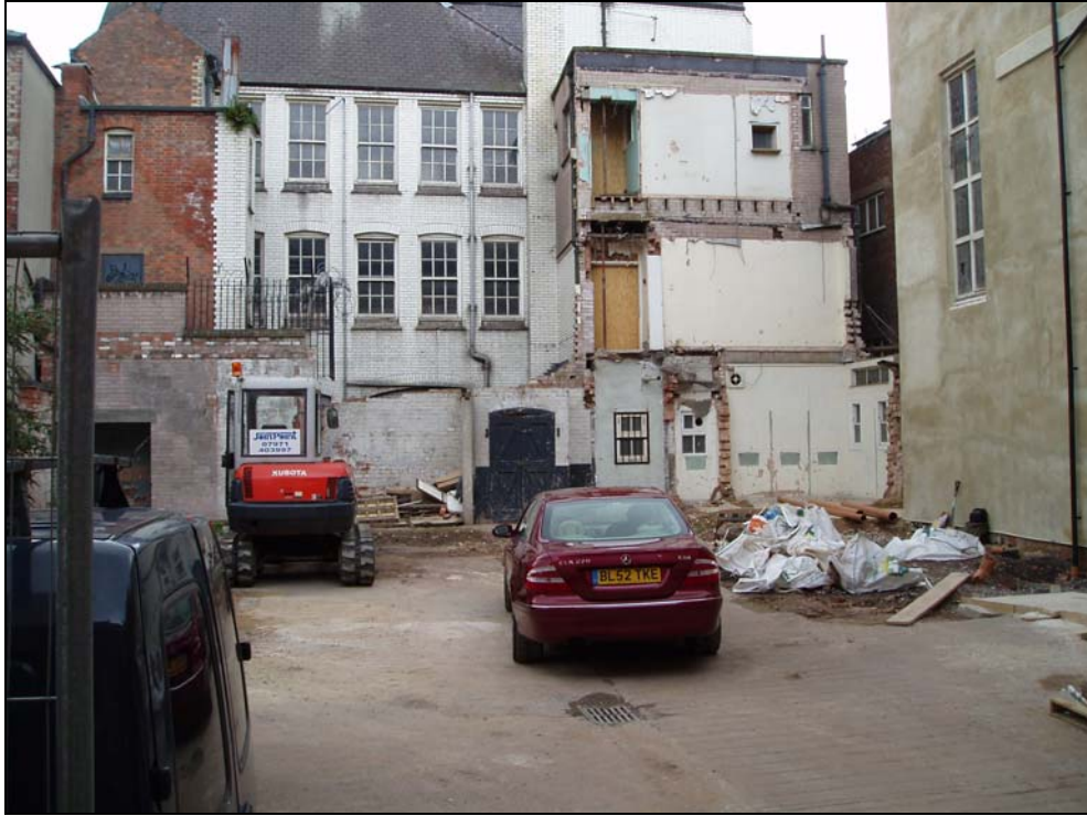
Plate 2. Trench location before excavation. Looking east.
