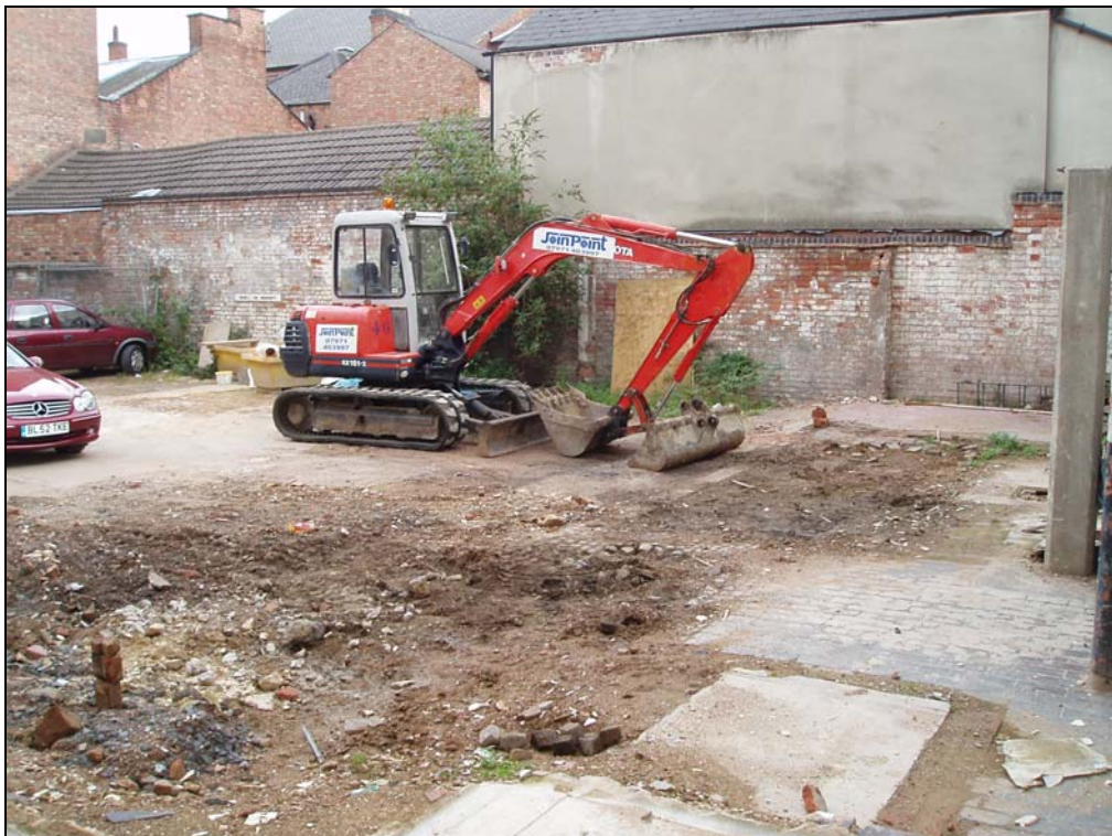
Plate 1. Trench location before excavation. Looking north.
